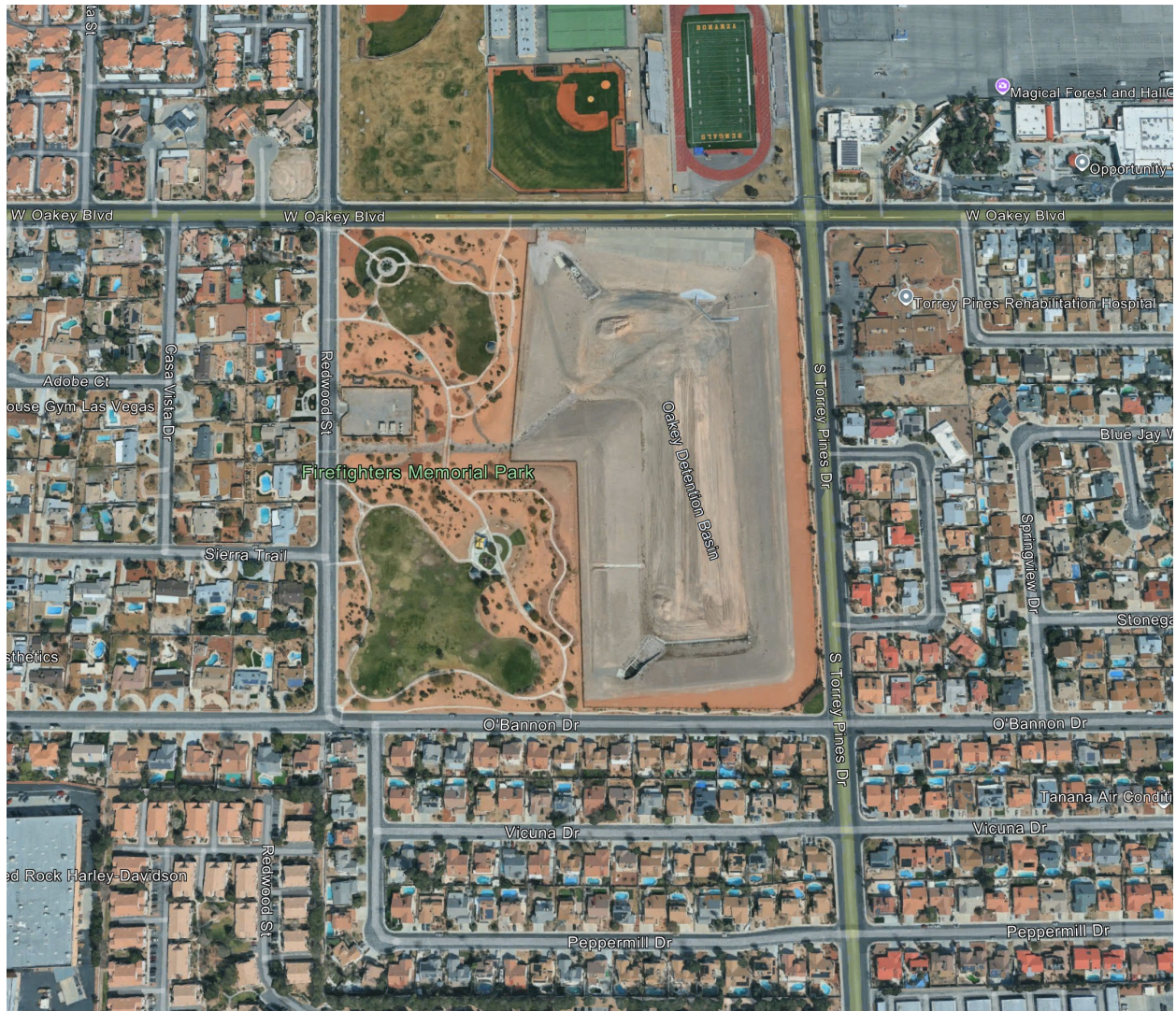
Figure 5. Oakey Detention Basin
