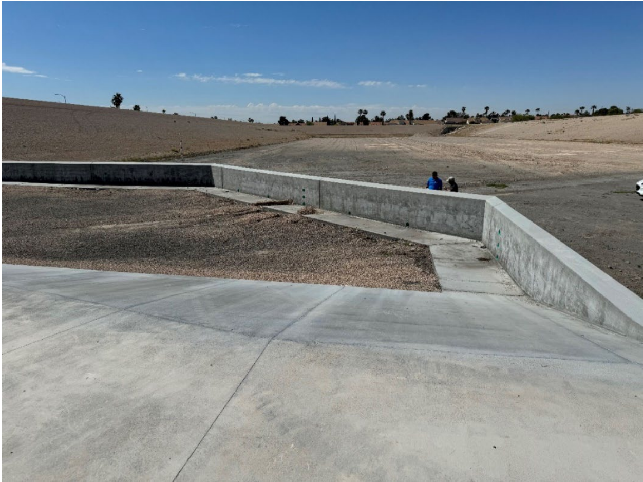
Figure 7. Low-flow feature at Oakey Detention Basin
