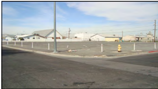
Asphalt sidewalk, light pole, bollard, and hydrant in sidewalk
