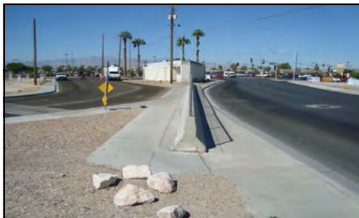
Concrete barrier in sidewalk path at Harrison Avenue
