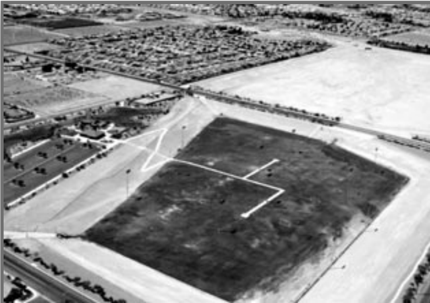
Flood detention basins at Gowan Road and Tenaya Way serve a secondary function as soccer fields.
