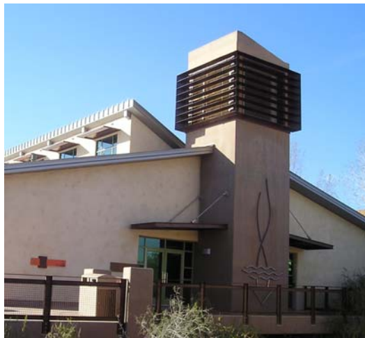
Evaporative cooling tower, Desert Living Center
