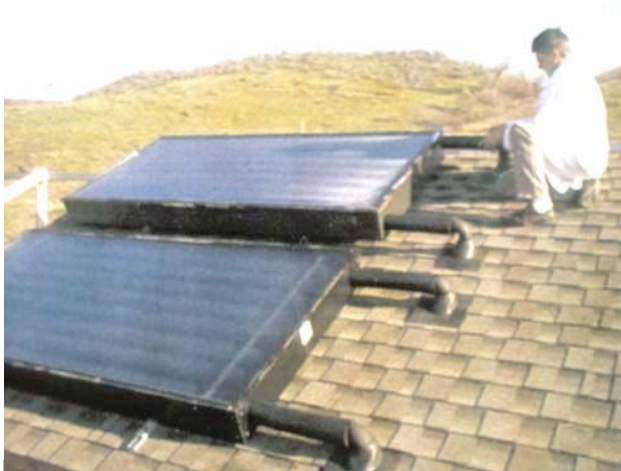
Solar water heating system (medium temperature solar thermal collector); source: azsolarcenter.co
