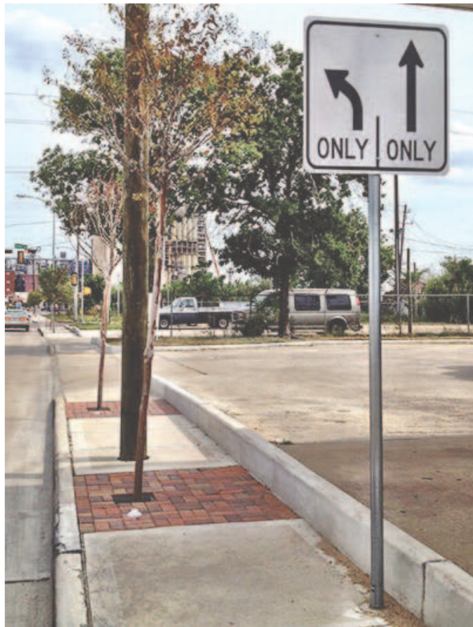
▲ Figure 158: Design error — sidewalk obstructions (photo: swamplot.com).
