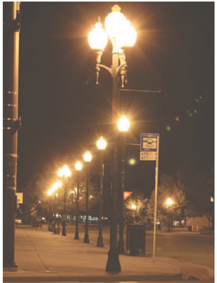
▲ Figure 156: Design error — more expensive lighting fixtures than necessary, contributing to light pollution (photo: flickr.com).
