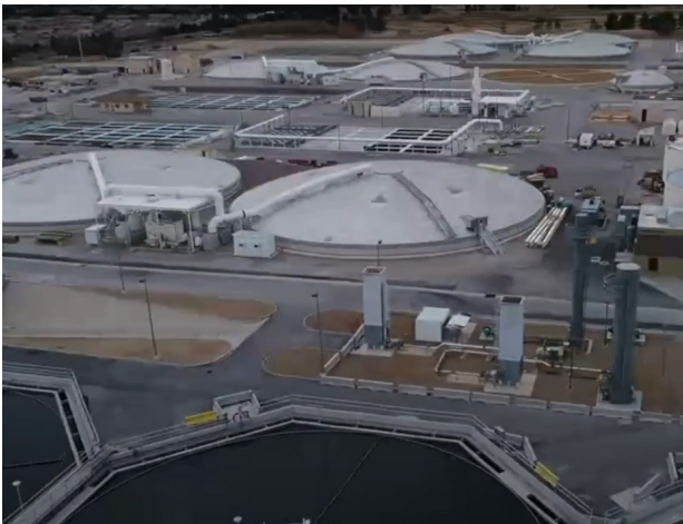
Las Vegas Water Pollution Control Facility
