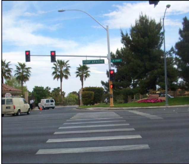
An existing Continental style crosswalk at the intersection of Fort Apache Road and Red Hills Road
