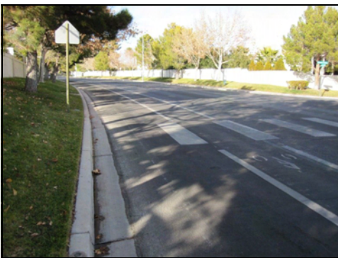
Crosswalk at Mariner Cove and Grand Canyon Drives without a curb cut and sidewalk
