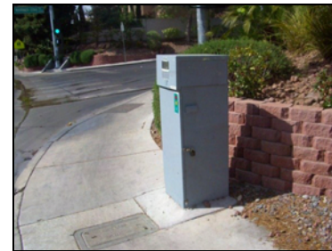
Utility boxes in the sidewalk path
