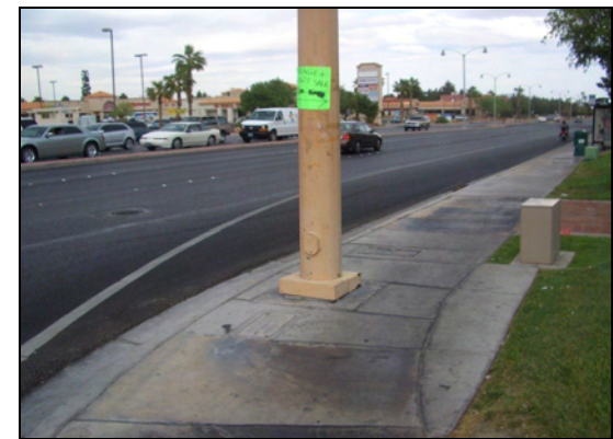
Streetlight pole obstructing the sidewalk
