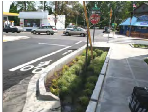
Using a complete street design in Tacoma, WA that incorporates stormwater management best practices. Source: Complete Streets Design Guidelines Project - City of Tacoma http://www.cityoftacoma.org/
