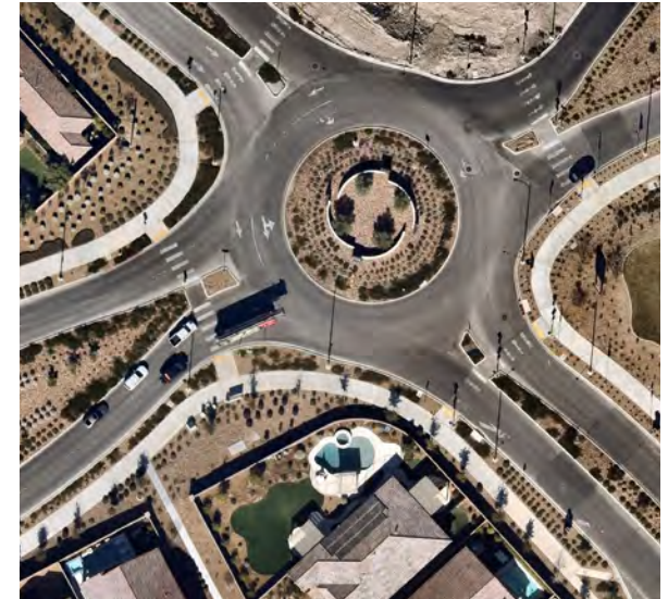
Roundabout, Via Inspirada
