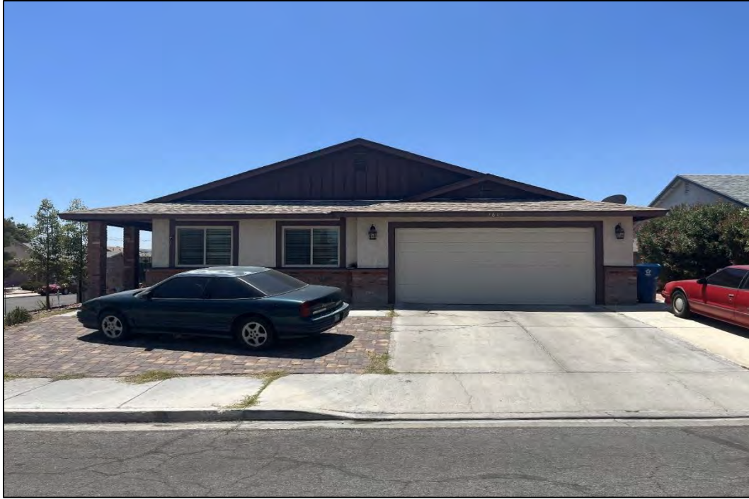
Photograph 57. North façade of the Ranch-style home with square plan at 3605 Briarglen Lane, facing south (North Wind 2023).
