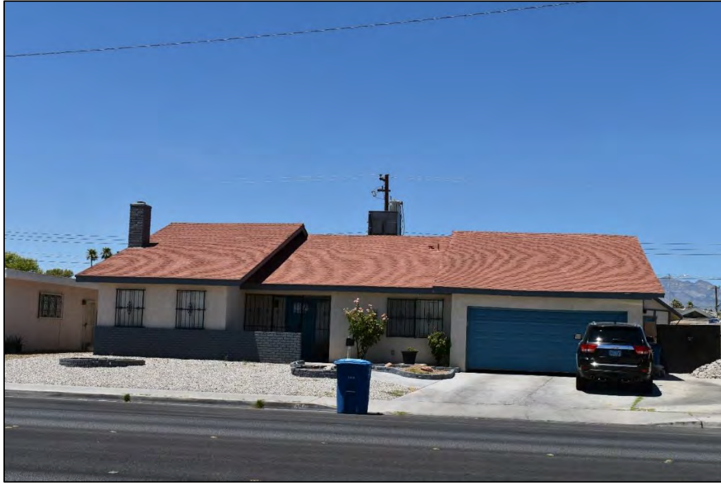
Photograph 39. East façade of the Ranch-style home at 717 N. Valley View Boulevard, facing west (North Wind 2023).
