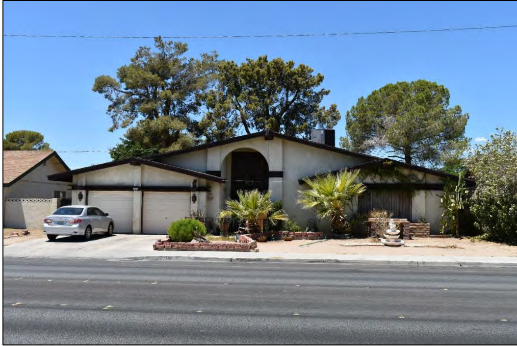
Photograph 41. West façade of the Spanish Ranch-style home at 705 N. Valley View Boulevard, facing east (North Wind 2023).
