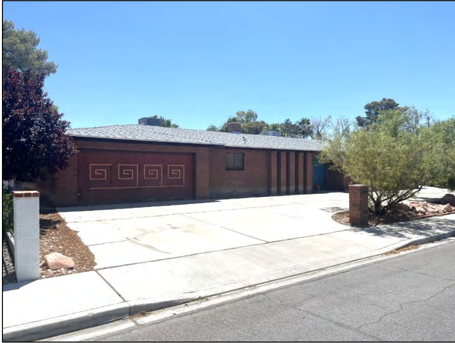
Photograph 62. West façade of the custom, Contemporary Ranch-style home at 1008 Oak Tree Lane, facing southeast (North Wind 2023).
