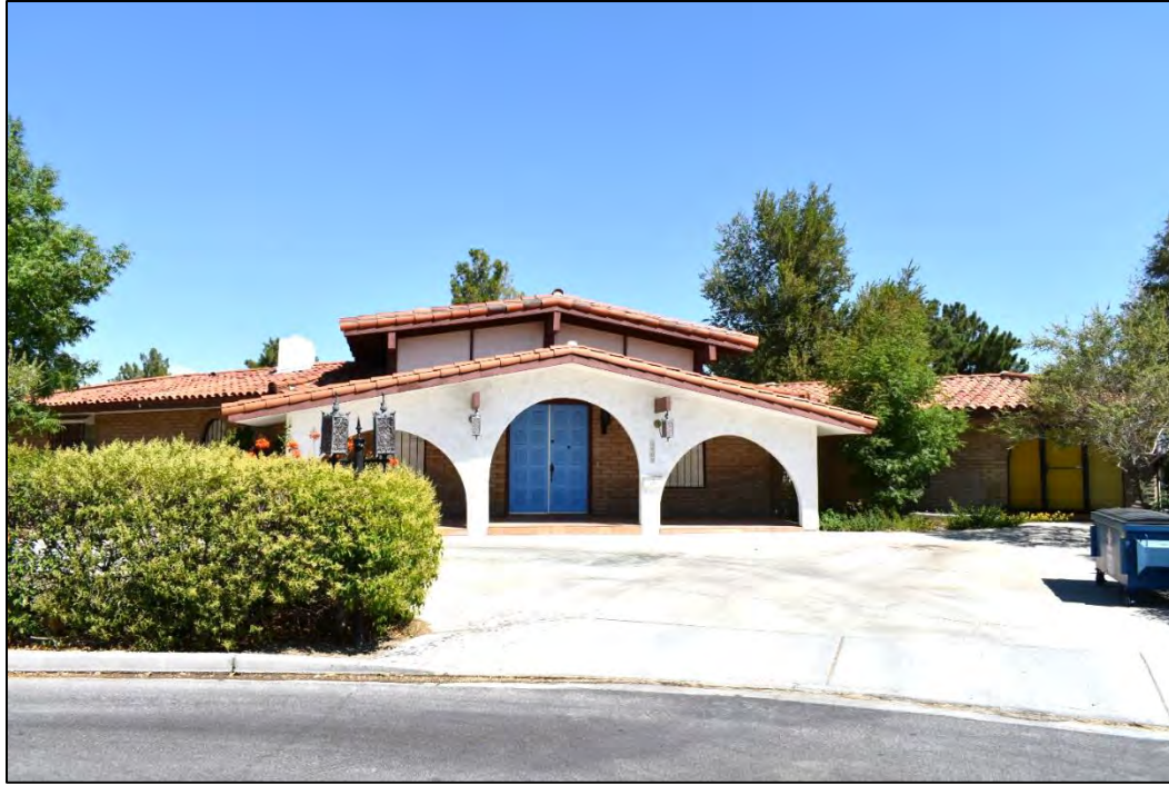
Photograph 34. South façade of the Spanish Ranch-style home at 3800 Fairway Circle, facing north. Note the single-leaf glass entry with side-lites on the far right (east) end of the main façade, indicating a possible garage infill. Otherwise, the home is believed to be mostly intact (North Wind 2023).
