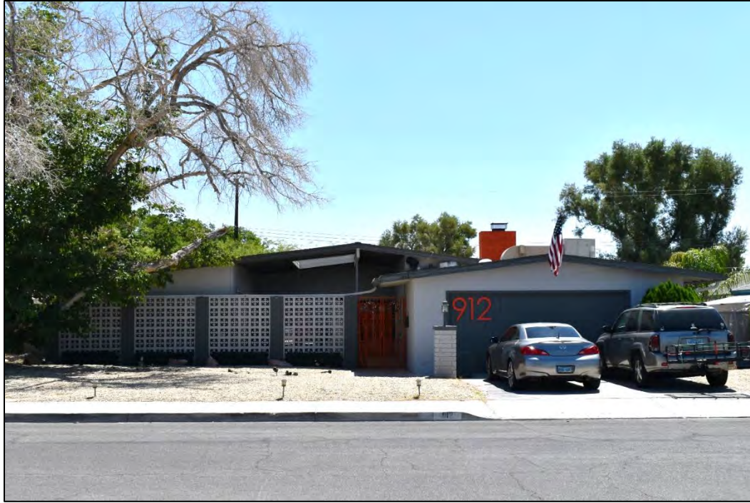
Photograph 31. West (front) façade of 912 Niblick Drive, facing east. This home is an example of the front gable type of the Contemporary Ranch style within the subdivision. Note the central, recessed porch, breezeblock wall, projecting roof beams, and carriage lamp (North Wind 2023).
