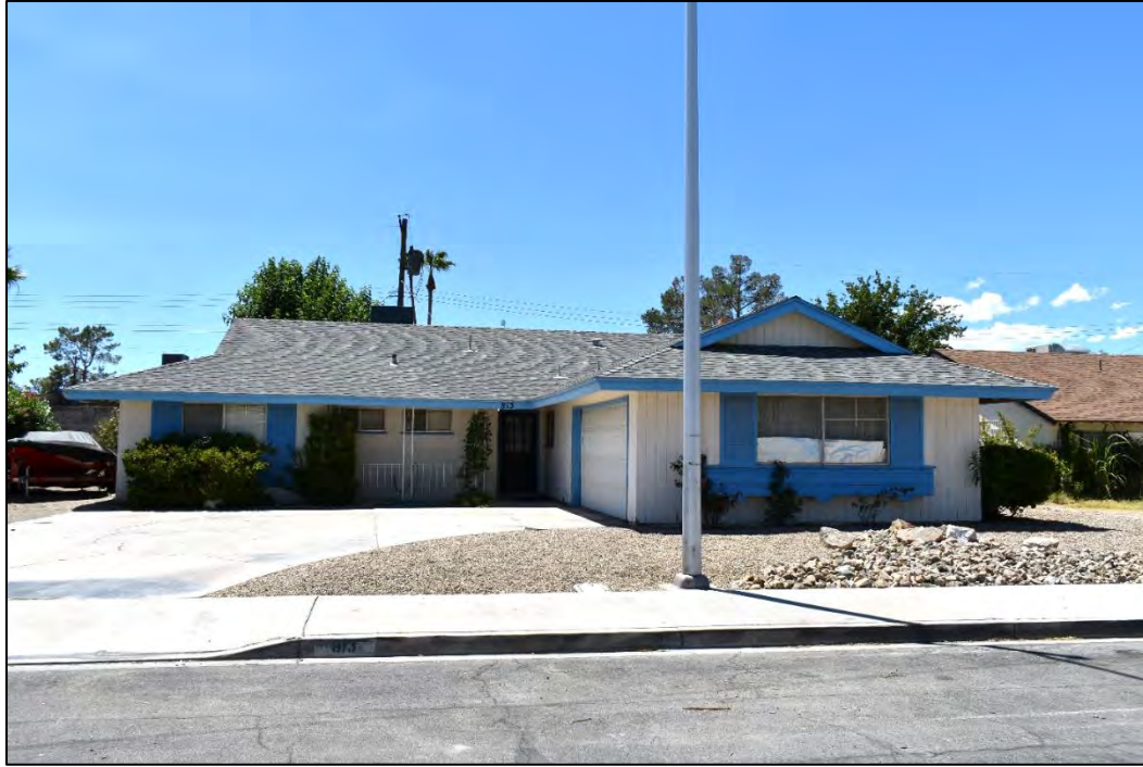
Photograph 35. East façade of the Ranch-style home at 825 Langtry Drive, facing west. The garage on this home faces the driveway and contains a boxed window with brackets and shutters on the street-facing façade of the garage. This home retains the original windows and vertical siding (North Wind 2023).
