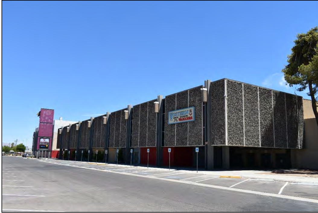
Photograph 8. View of the original portion of Western High School, located at 4701 W. Bonanza Road, facing southeast. Note the pebbledash exterior of the building (North Wind 2023).
