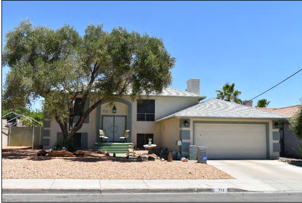
Photograph 52. West façade of the New Traditional – Italian Renaissance-style home at 712 Langtry Drive, facing east. The New Traditional elements include the massing, quoining, and arched entry. Note the asymmetrical treatment of shutters (North Wind 2023).
