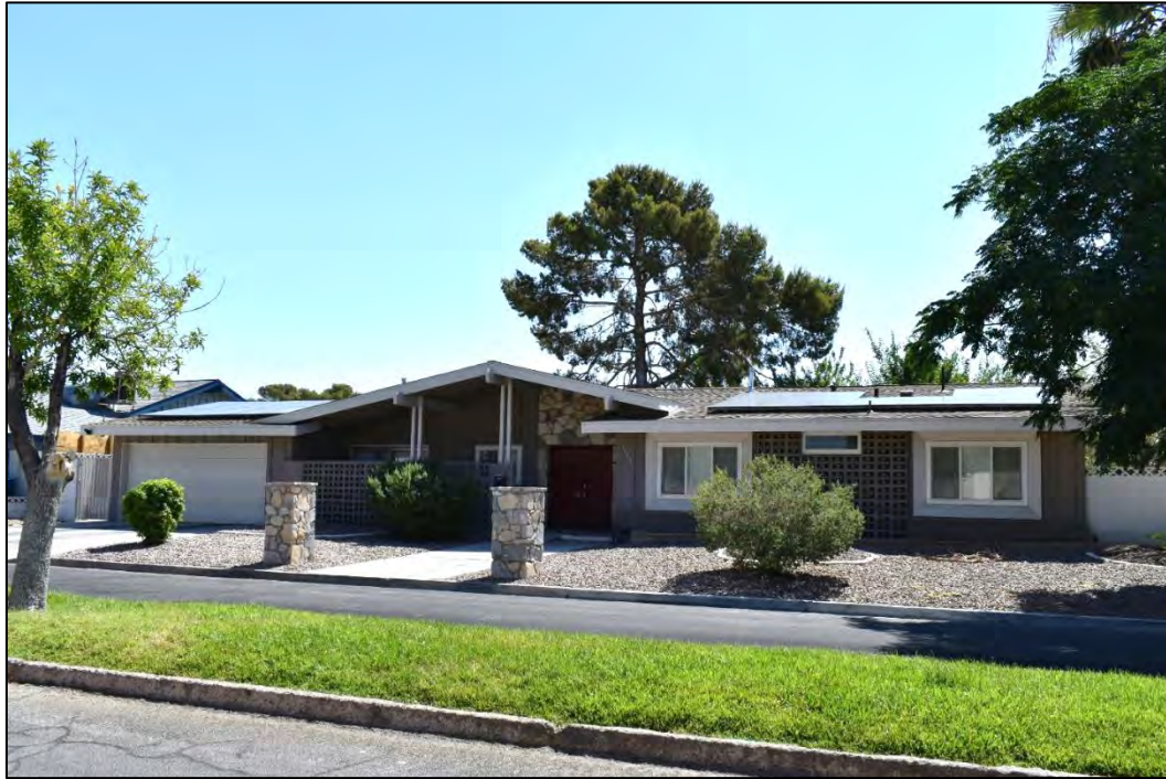
Photograph 30. West (front) façade of 1104 Ironwood Drive, facing east. This home is a cross-gable example of the Contemporary Ranch style with recessed center porch, breezblock wall, stone accents, and extended roof beams. Note the original aluminum-frame windows and wood shake roof have been replaced with vinyl-frame windows and composition shingle (North Wind 2023).
