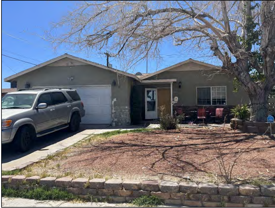
Photograph 21. East façade of 205 Eldorado Canyon Street, facing southwest. This home represents the two front-facing gable type with flat-roof porch. The stone veneer and vinyl-framed windows are not original to the home (North Wind 2023).
