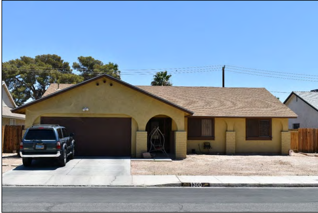
Photograph 59. West façade of the Spanish Ranch-style home at 1300 Woodbridge Drive, facing east (North Wind 2023).
