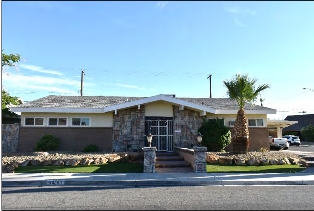
Photograph 48. The south façade of the Contemporary Ranch-style home at 4200 Snead Drive, facing north. The windows, roof sheathing, and decorative metal gate are believed to be alterations (North Wind 2023).
