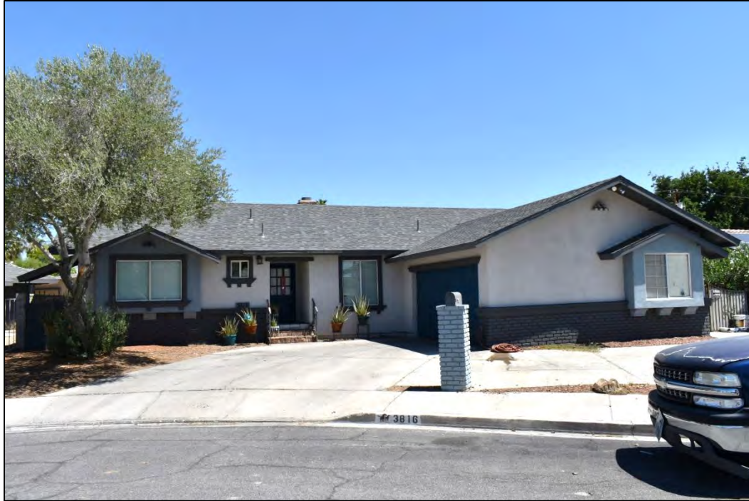
Photograph 33. South (main) façade of the Storybook Ranch-style 3816 Golf Lane, facing north. Note the boxed windows with small gable roofs and brackets. Decorative vergeboards at gable ends have been replaced with plain fascia, and original aluminum-frame windows have been replaced with vinyl windows. Additionally, this home likely had vertical siding where stucco is now extant (North Wind 2023).
