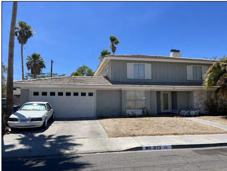
Photograph 42. East façade of the “Masters” model Raised Ranch-style home at 813 Chabot Drive, facing west. This home retains the original board-and-batten siding and stone veneer, and stone planter near the main entry. The roof sheathing and windows have been replaced (North Wind 2023).
