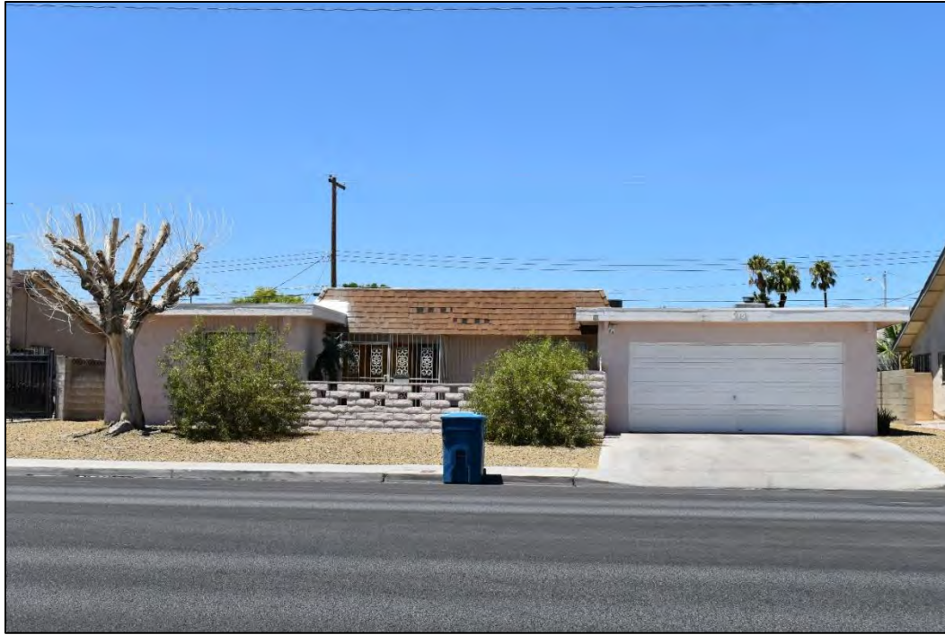
Photograph 50. East façade of the Mansard-style home at 713 N. Valley View Boulevard, facing west. This home is unique in the neighborhood, having a U-shaped plan and only one story (North Wind).
