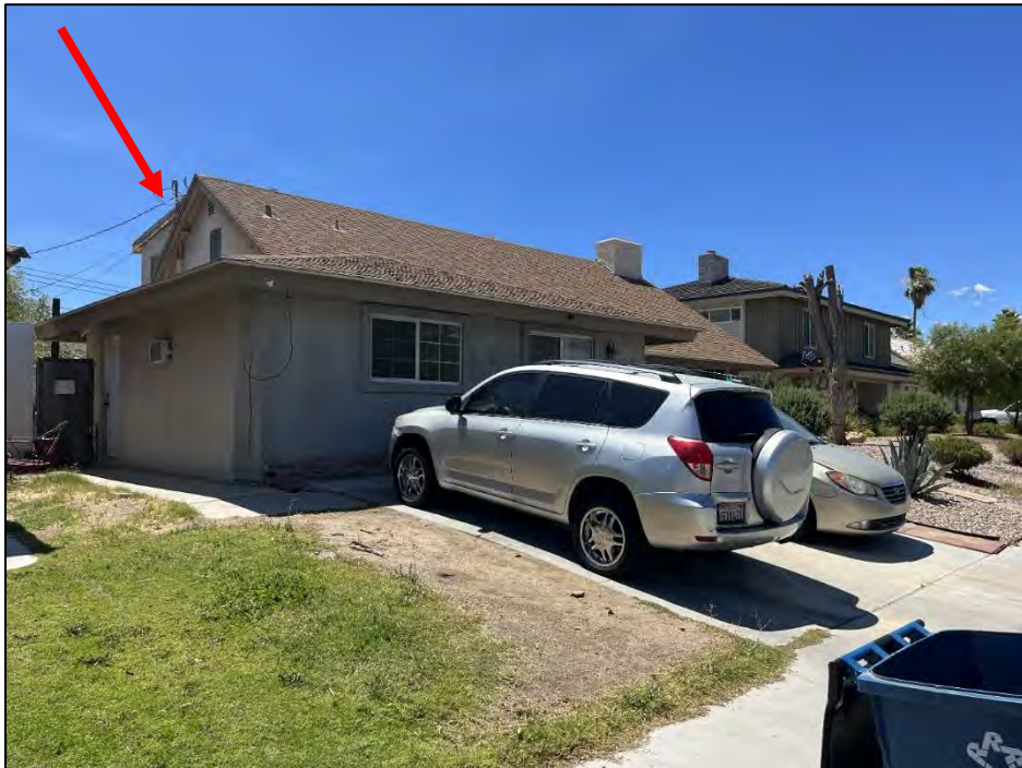
Photograph 38. Northeast (main) and southeast (side) facades of 801 Chabot Drive, showing the shed-style roof, denoted by the red arrow, over the rear façade (North Wind 2023).
