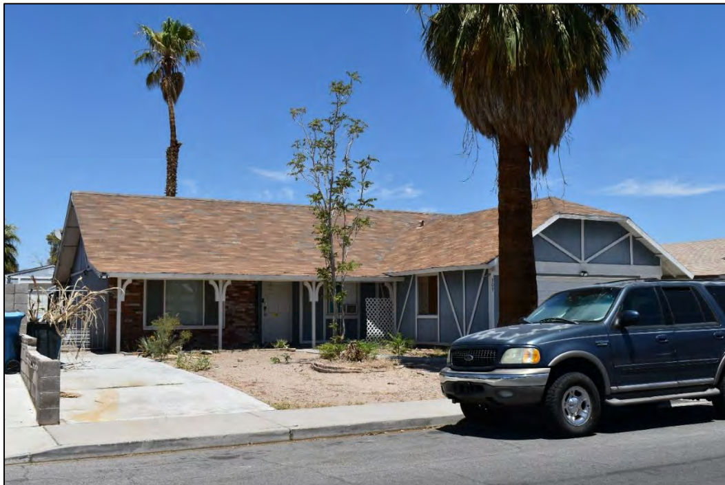
Photograph 45. Southeast façade of the one-story, jerkinhead roof variant of the Tudor Ranch-style home at 309 Estella Avenue, facing northwest (North Wind 2023).
