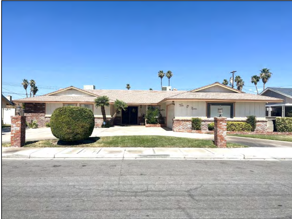
Photograph 28. East façade of 1009 Ironwood Drive, facing northwest. Note the U-shaped plan with low-pitched roof, variations in siding and brick veneer, the recessed, double-leaf entry, and the brick carriage lights. Note the window on the east façade of the garage, and the original wood shake roof, has been replaced (North Wind 2023).
