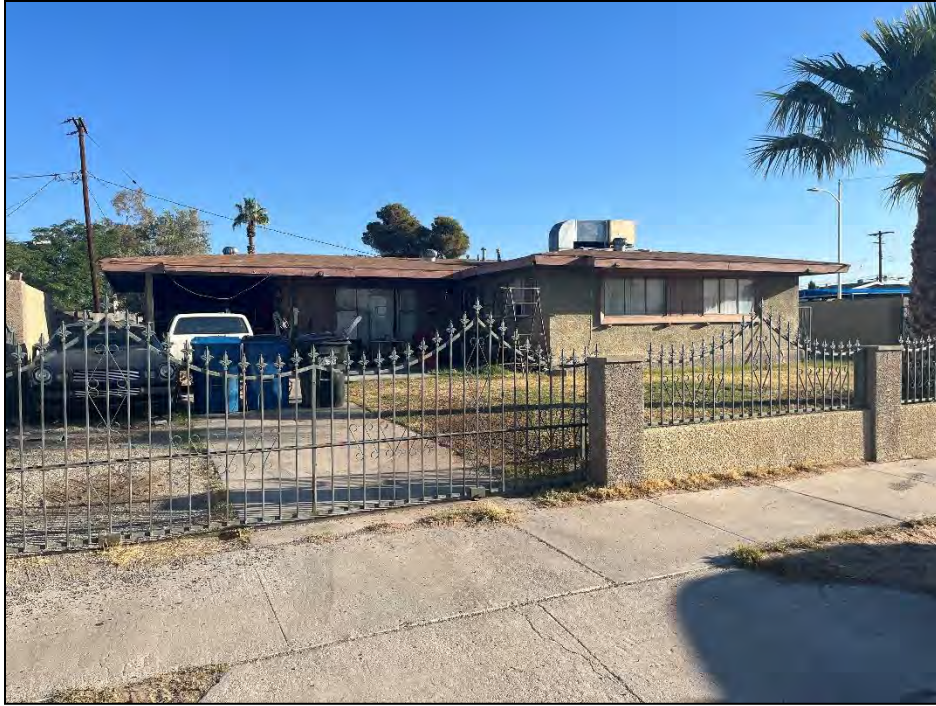
Photograph 1. View of the house at 3300 Turquoise Road, facing north. This house is an example of the cross-hipped roof subtype of the Ranch architectural style (North Wind 2023).
