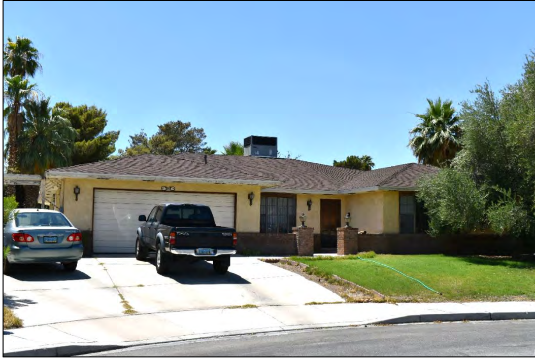
Photograph 56. North façade of the Ranch-style home at 3713 Bridge Glen Drive, facing south. This home is an example of the U-shaped plan with hipped roof and multi-lite bay windows (North Wind 2023).
