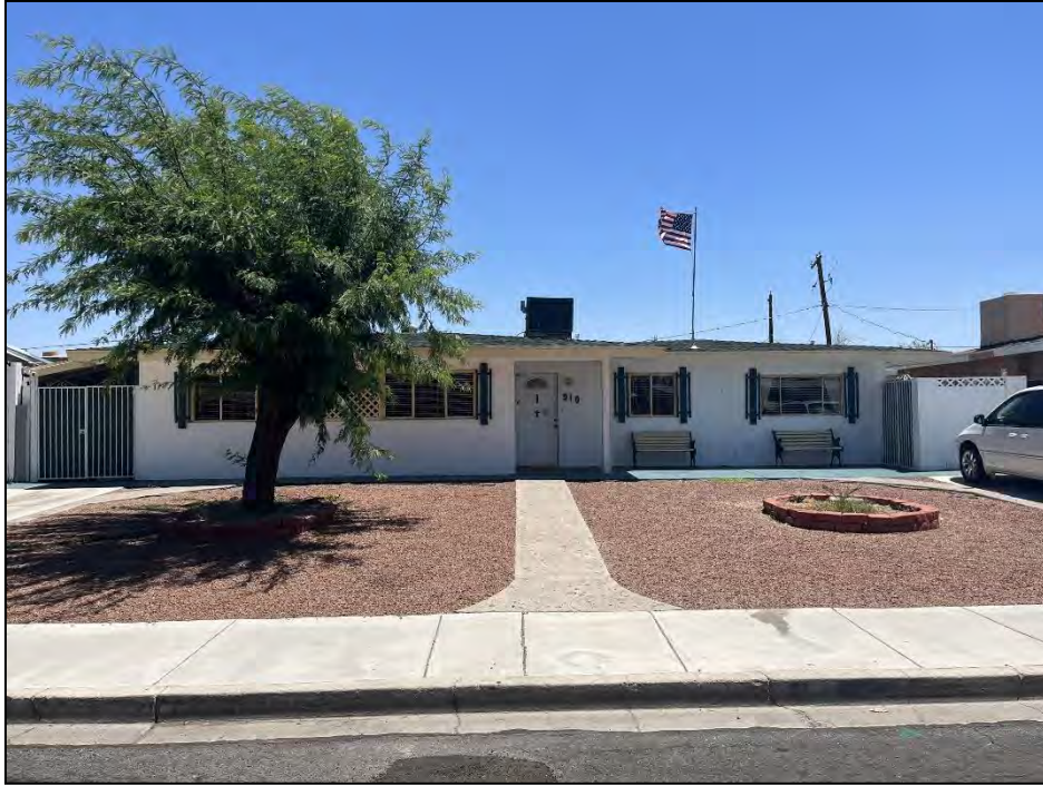
Photograph 10. View of the Ranch style residence at 910 Baker Avenue in Heers Subdivision Nevada 1, facing east. This house is an example of the “Capri Modern” plan (North Wind 2023).
