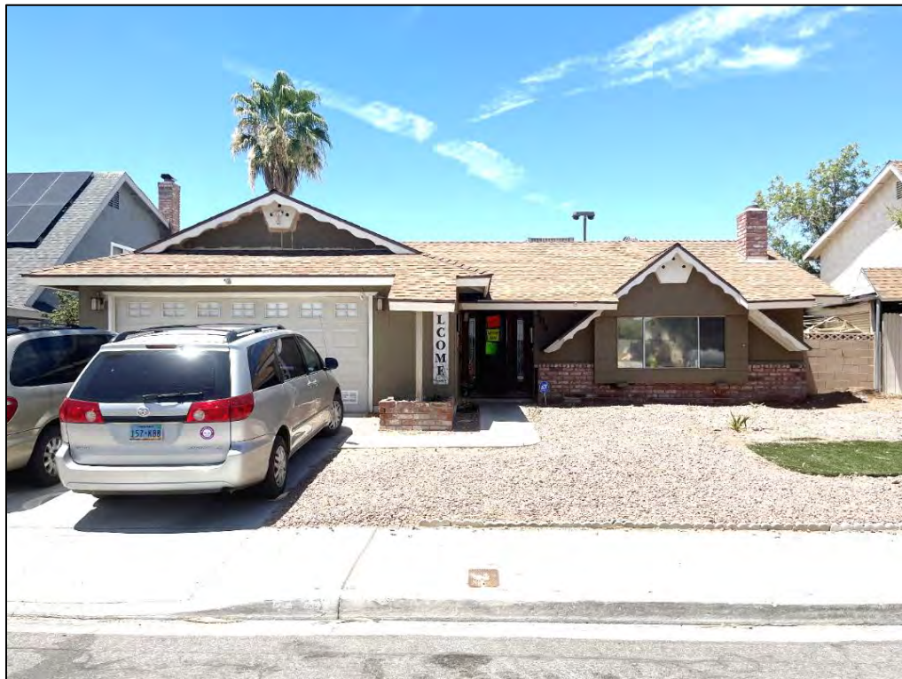
Photograph 40. East façade of the Storybook Ranch-style home at 309 Horn Street, facing west. The wood shake roof has been replaced with composition shingle. Note the brick planter to the right (north) of the garage door (North Wind 2023).
