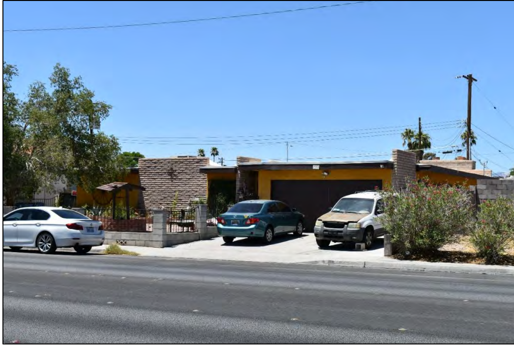
Photograph 47. East façade of the Contemporary Ranch-style home at 721 N. Valley View Boulevard. This home is believed to be a custom design (North Wind 2023).
