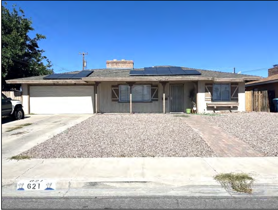
Photograph 17. East façade of the Ranch-style home at 621 Helyne Street, facing west. This is an example of the rectangular plan home with its original board-and-batten siding, wood shutters, and bracketed window box (North Wind 2023).
