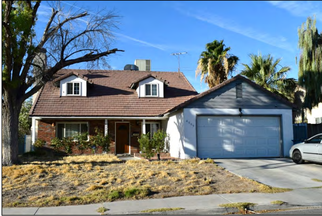
Photograph 54. North façade of the Colonial Revival-style home at 4009 Fortune Avenue, facing south. This home has replaced the original wood shake shingles with concrete tile, and the original steel casement windows with vinyl-frame sliding windows (North Wind 2023).
