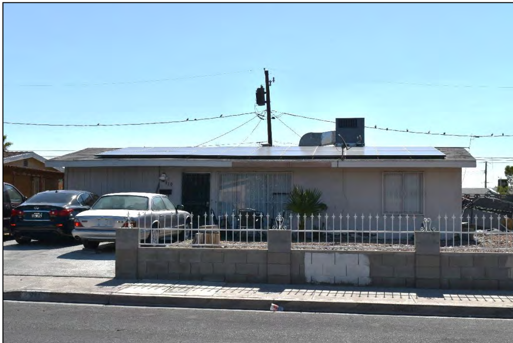
Photograph 15. View of the Ranch style residence at 910 Magnolia Avenue in Heers Subdivision Nevada 1, facing east. Note the alterations to the “Nevada Ranch House” plan (North Wind 2023).
