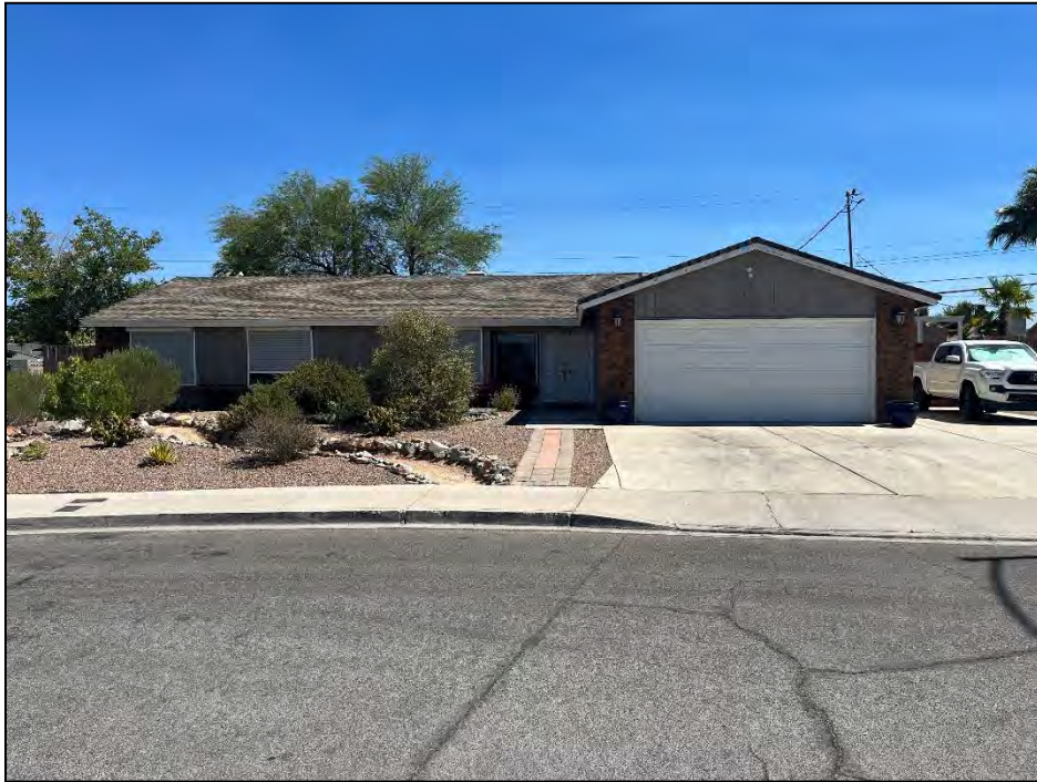
Photograph 63. View of the Ranch style residence located at 701 Glen Abbey Circle in The Priory, showing L-shaped plan and combination front gable and side-gabled roof, facing southeast (North Wind 2023).
