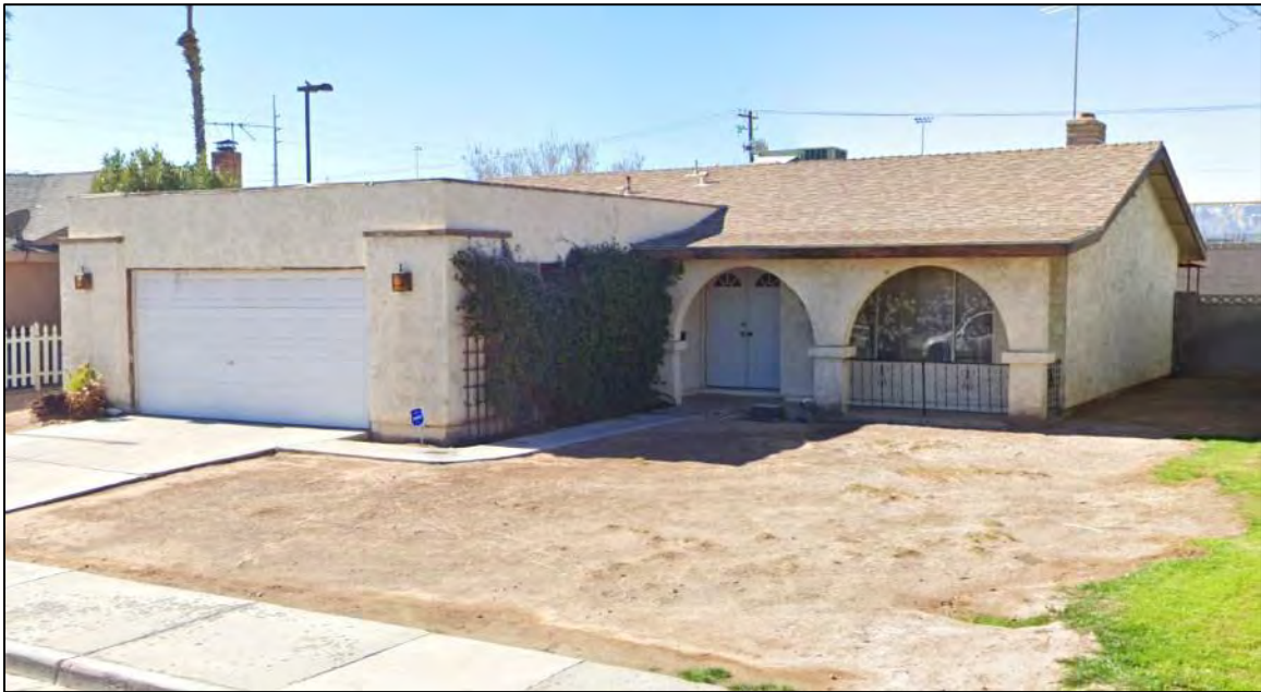
Figure 62. East façade of the Spanish Ranch-style home at 301 Horn Street, facing southwest. Other examples of this model have a window on the side of the garage, facing the front yard. The home retains the original stucco exterior and front window (Google Streetview 2023).
