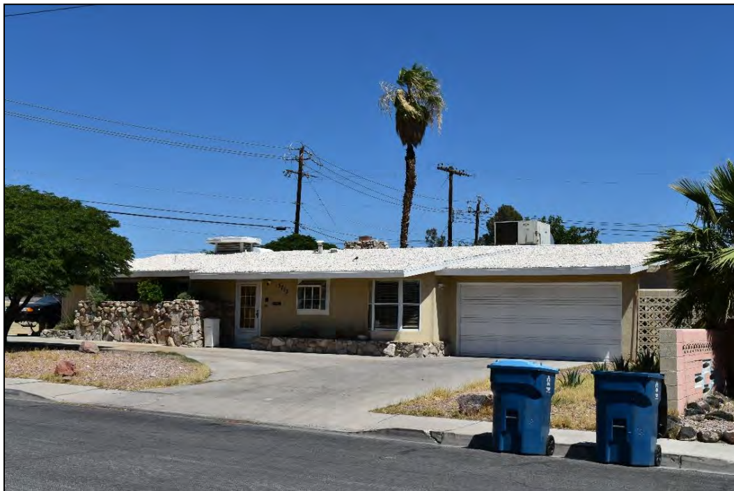
Photograph 2. View of the house at 3712 Apache Lane, facing northwest. This house is an example of the side-gabled roof subtype (with original rock roof) of the Ranch architectural style (North Wind 2023).
