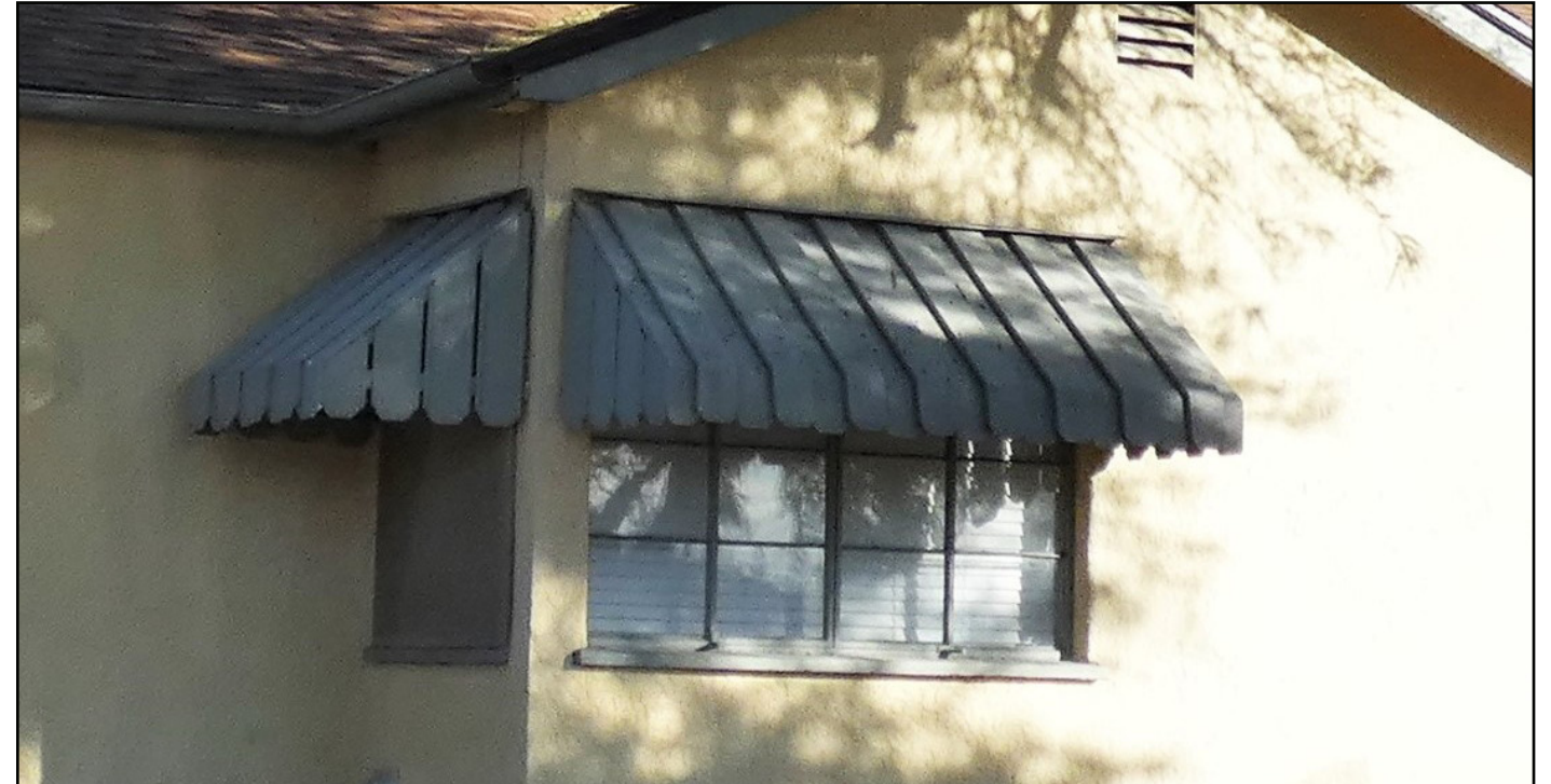
Image 27: Recommend retention of early wood awnings.
