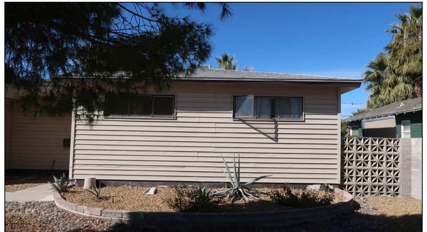
Image 21: Example of vinyl siding.
