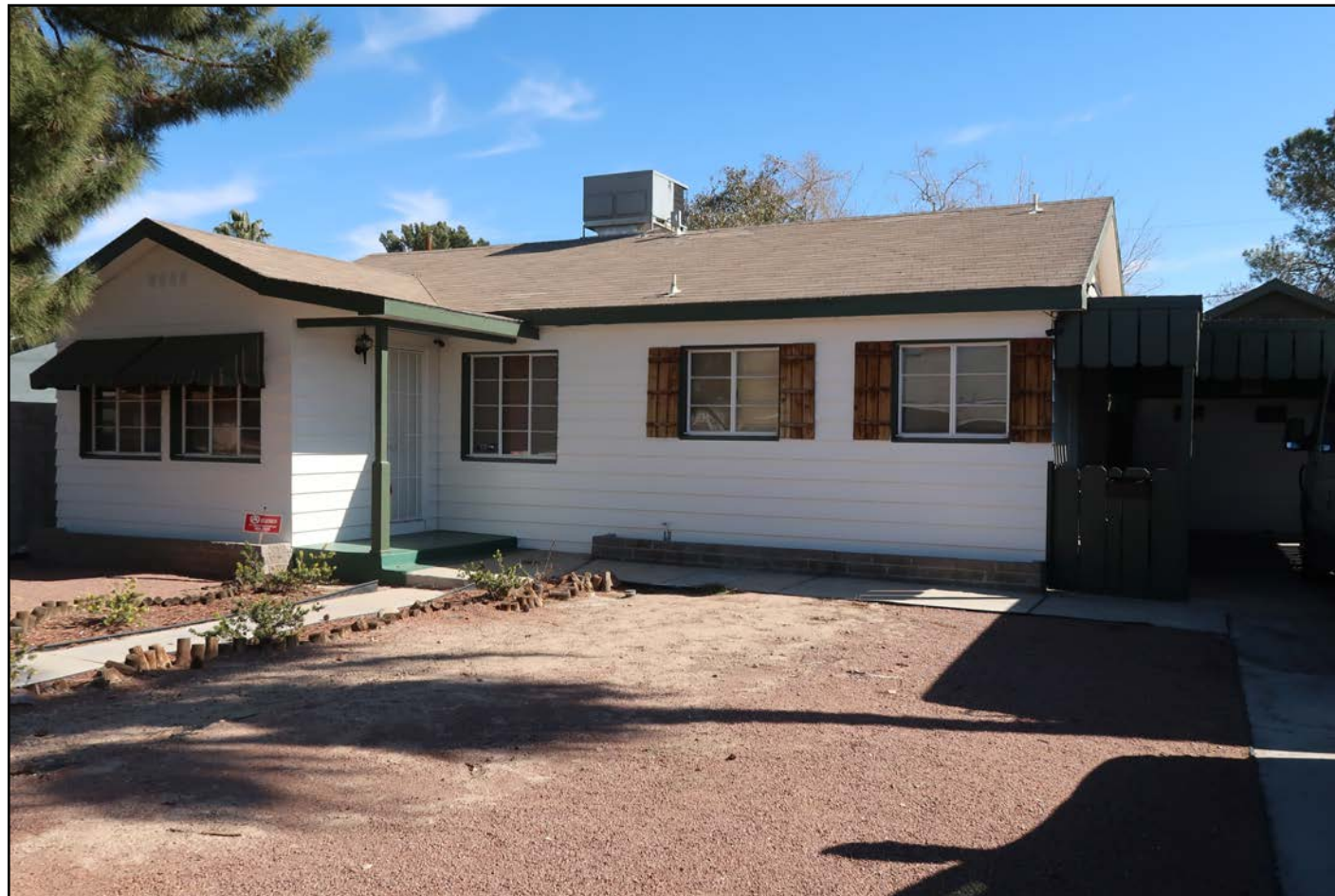
Image 10: Recommended example of in-kind replacement of windows.
