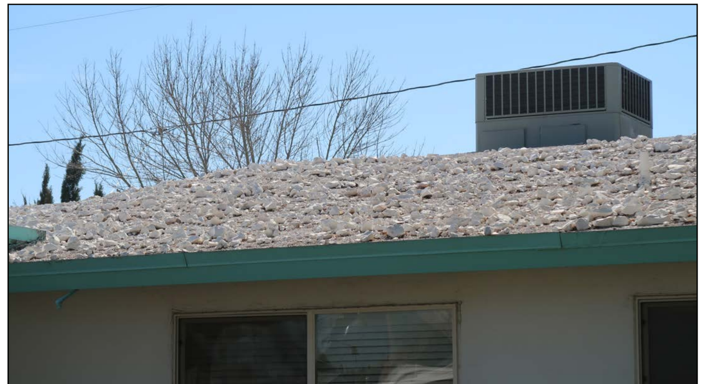
Image 5: Recommend retention of historic rock roof.
