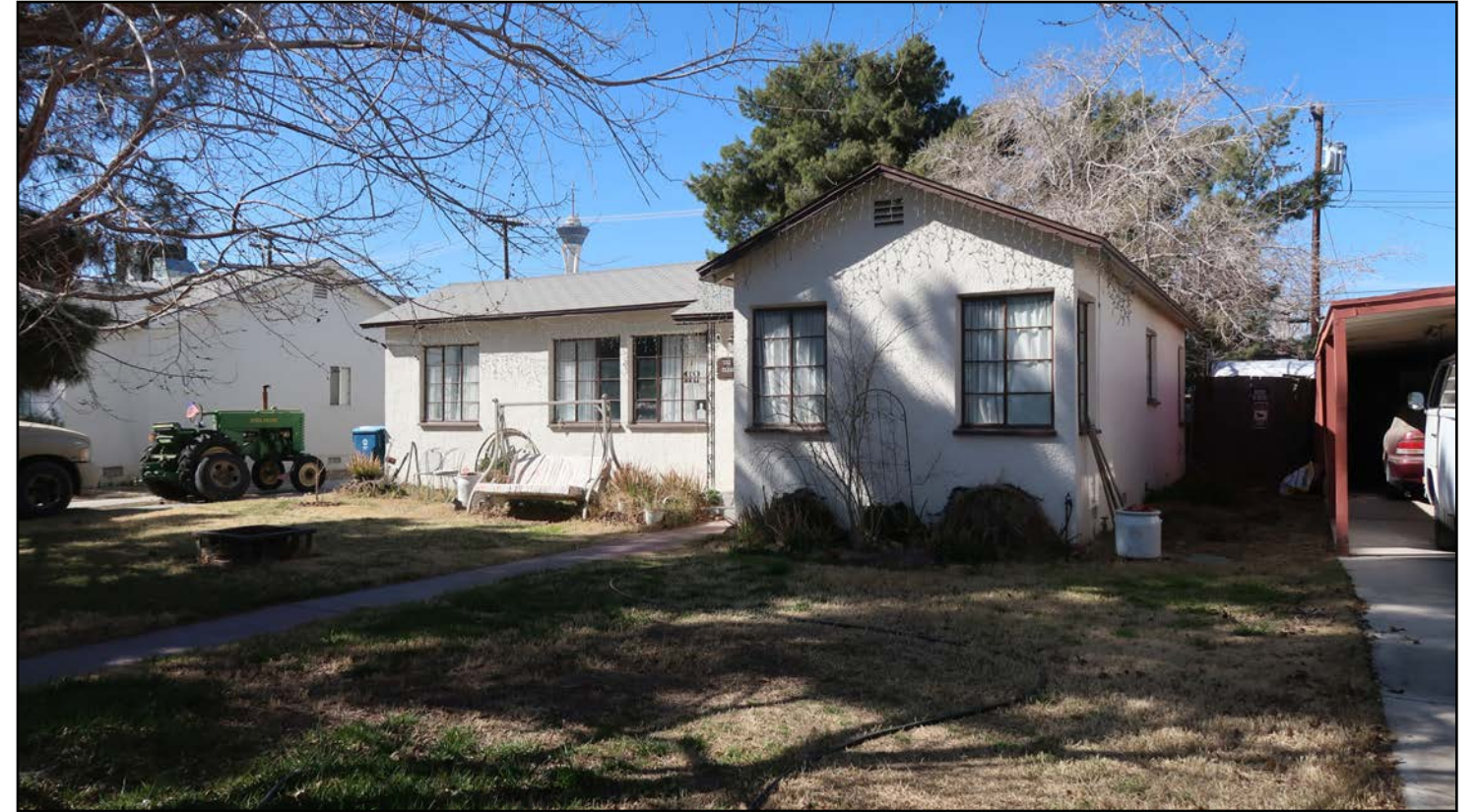
Image 9: Recommend retaining historic windows whenever possible.
