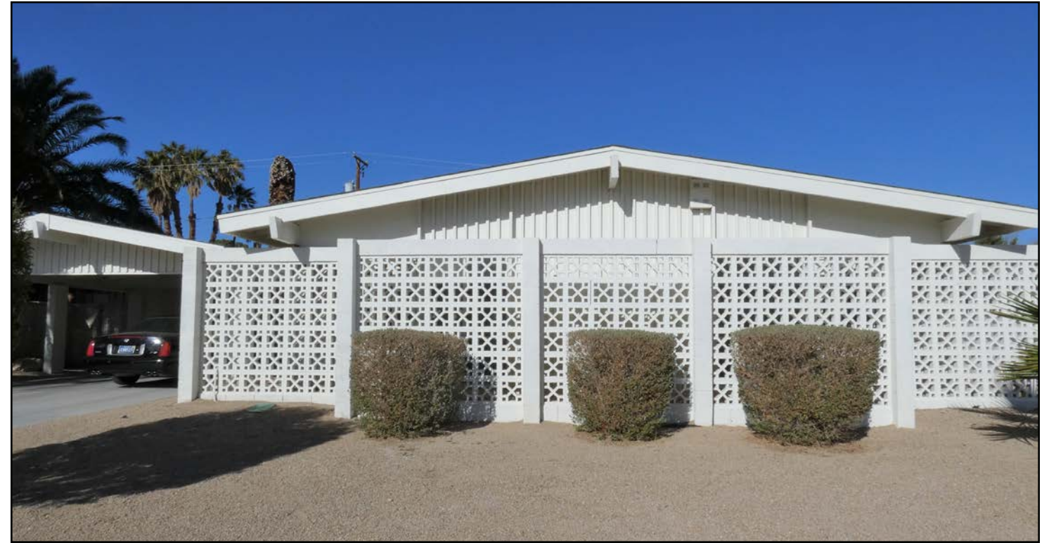
Image 2: Recommended enclosure that is compatible and reversible without removing or altering character-defining features.
