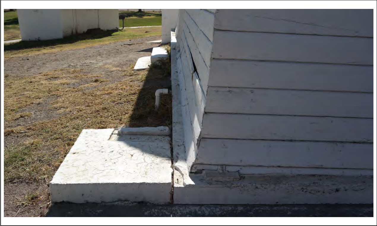
Water Tower – Foundation detail, northeast corner Kautz Environmental Consultants, Inc., November 2024
