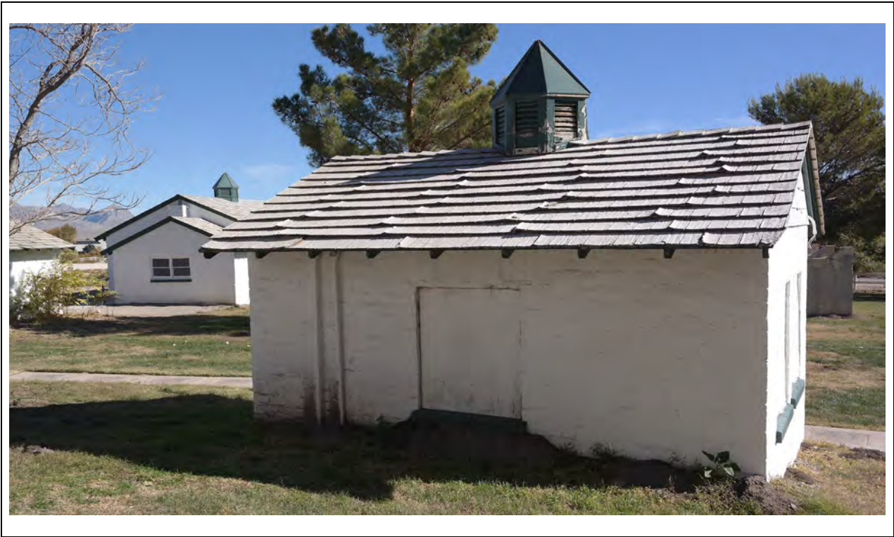
Power House – Northwest elevation and west corner Kautz Environmental Consultants, Inc., November 2024
