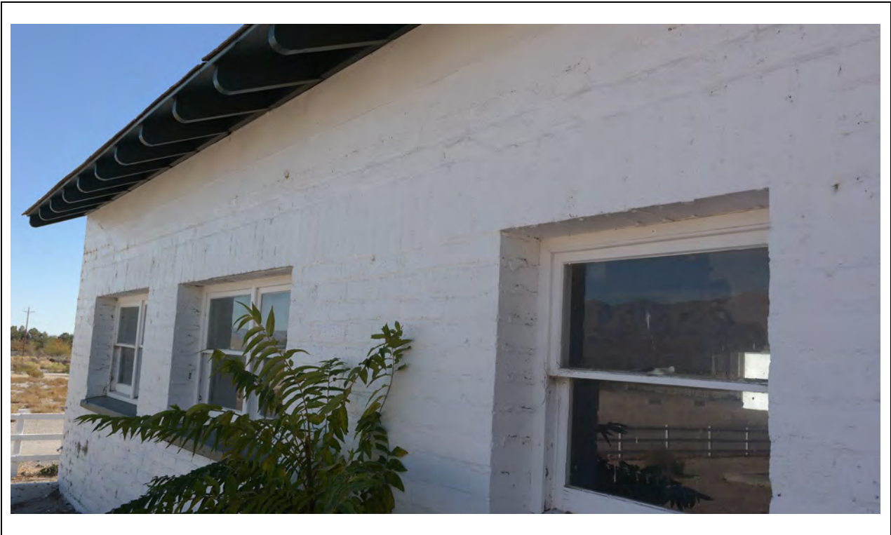
Generator Building – North elevation window detail Kautz Environmental Consultants, Inc., November 2024
