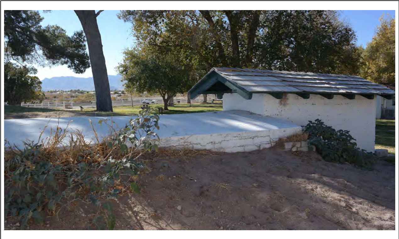
Root Cellar – Northeast elevation and east corner Kautz Environmental Consultants, Inc., November 2024
