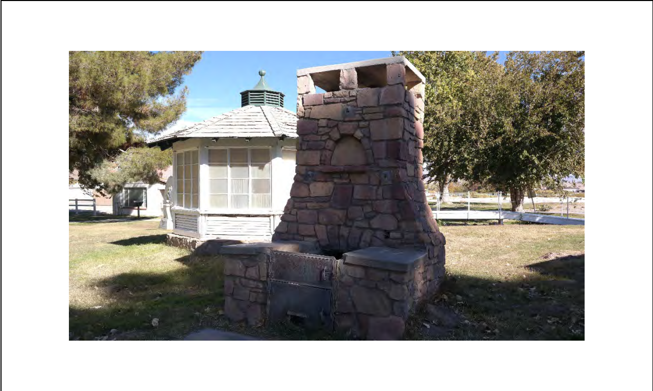
Outdoor Fireplace – West elevation and southwest corner Kautz Environmental Consultants, Inc., November 2024
