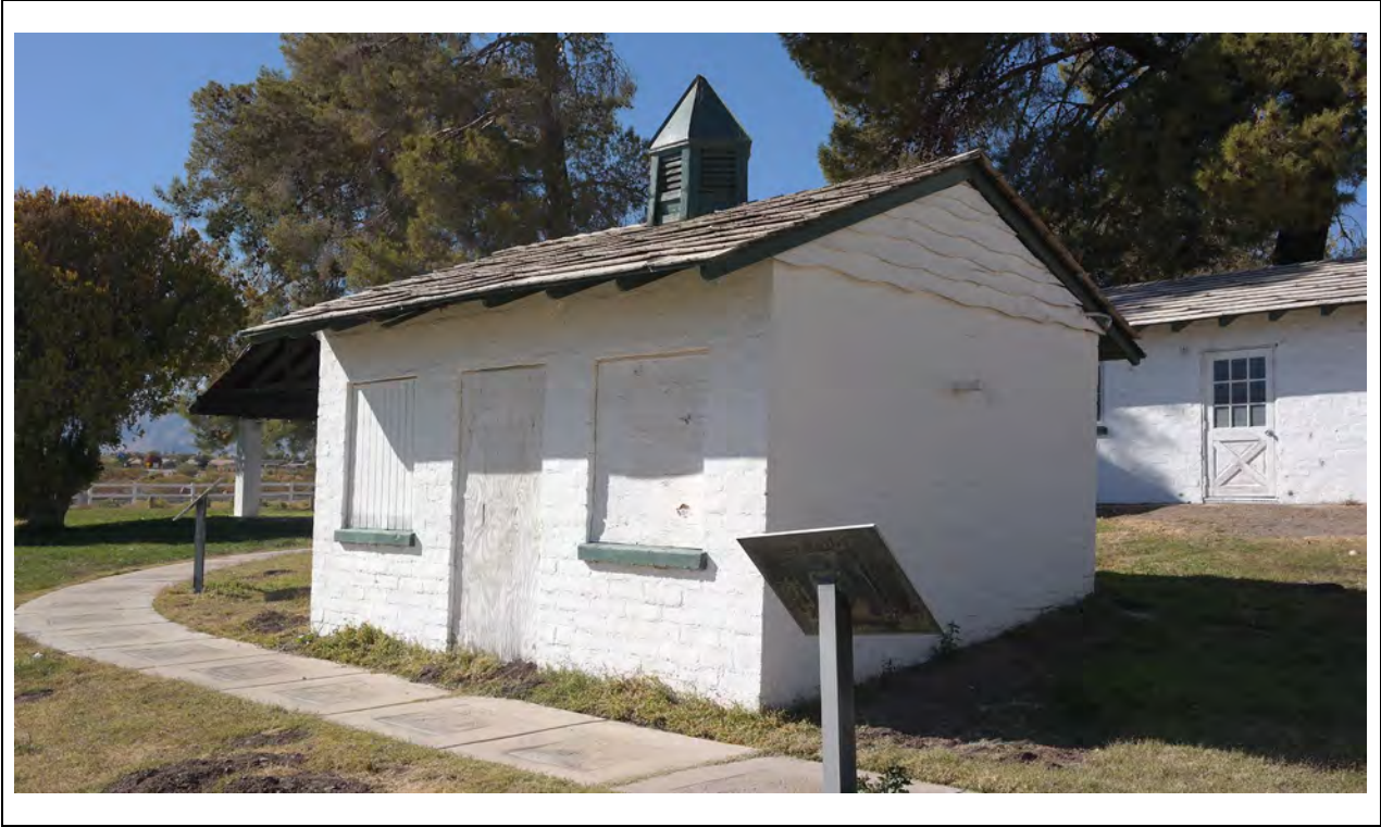
Power House – East corner Kautz Environmental Consultants, Inc., November 2024
