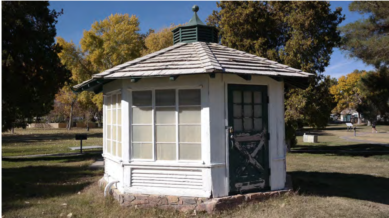
Pump House – Southeast elevation
