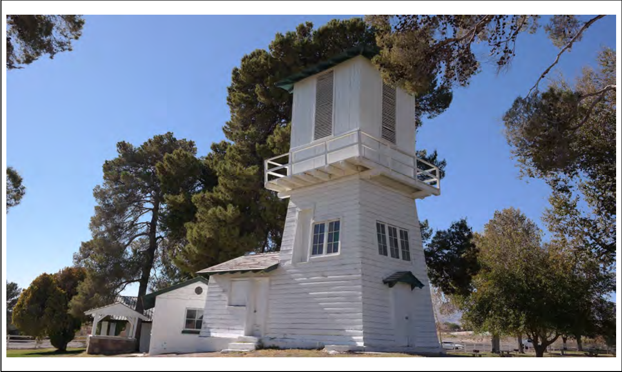
Water Tower – Northeast corner Kautz Environmental Consultants, Inc., November 2024
