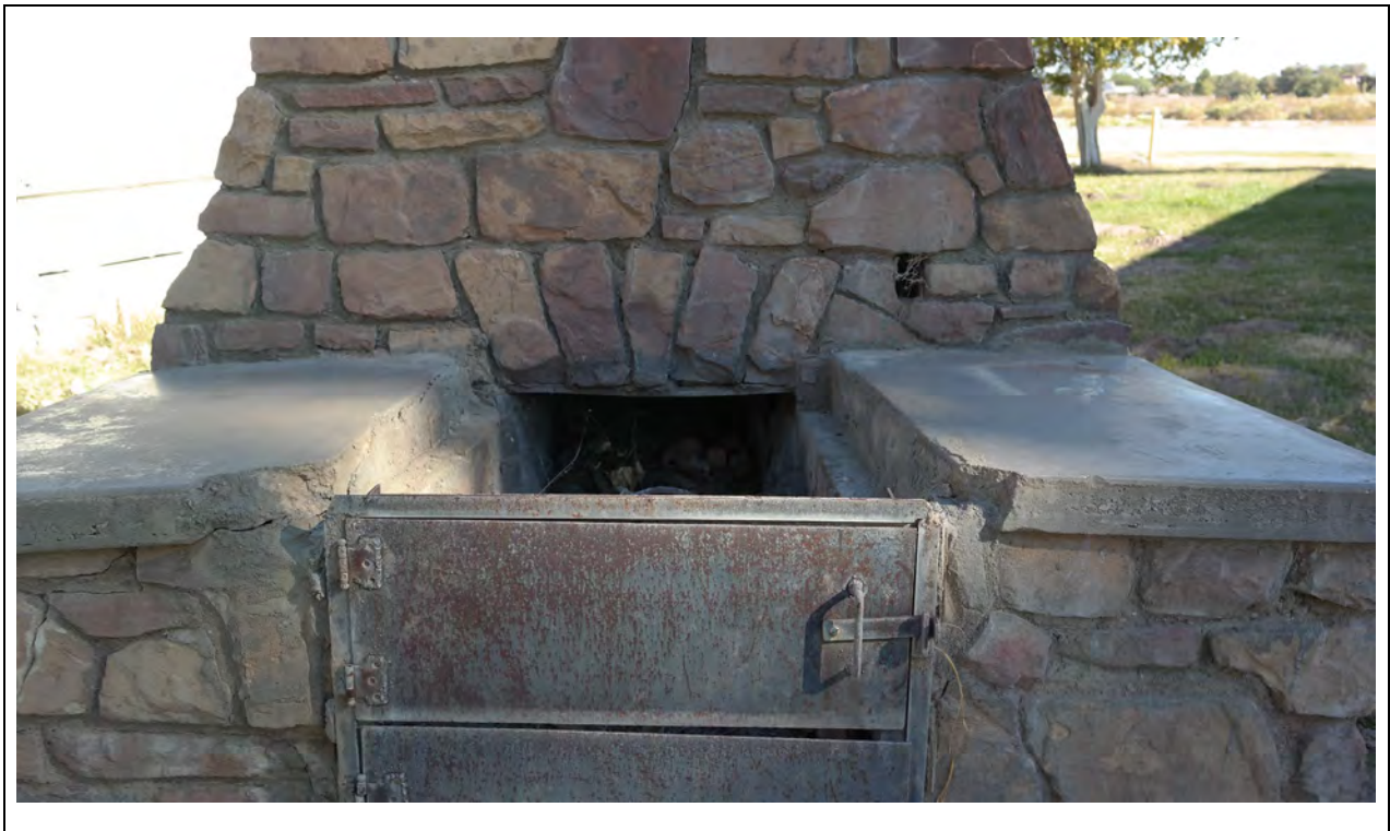
Outdoor Fireplace – Concrete detail Kautz Environmental Consultants, Inc., November 2024
