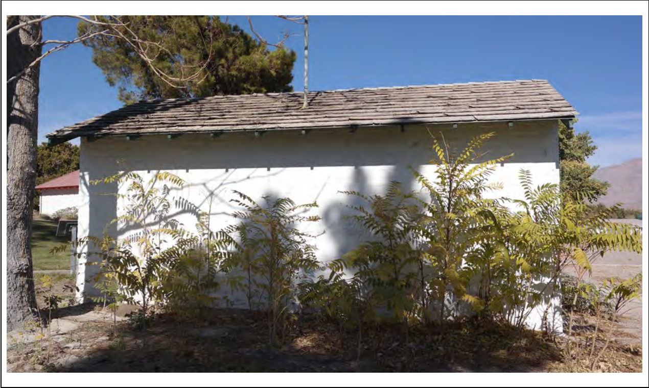
Bath House – South elevation Kautz Environmental Consultants, Inc., November 2024
