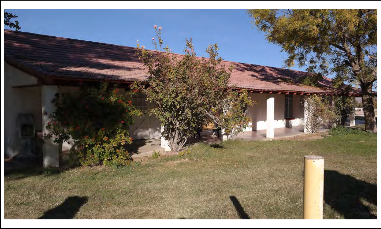
Guest House – South elevation Kautz Environmental Consultants, Inc., November 2024
