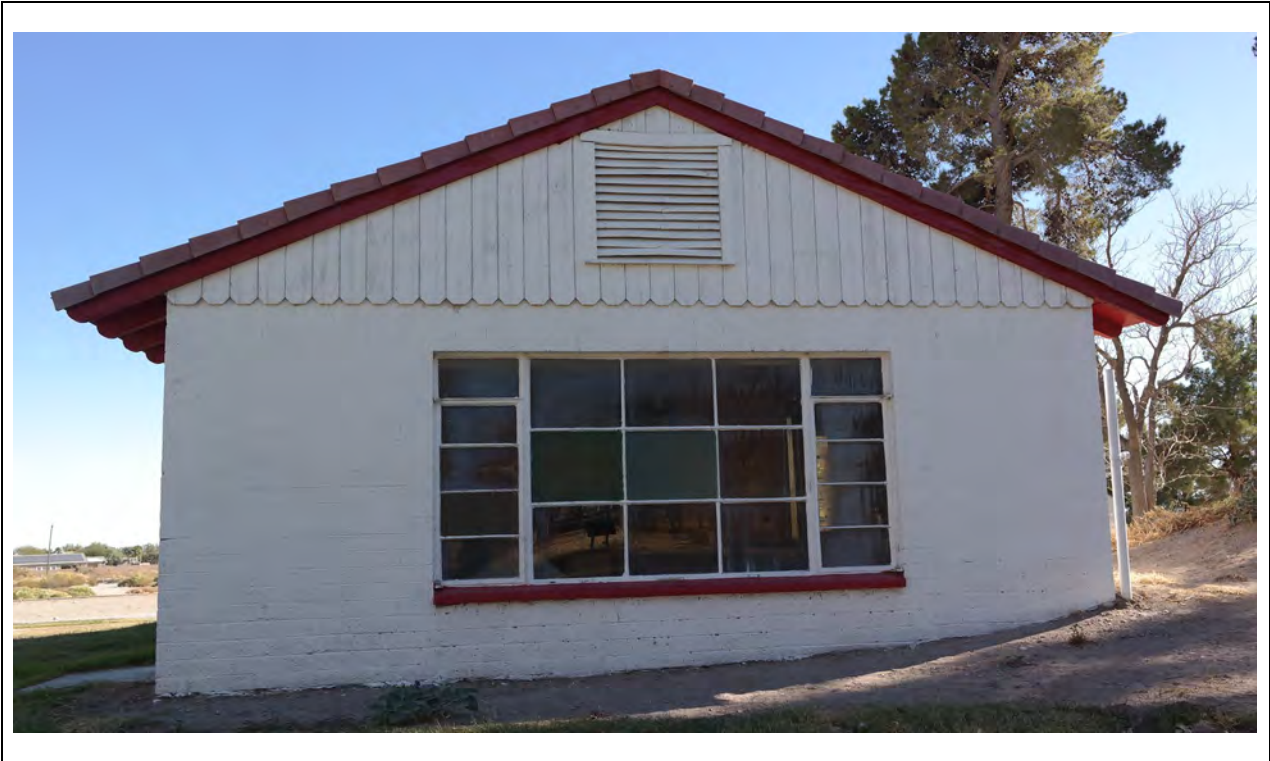
Duplex – Northwest elevation Kautz Environmental Consultants, Inc., November 2024
