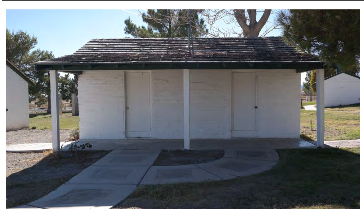
Bath House – North elevation
