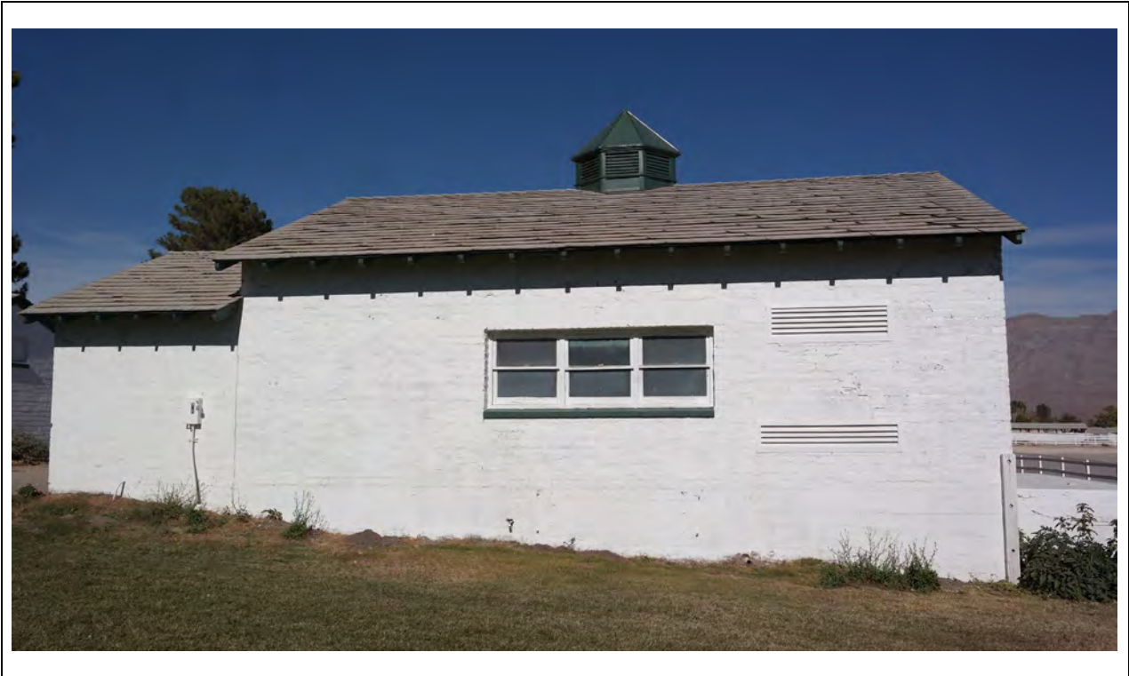
Generator Building – South elevation Kautz Environmental Consultants, Inc., November 2024
