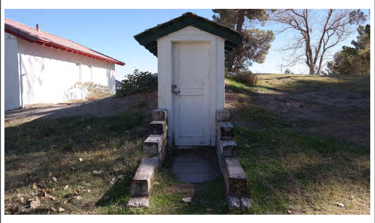
Root Cellar – Northwest elevation Kautz Environmental Consultants, Inc., November 2024
