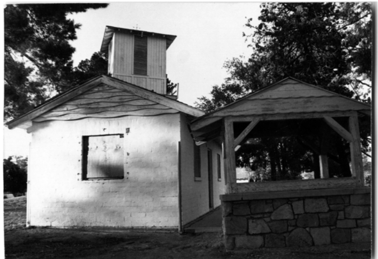
Pump house, well, with water tower in the rear, earl...
