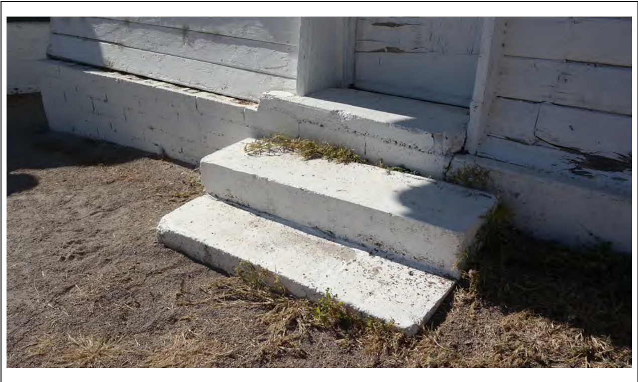
Water Tower – Step detail, east elevation Kautz Environmental Consultants, Inc., November 2024
