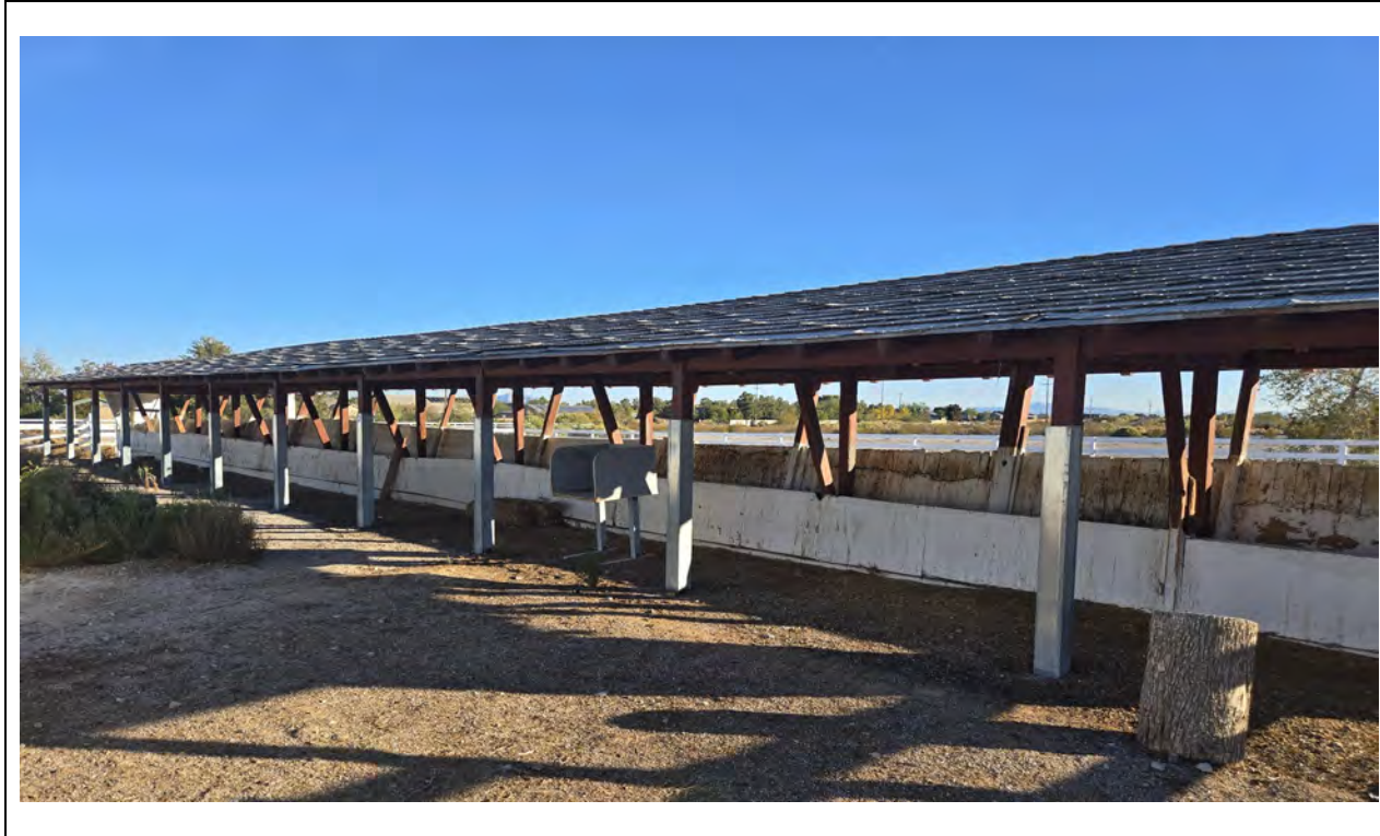
Feed Shelter – North elevation
