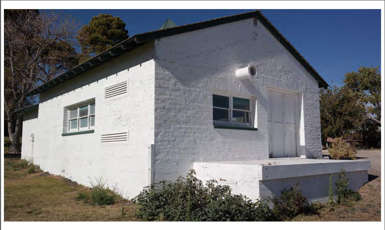
Generator Building – Southeast corner Kautz Environmental Consultants, Inc., November 2024
