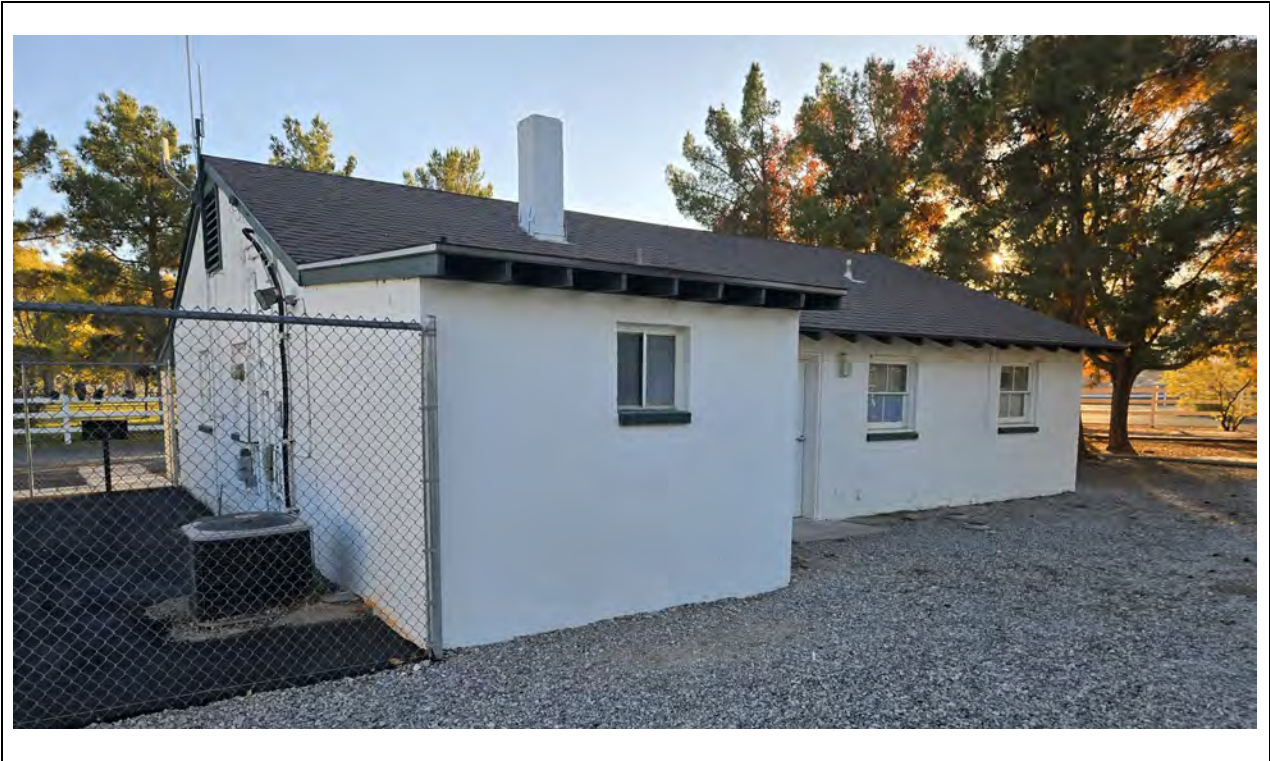
Caretaker's House – Northeast corner Kautz Environmental Consultants, Inc., November 2024
