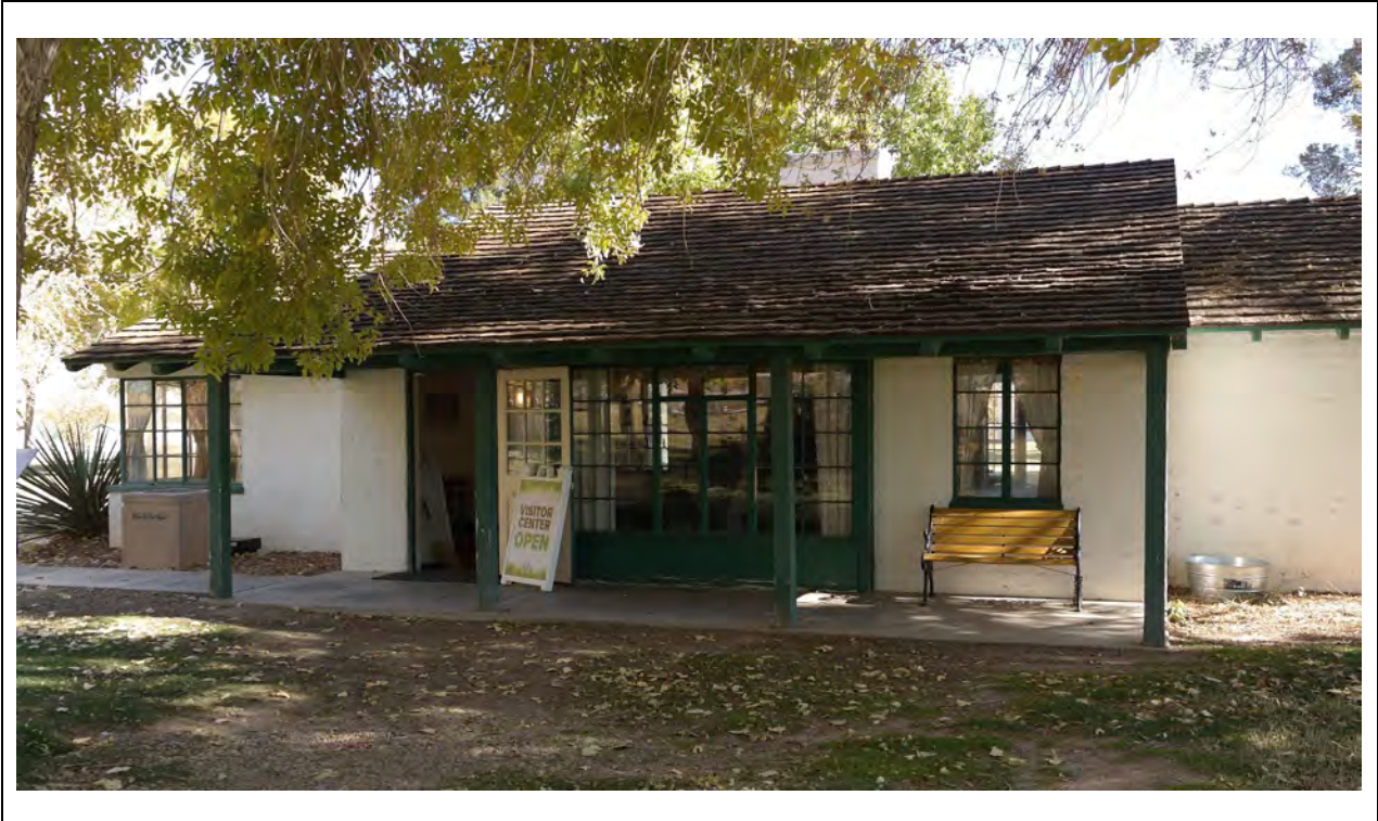
Foreman's House – West entry porch detail Kautz Environmental Consultants, Inc., November 2024
