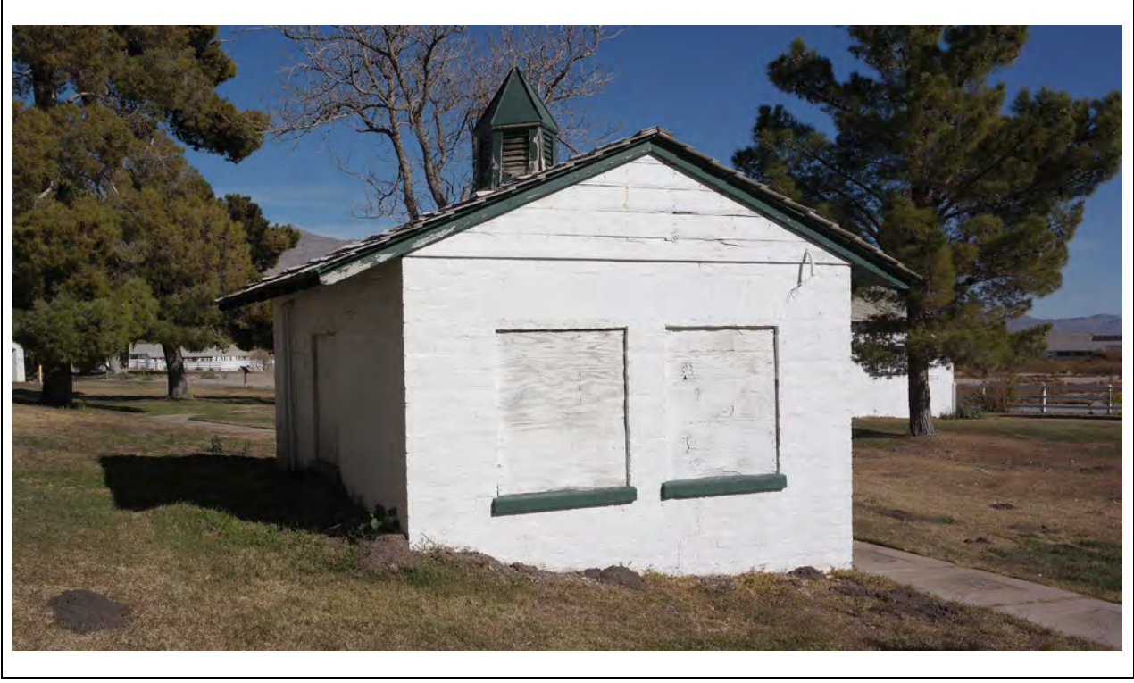
Power House – Southwest elevation and west corner Kautz Environmental Consultants, Inc., November 2024
