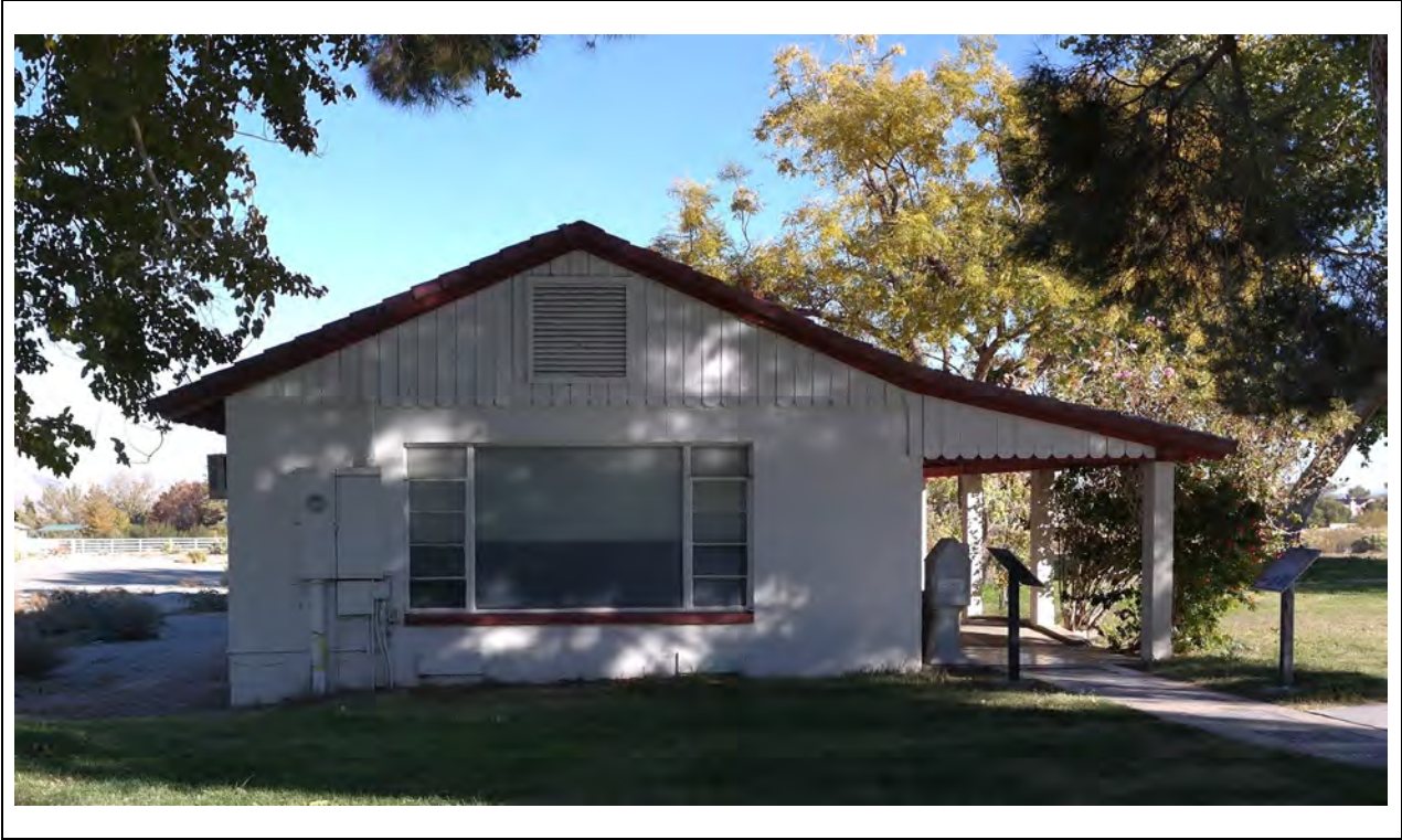
Guest House – West elevation Kautz Environmental Consultants, Inc., November 2024
