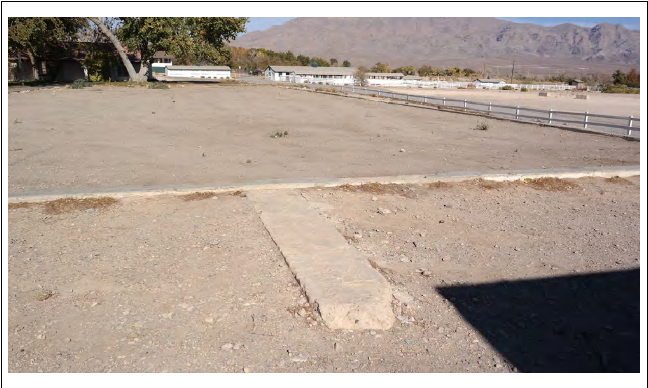
Swimming Pool – Former diving board location Kautz Environmental Consultants, Inc., November 2024
