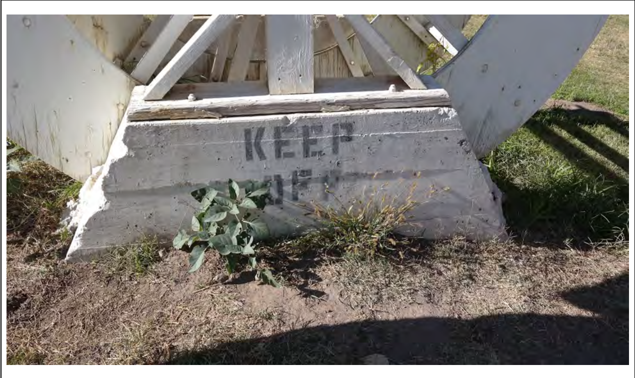
Water Wheel – Base detail Kautz Environmental Consultants, Inc., November 2024
