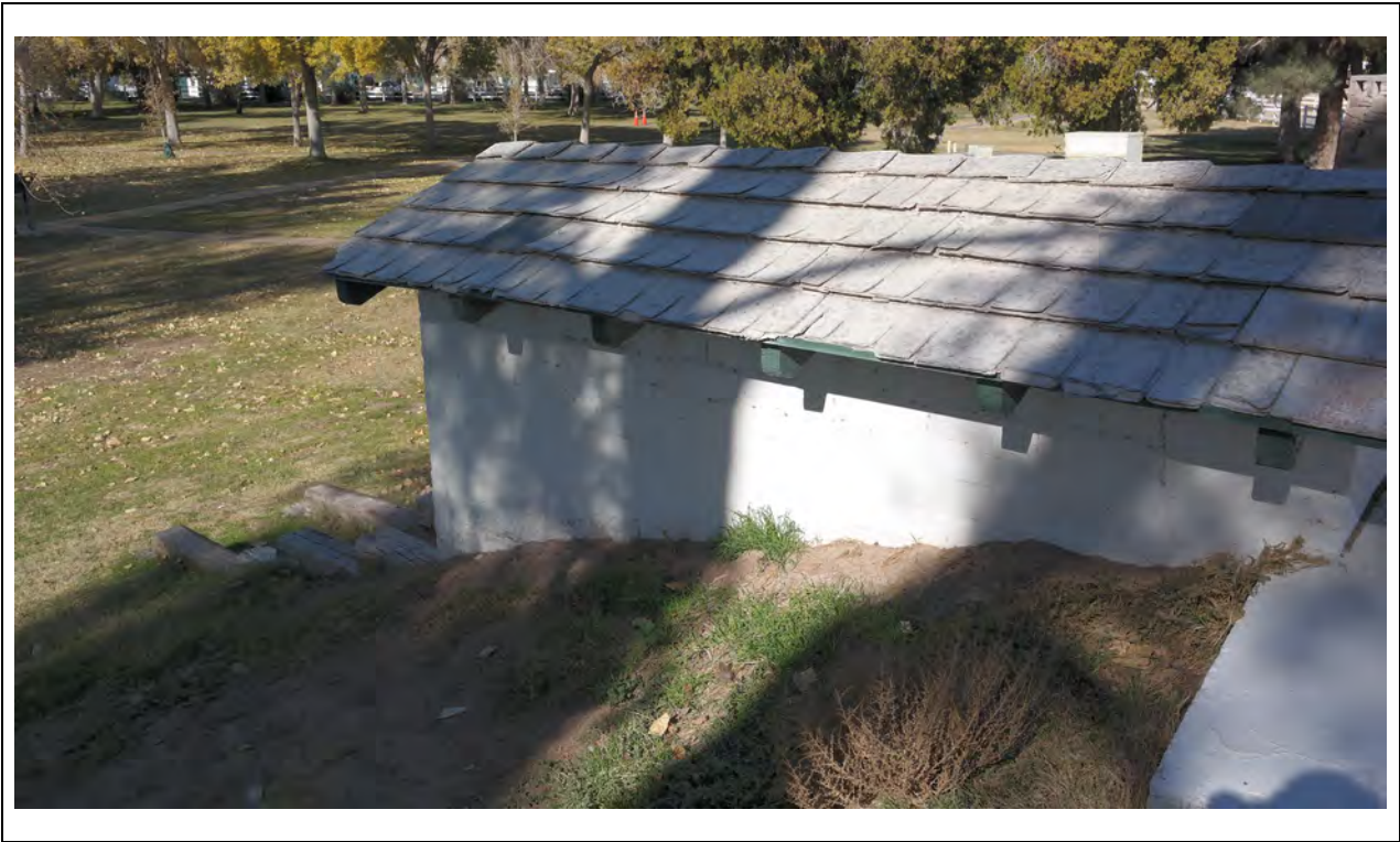
Root Cellar – Southwest elevation detail Kautz Environmental Consultants, Inc., November 2024
