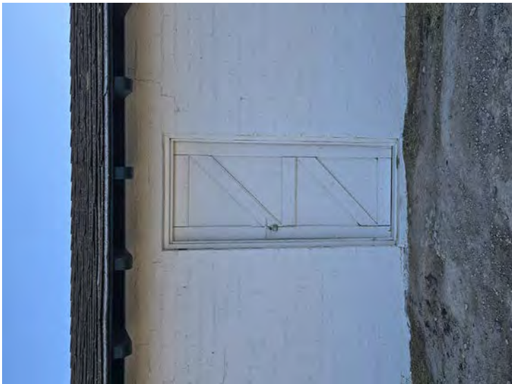
Cow Barn-Dairy - N door detail 11.20.24
