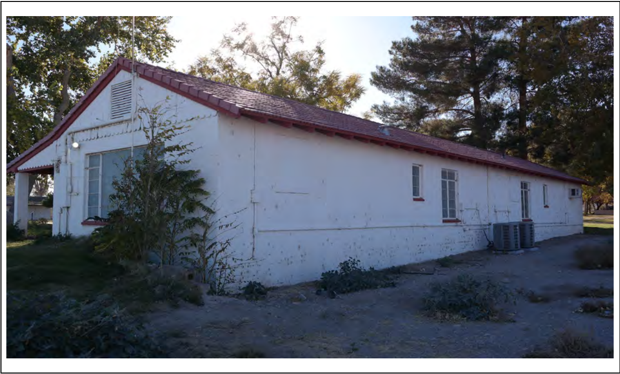
Guest House – North elevation and northeast corner Kautz Environmental Consultants, Inc., November 2024
