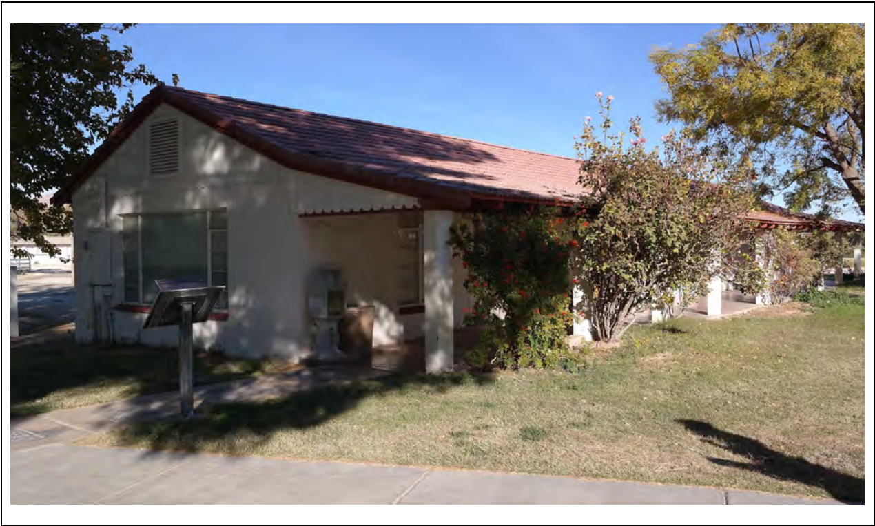
Guest House – Southwest corner Kautz Environmental Consultants, Inc., November 2024
