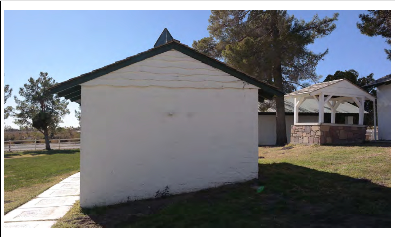
Power House – Northeast elevation Kautz Environmental Consultants, Inc., November 2024
