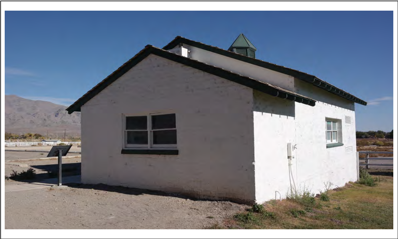
Generator Building – West elevation and southwest corner Kautz Environmental Consultants, Inc., November 2024
