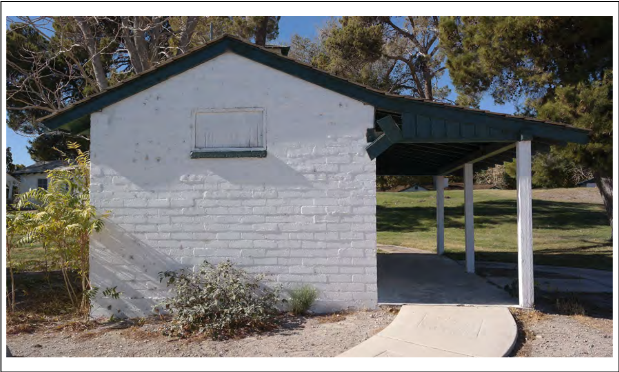
Bath House – East elevation Kautz Environmental Consultants, Inc., November 2024
