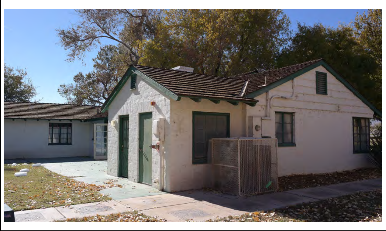
Foreman's House – North elevation and northeast corner Kautz Environmental Consultants, Inc., November 2024
