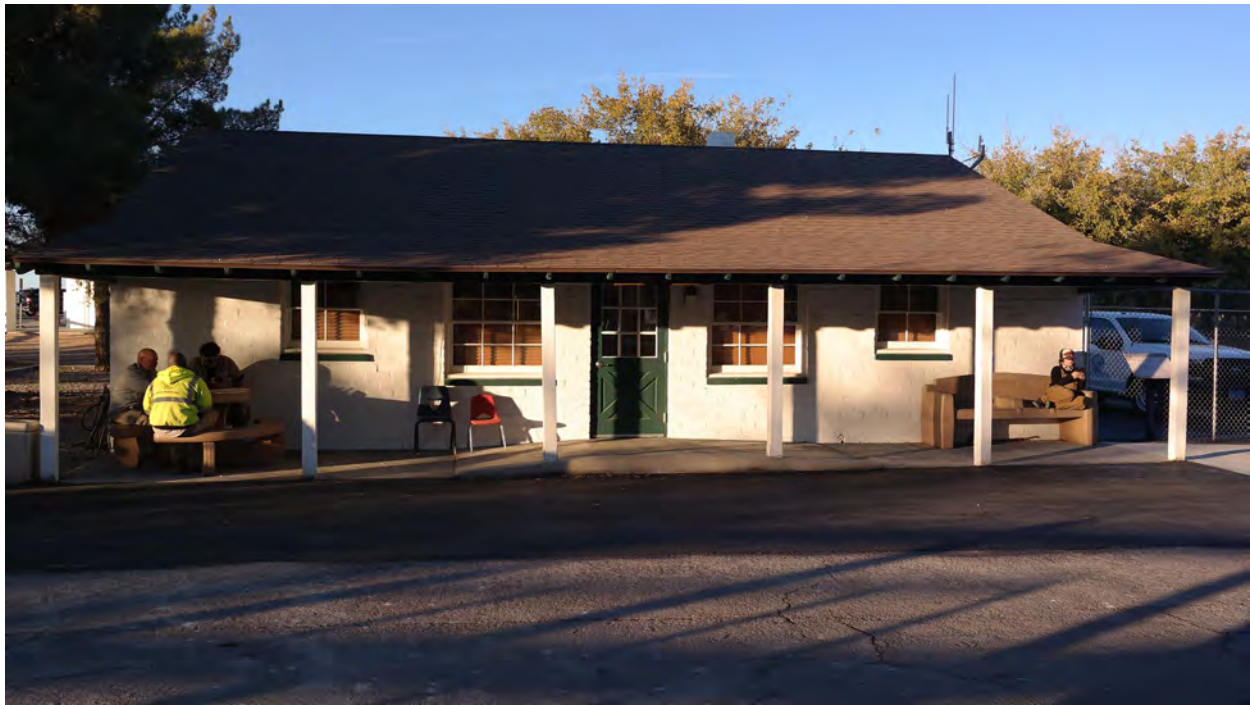
Caretaker's House – South elevation
