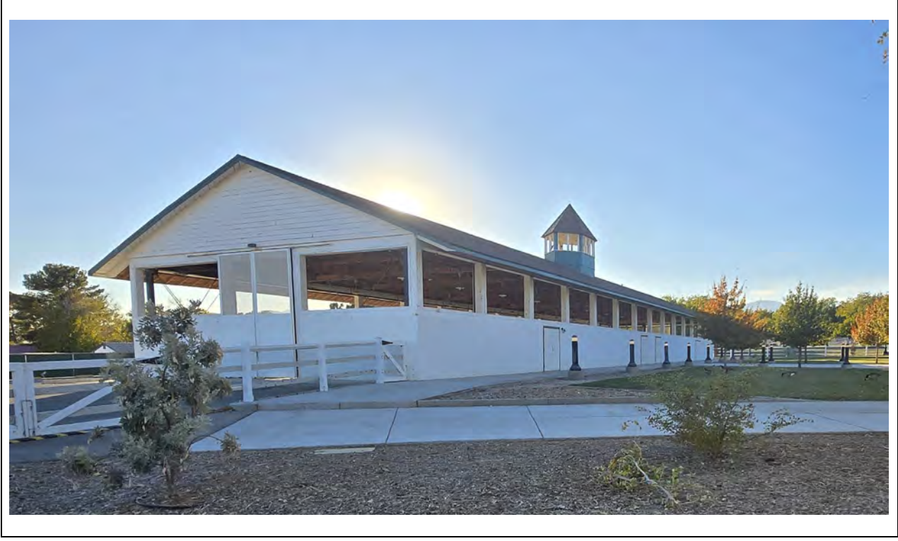
Hay Barn – East elevation, north elevation, and northeast corner Kautz Environmental Consultants, Inc., November 2024
