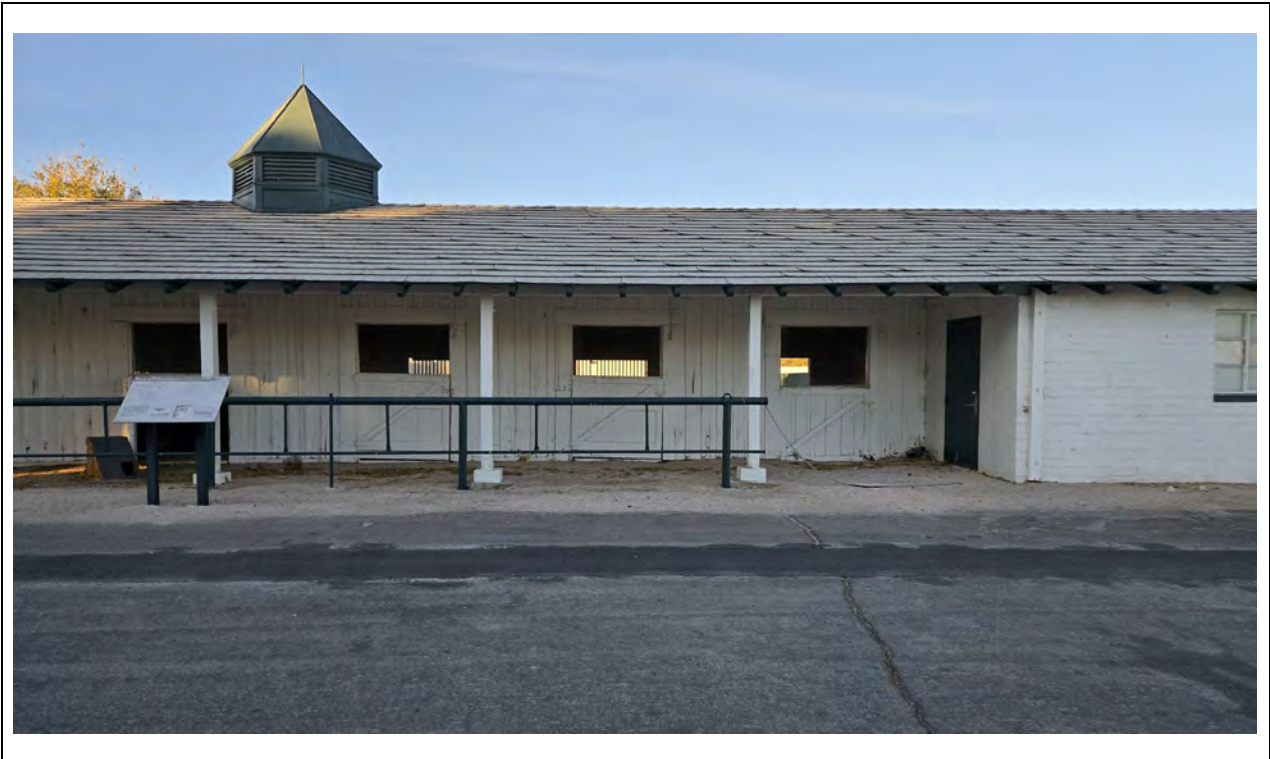
Office/Stables – South elevation, east/center Kautz Environmental Consultants, Inc., November 2024
