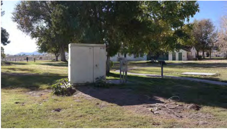
Overview - Near Water Wheel looking SW 11.20.24
