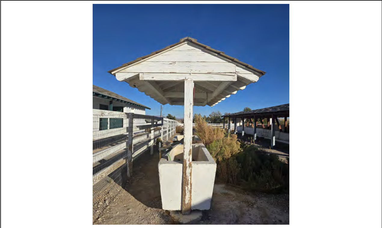
Covered Trough – West elevation Kautz Environmental Consultants, Inc., November 2024
