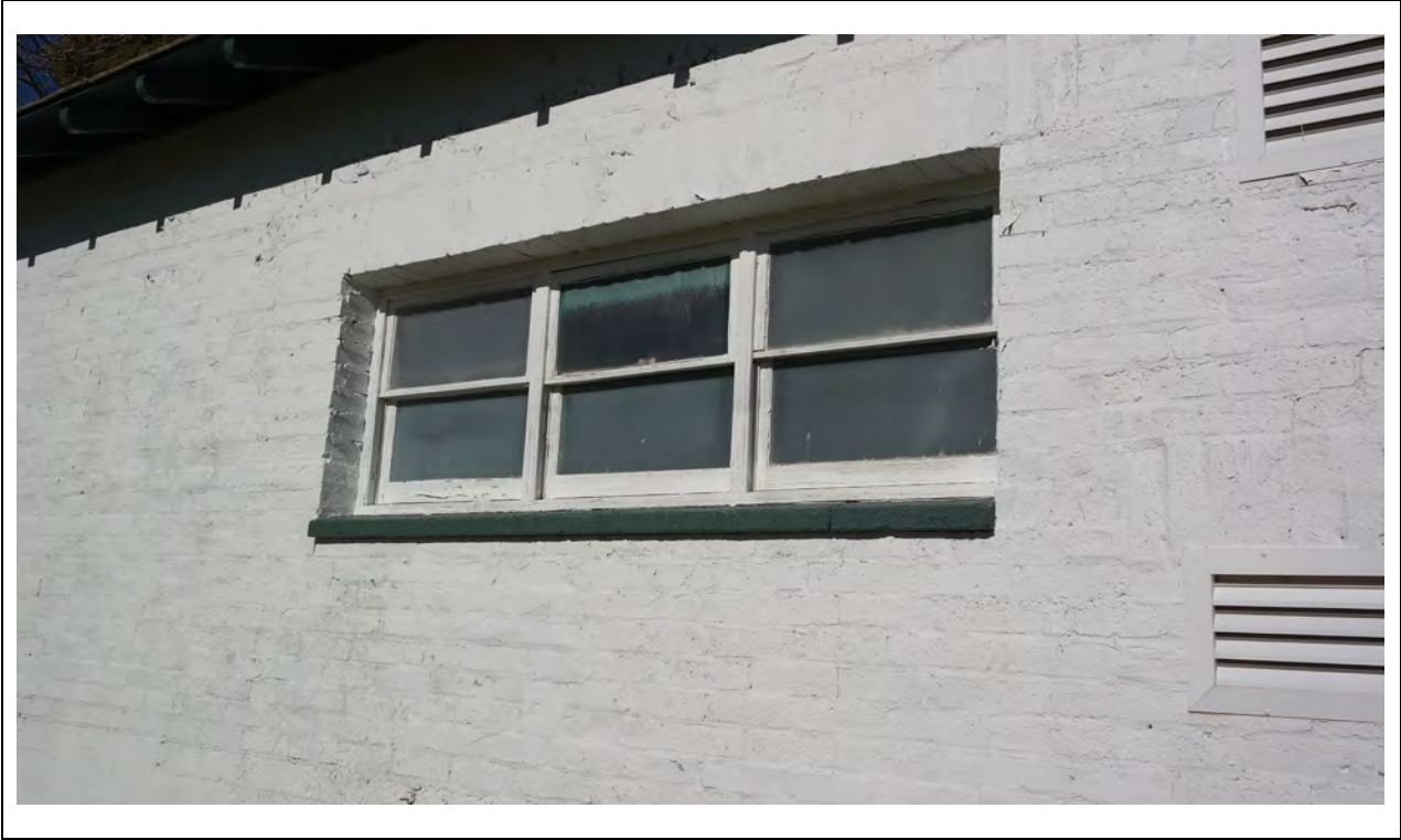
Generator Building – South elevation window detail Kautz Environmental Consultants, Inc., November 2024
