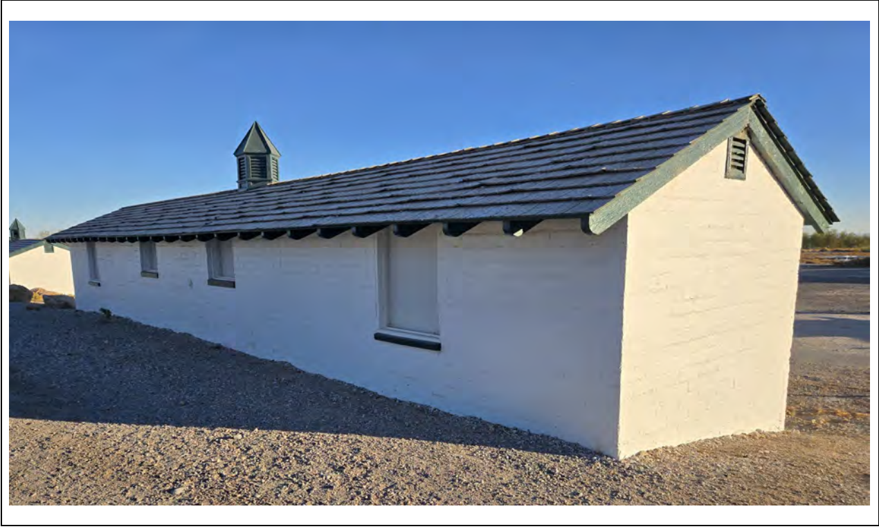
East Chicken Coop – Northwest corner Kautz Environmental Consultants, Inc., November 2024
