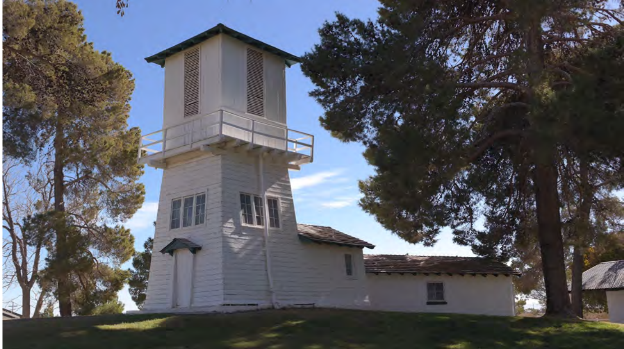
Water Tower – Northwest corner
