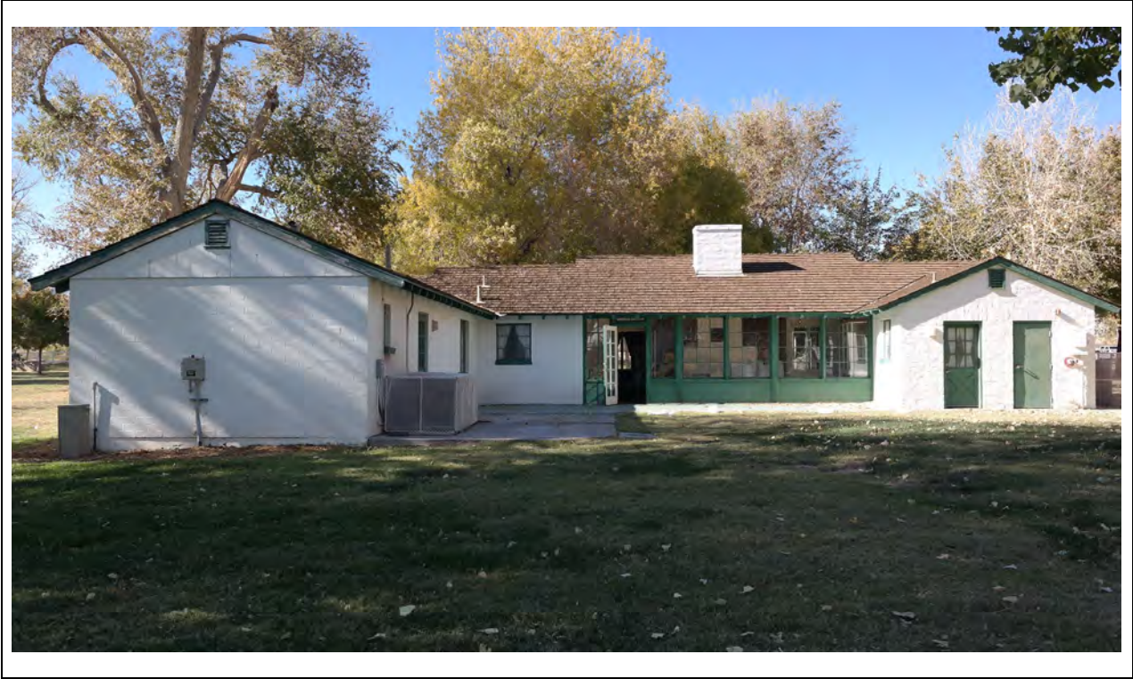
Foreman's House – East elevation Kautz Environmental Consultants, Inc., November 2024
