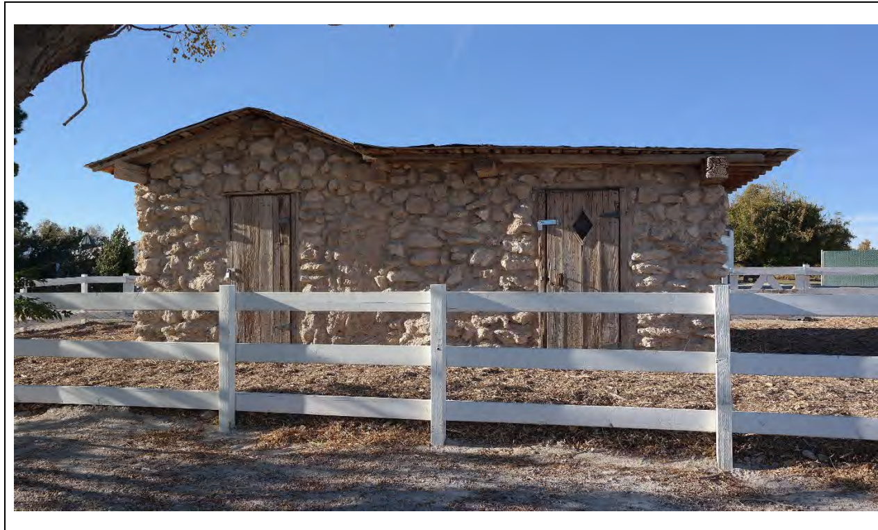
Adobe Hut – Southeast elevation
