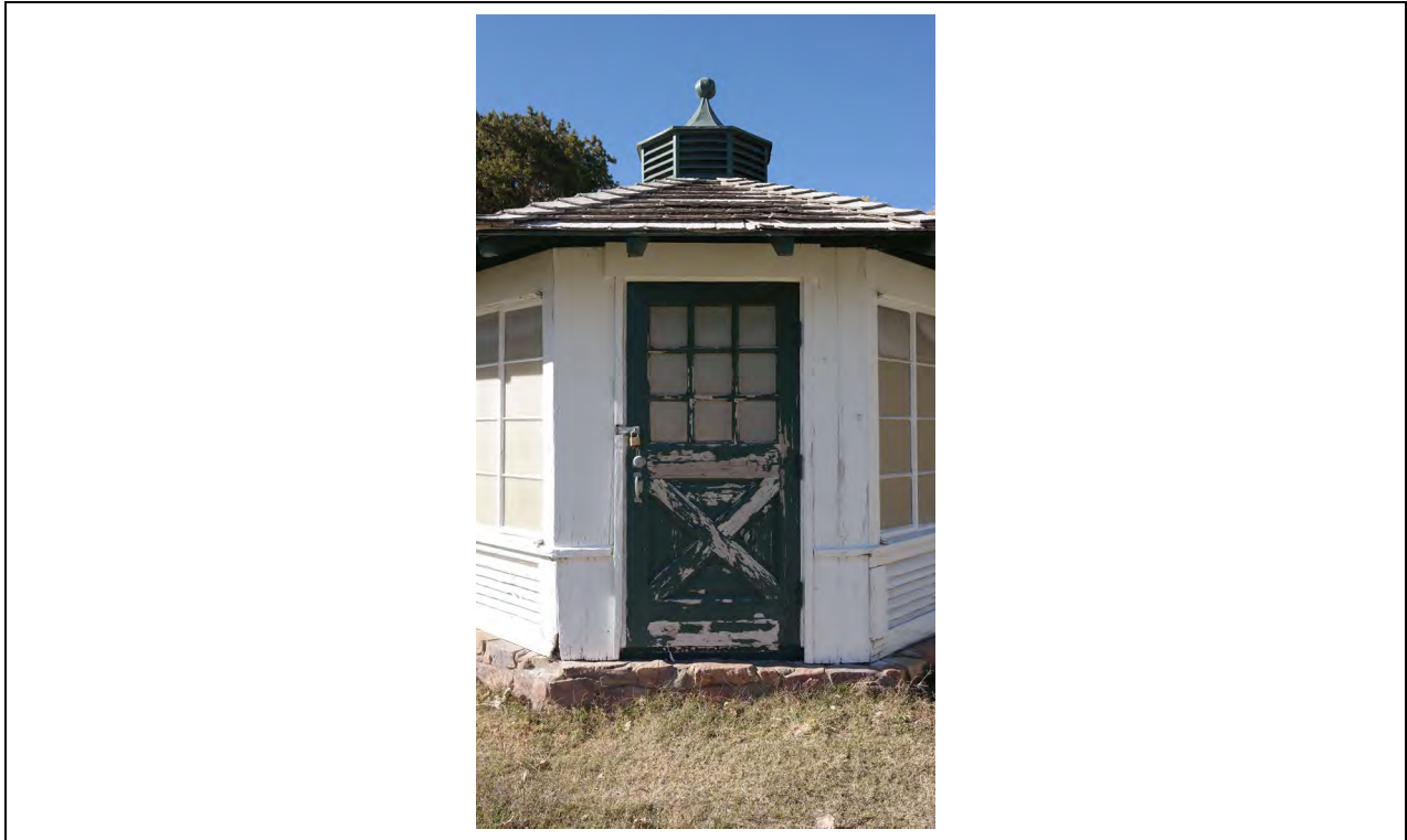
Pump House – Door detail
