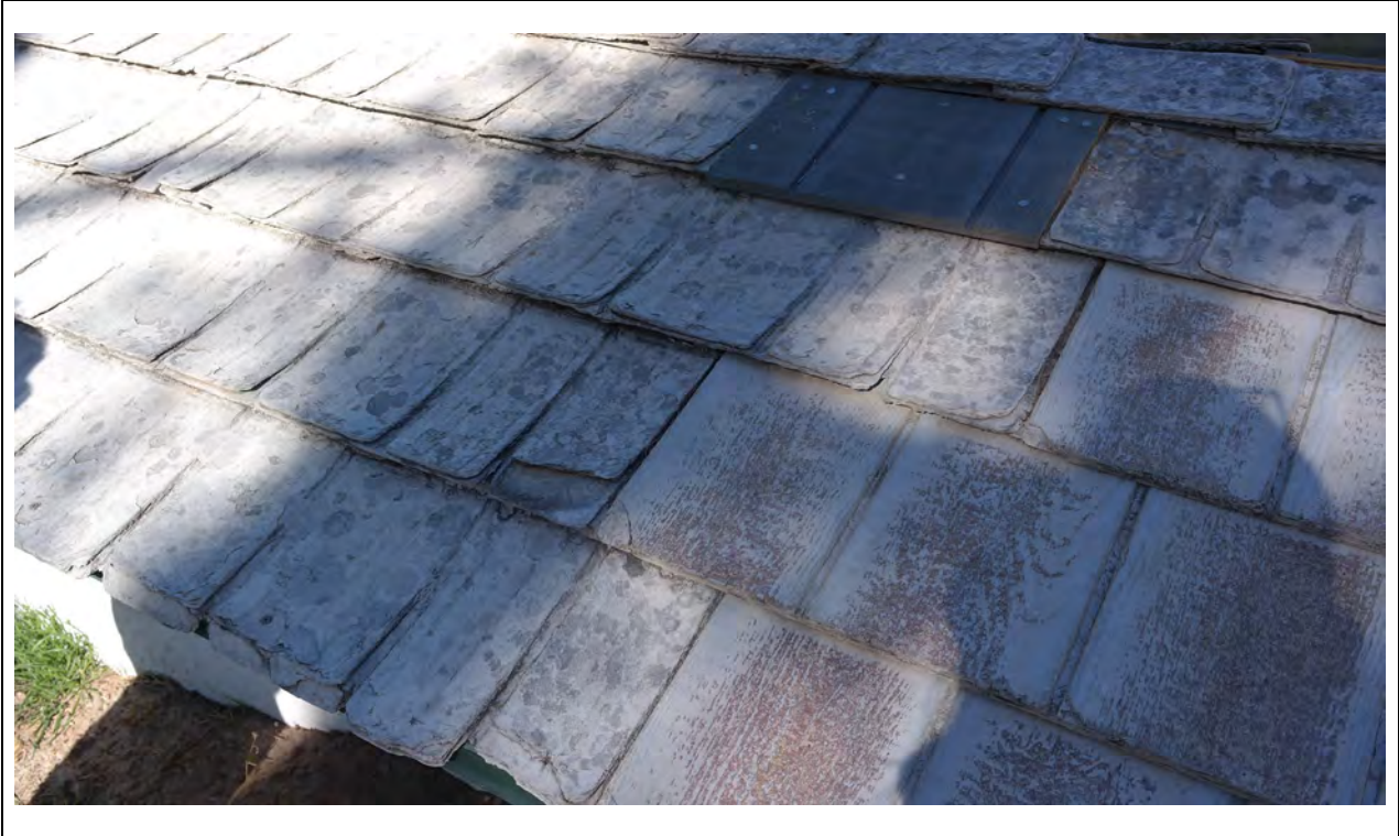
Root Cellar – Roof detail Kautz Environmental Consultants, Inc., November 2024
