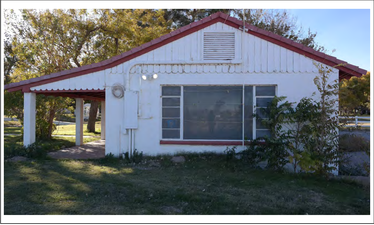
Guest House – East elevation Kautz Environmental Consultants, Inc., November 2024
