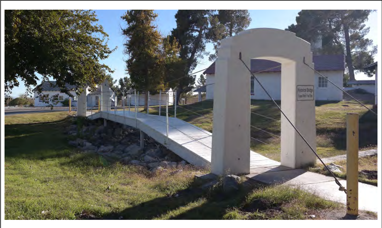
Suspension Bridge – Northeast corner Kautz Environmental Consultants, Inc., November 2024
