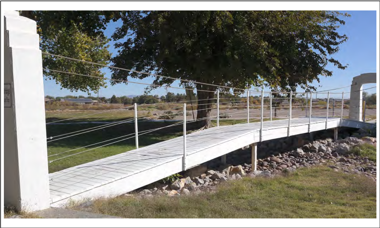
Suspension Bridge – Deck detail Kautz Environmental Consultants, Inc., November 2024
