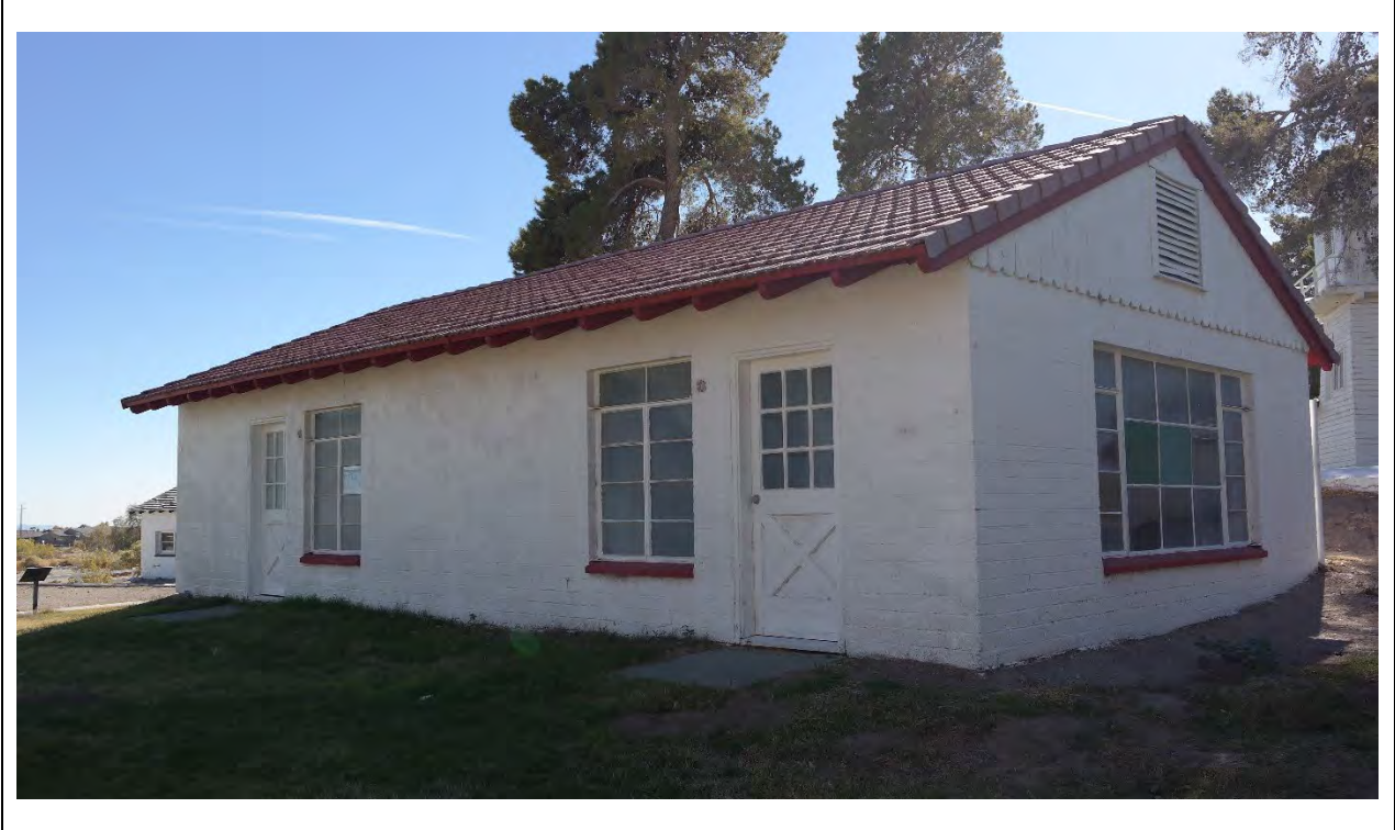
Duplex – Northeast elevation and north corner Kautz Environmental Consultants, Inc., November 2024
