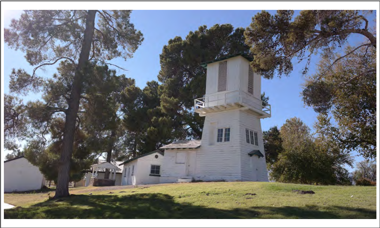
Water Tower – Northeast corner overview Kautz Environmental Consultants, Inc., November 2024
