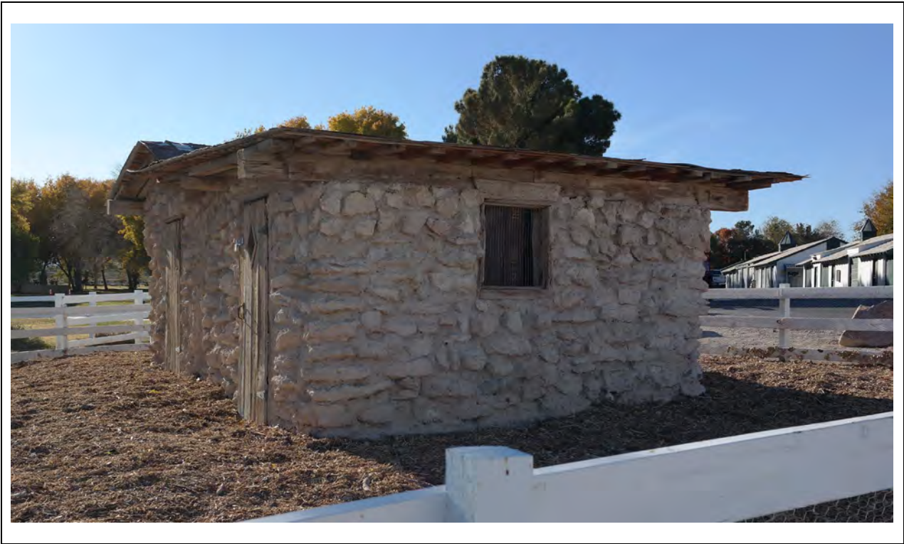
Adobe Hut – Northeast elevation and east corner Kautz Environmental Consultants, Inc., November 2024
