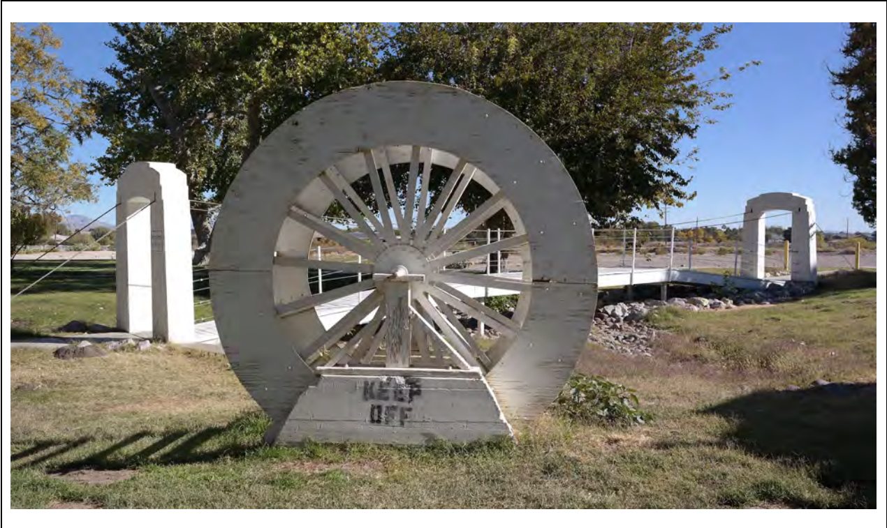
Water Wheel – West elevation Kautz Environmental Consultants, Inc., November 2024
