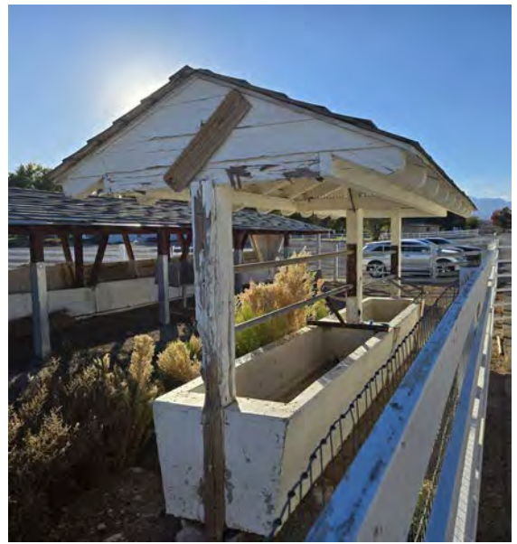
Covered Trough - NE corner 11.20.24
