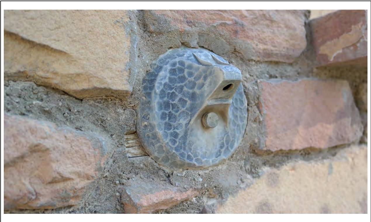
Outdoor Fireplace – Hardware detail Kautz Environmental Consultants, Inc., November 2024
