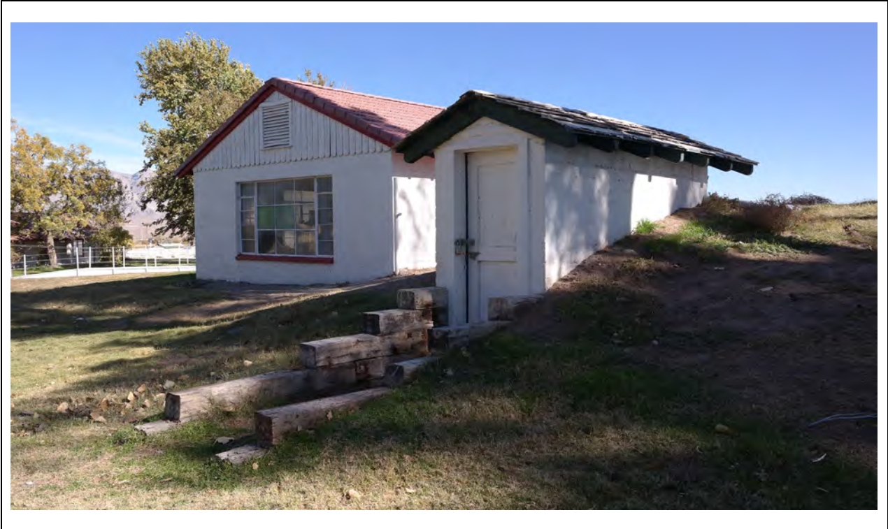
Root Cellar – West corner Kautz Environmental Consultants, Inc., November 2024
