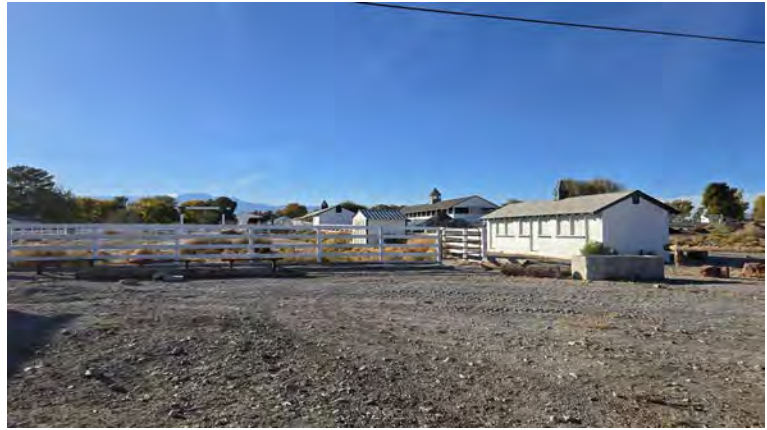
Overview - Near Orchard looking WNW 11.20.24
