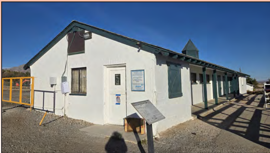
Figure 5.23 Cow Barn/Dairy Building (#23)
