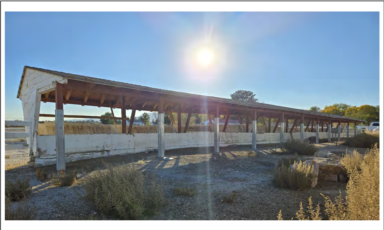
Feed Shelter – North elevation and northeast corner Kautz Environmental Consultants, Inc., November 2024
