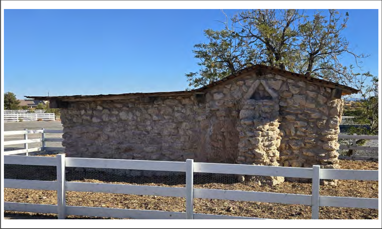
Adobe Hut – Northwest elevation Kautz Environmental Consultants, Inc., November 2024
