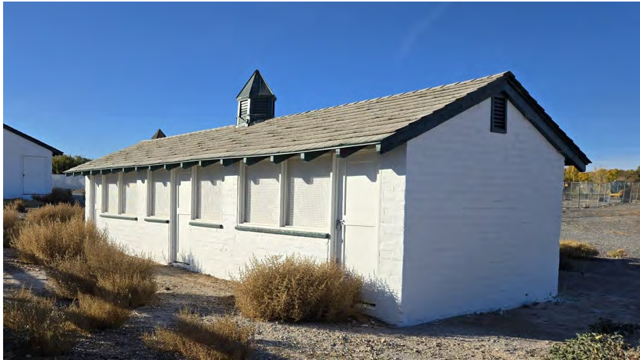
West Pig Housing – Southeast corner Kautz Environmental Consultants, Inc., November 2024
