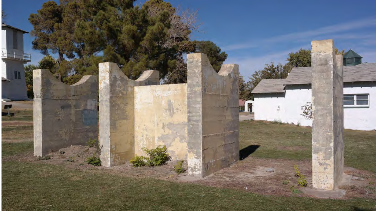
Diesel Oil Support – South elevation
