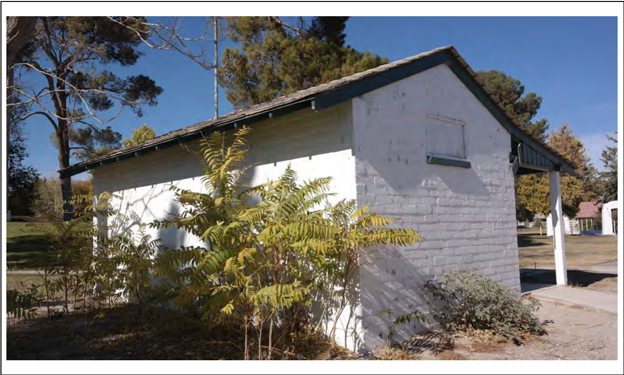
Bath House – Southeast corner Kautz Environmental Consultants, Inc., November 2024
