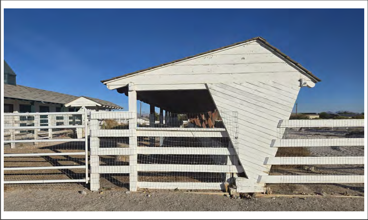
Feed Shelter – West elevation Kautz Environmental Consultants, Inc., November 2024
