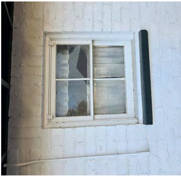
Caretaker's House - Window detail 11.20.24
