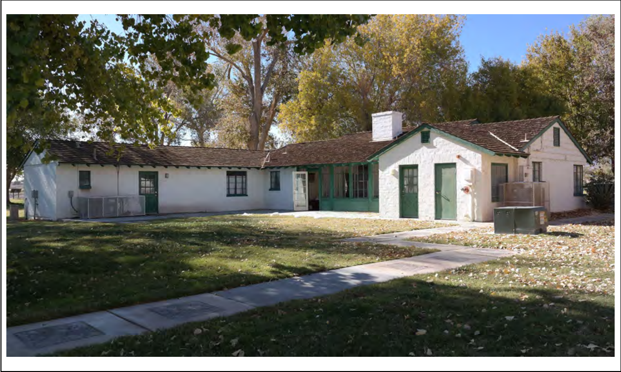
Foreman's House – East elevation and northeast corner Kautz Environmental Consultants, Inc., November 2024
