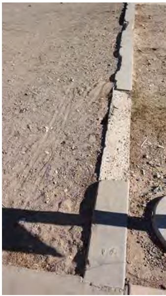
Swimming Pool - Coping detail 11.20.24
