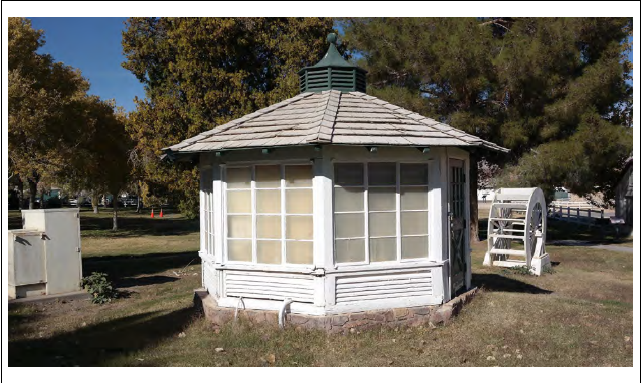
Pump House – South elevation Kautz Environmental Consultants, Inc., November 2024
