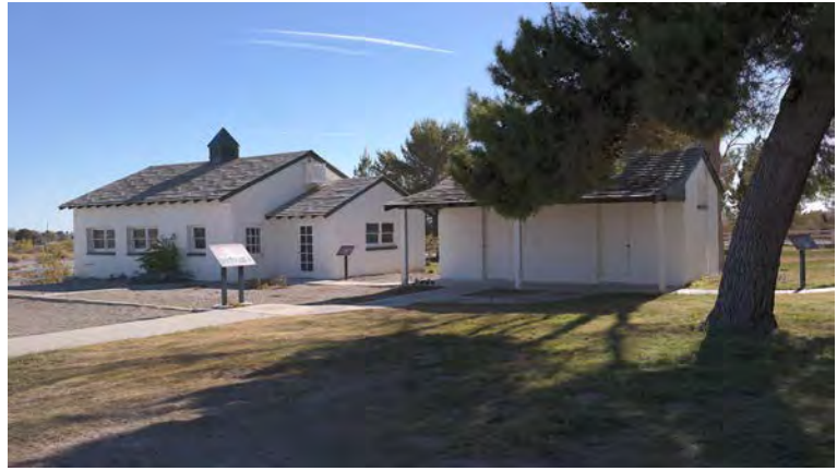
Overview - Near Duplex looking SSE 11.20.24
