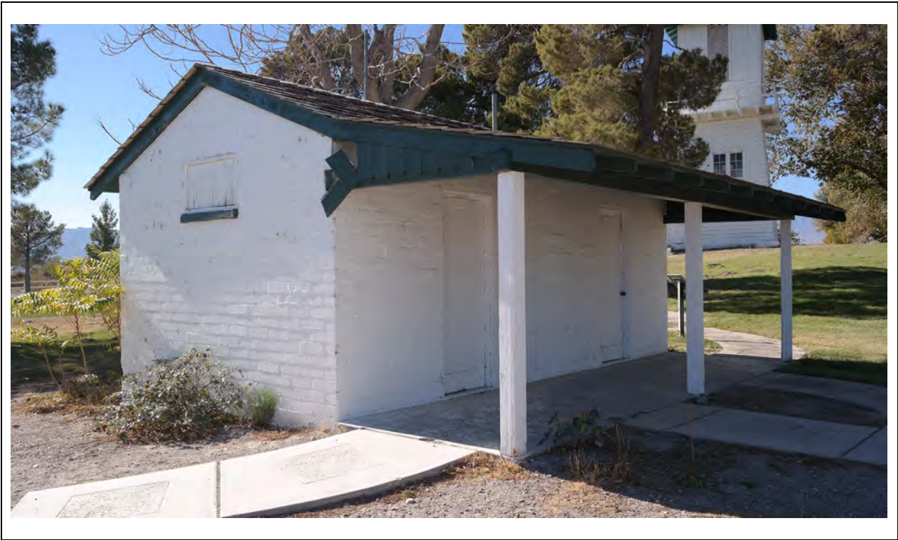
Bath House – Northeast corner Kautz Environmental Consultants, Inc., November 2024
