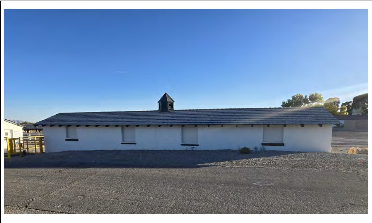
East Chicken Coop – North elevation Kautz Environmental Consultants, Inc., November 2024
