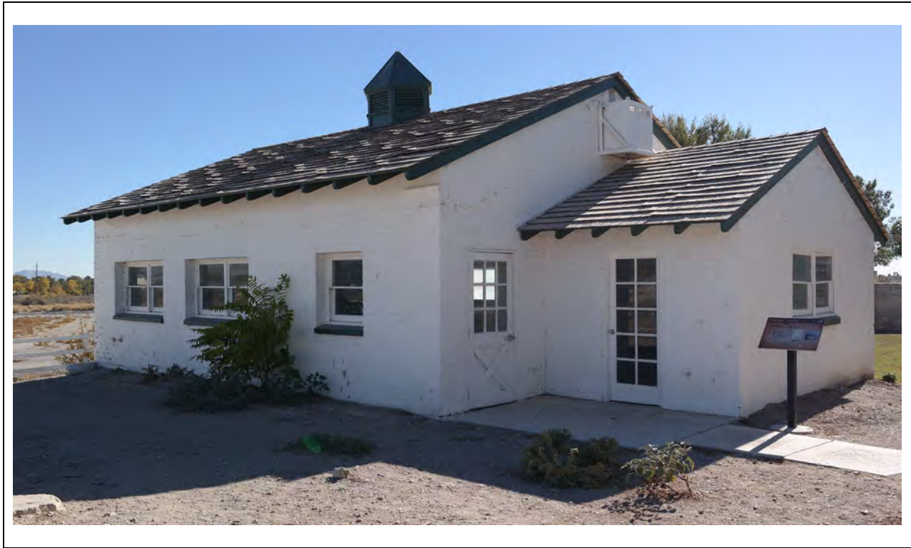
Generator Building – North elevation and northwest corner
