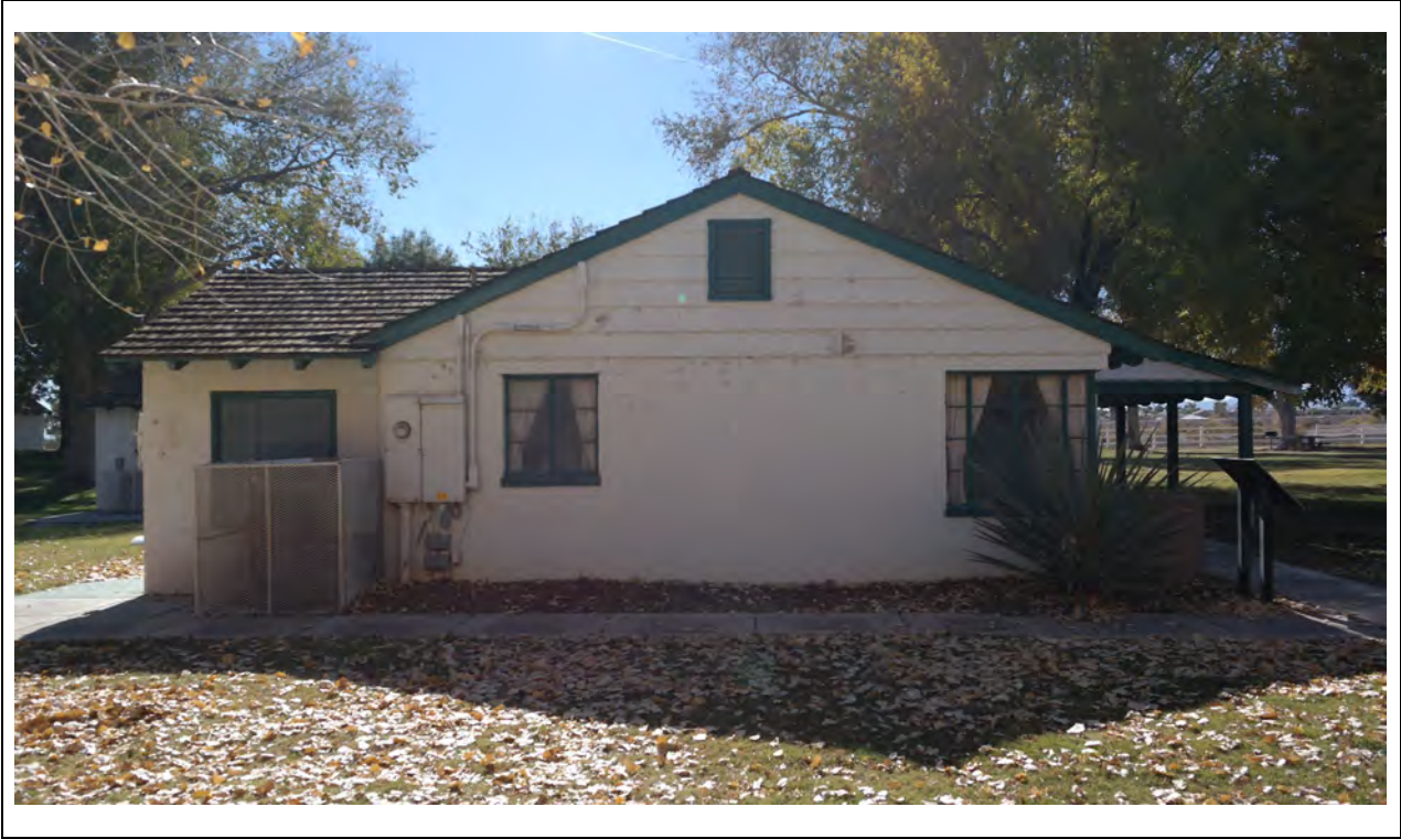
Foreman's House – North elevation Kautz Environmental Consultants, Inc., November 2024
