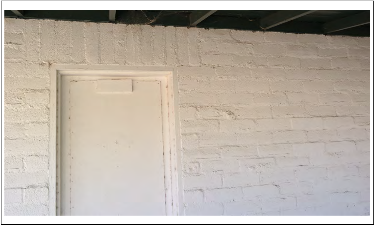
Bath House – Lintel detail
