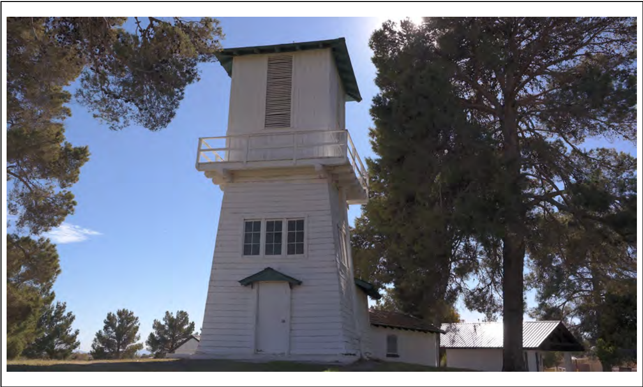
Water Tower – North elevation Kautz Environmental Consultants, Inc., November 2024
