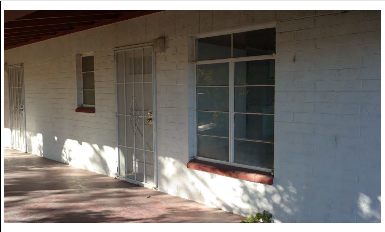
Guest House – South elevation door and window detail Kautz Environmental Consultants, Inc., November 2024
