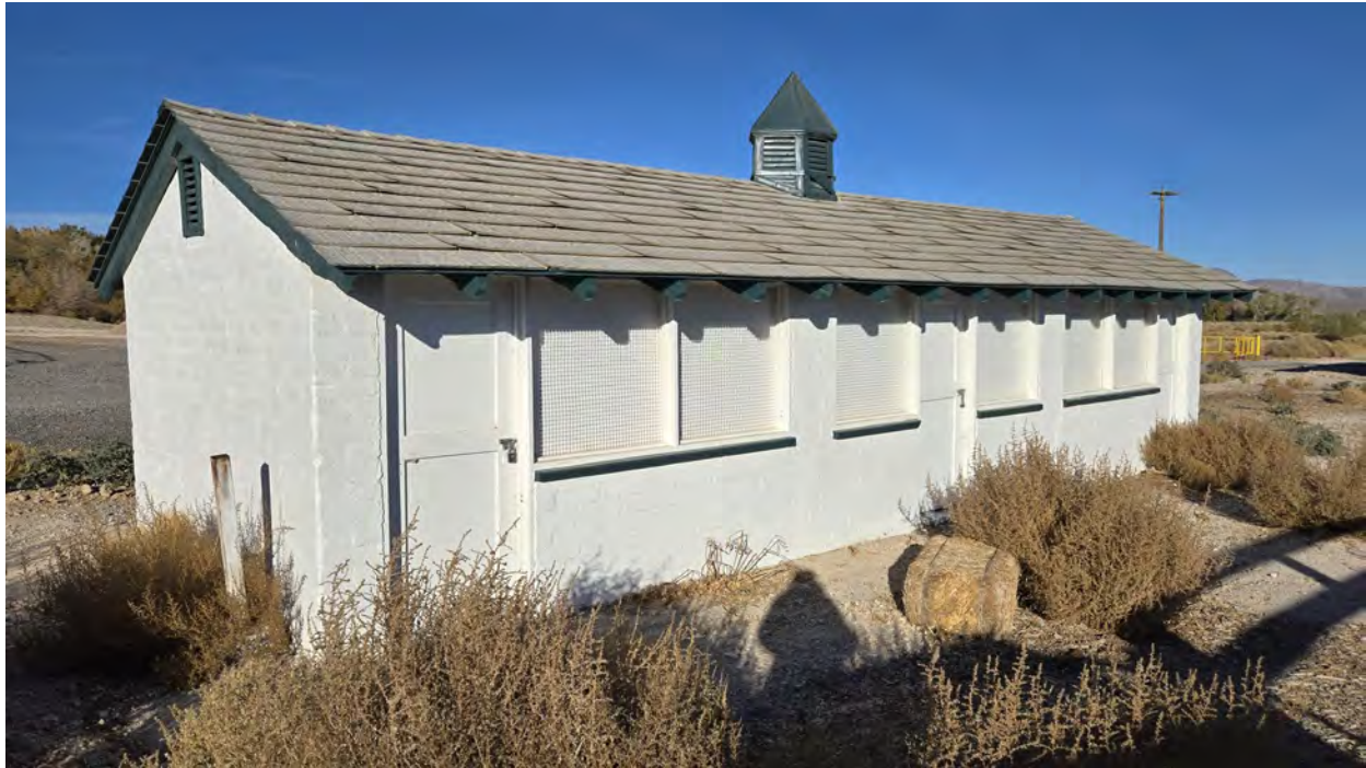
West Pig Housing – South elevation and southwest corner Kautz Environmental Consultants, Inc., November 2024
