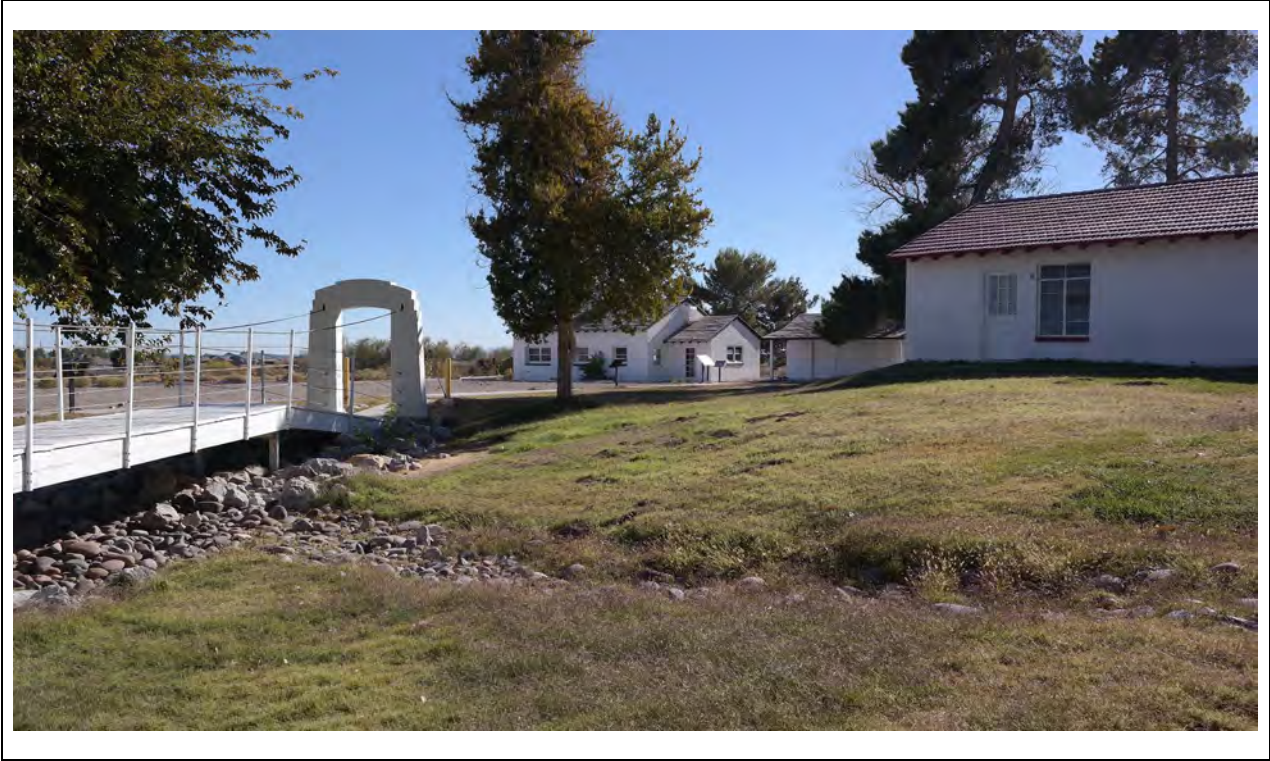
Suspension Bridge – Channel detail Kautz Environmental Consultants, Inc., November 2024
