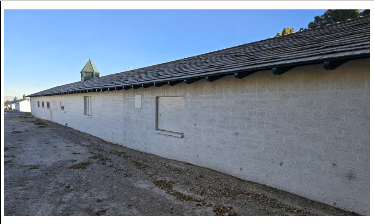
Office/Stables – North elevation, east end and center Kautz Environmental Consultants, Inc., November 2024
