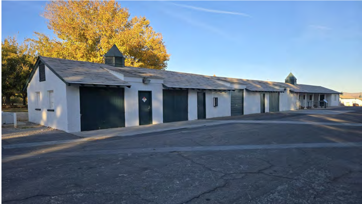
Office/Stables – South elevation and southwest corner
