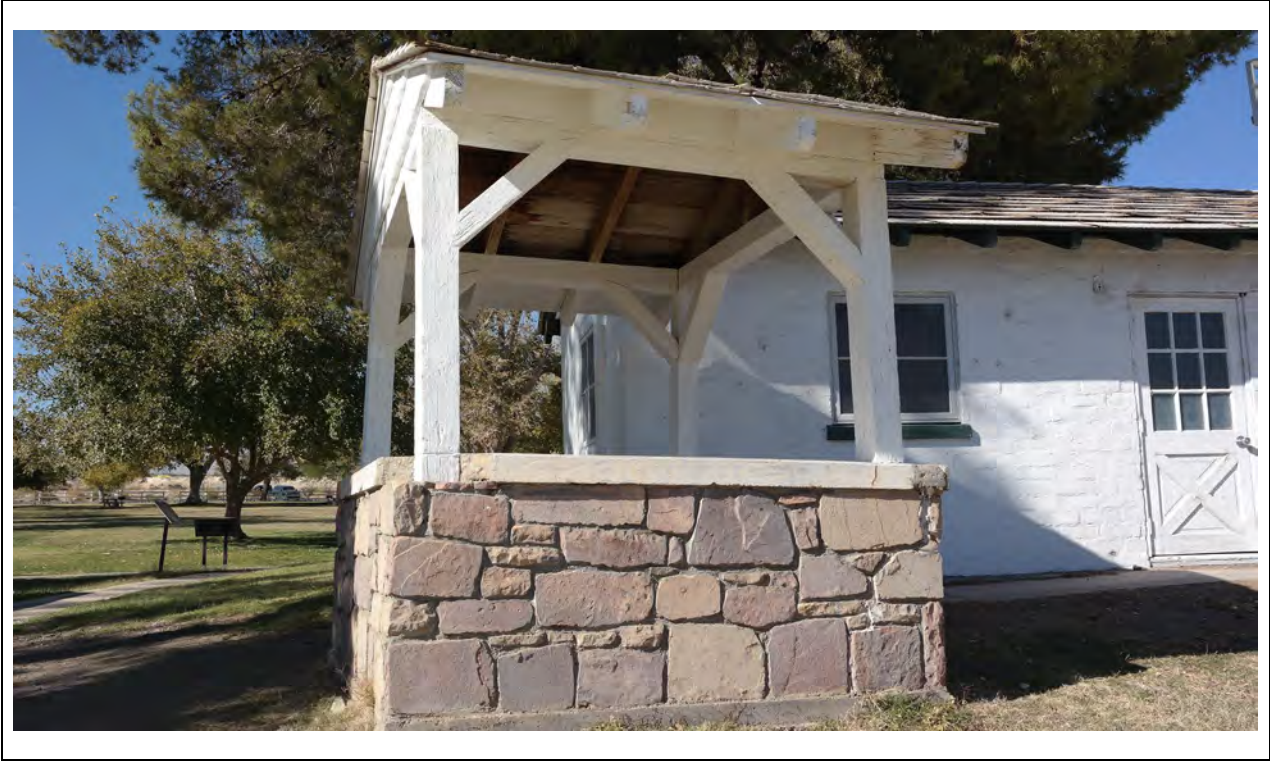
Well – East elevation Kautz Environmental Consultants, Inc., November 2024
