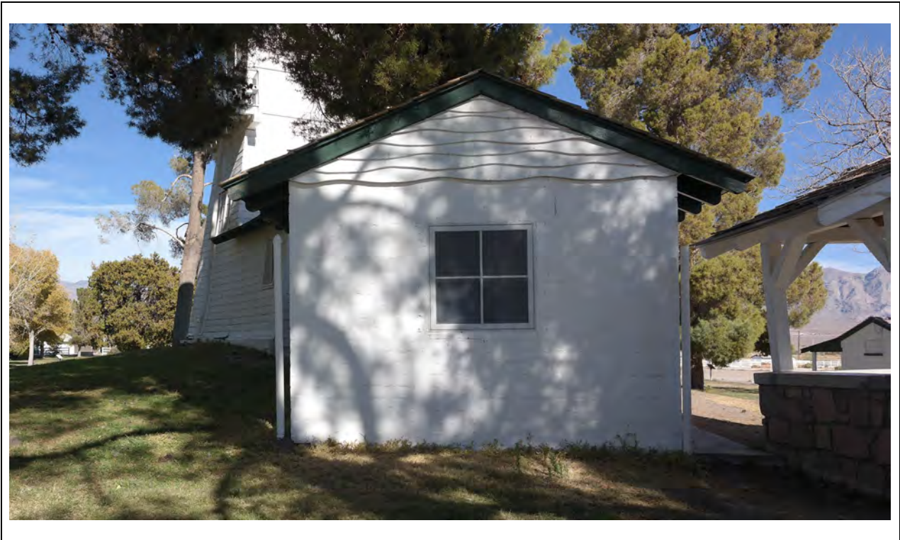
Spring House – Southwest elevation Kautz Environmental Consultants, Inc., November 2024
