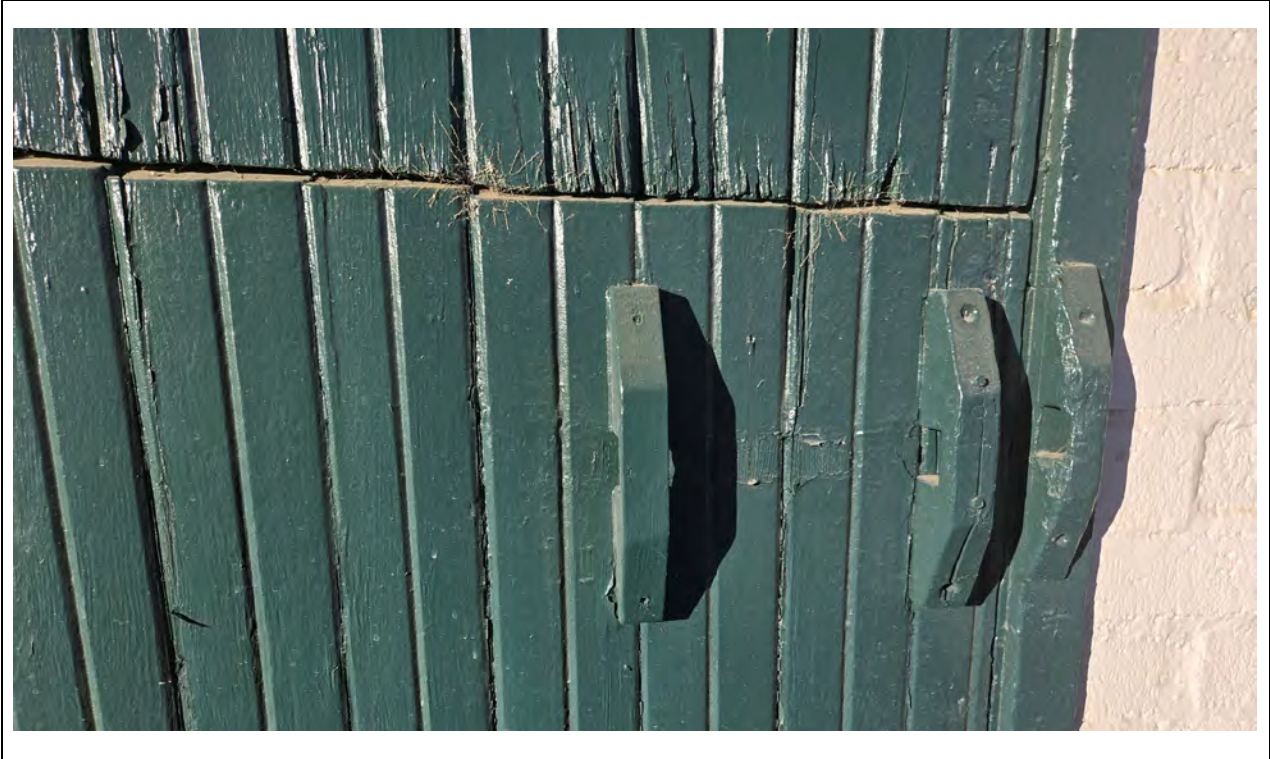
Cow Barn / Dairy Building – Door detail, south elevation Kautz Environmental Consultants, Inc., November 2024
