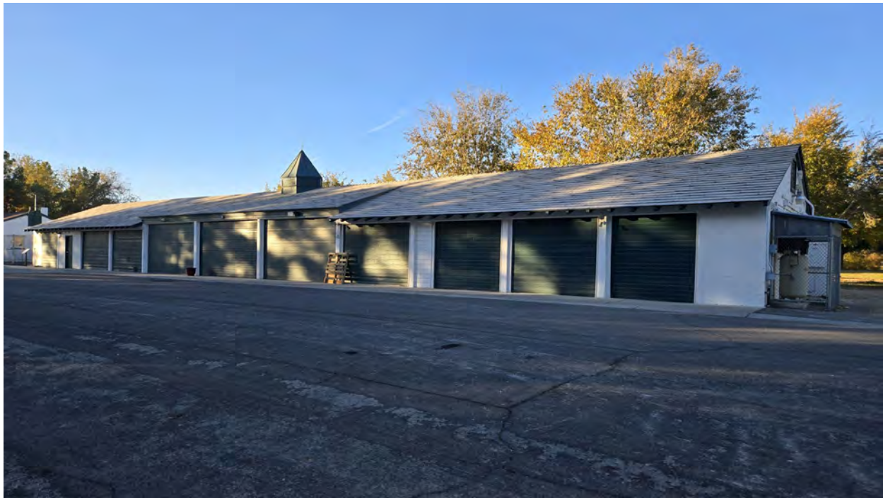
Machine Building/Firehouse – South elevation Kautz Environmental Consultants, Inc., November 2024
