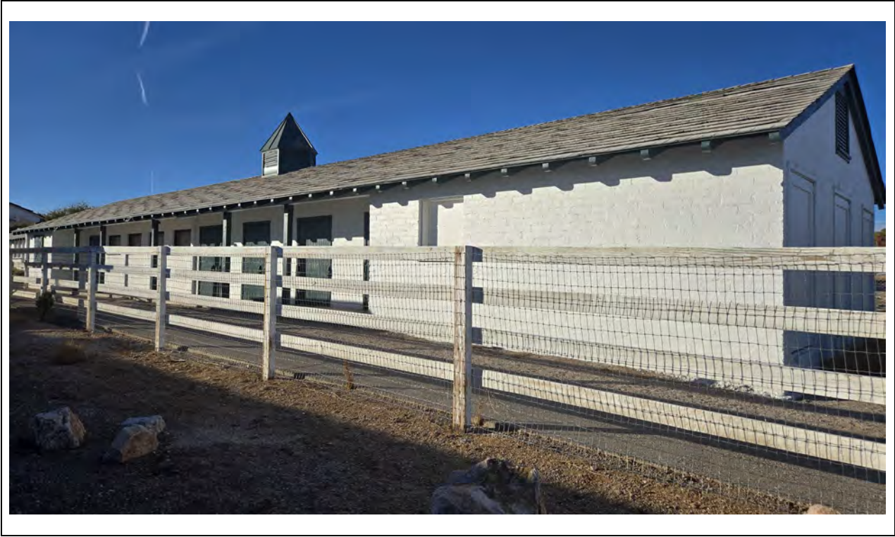
Cow Barn / Dairy Building – South elevation, east end Kautz Environmental Consultants, Inc., November 2024
