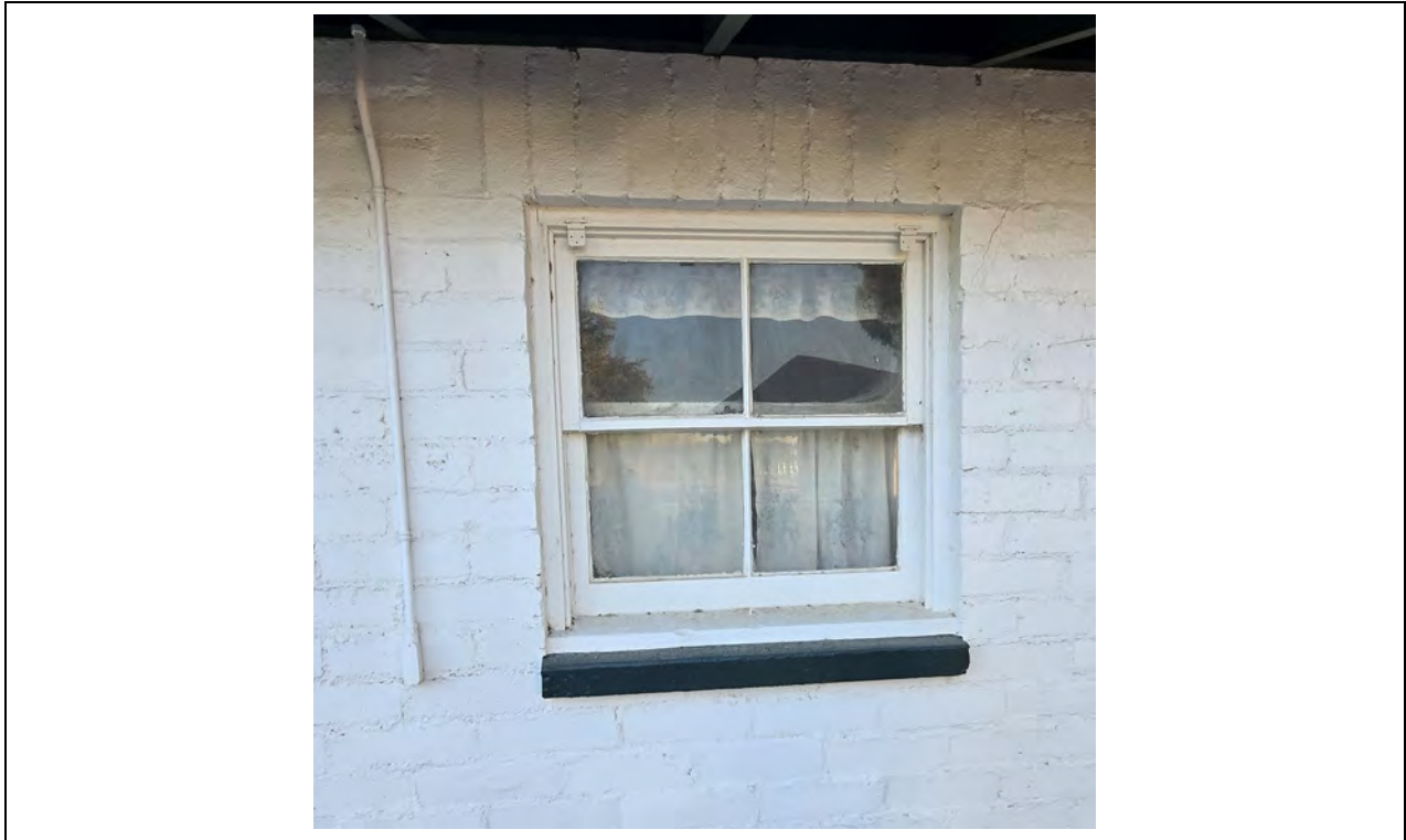
Caretaker's House – Window and lintel detail
