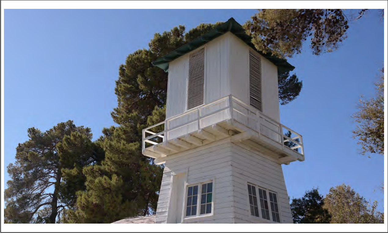
Water Tower – Tower detail, northeast corner Kautz Environmental Consultants, Inc., November 2024
