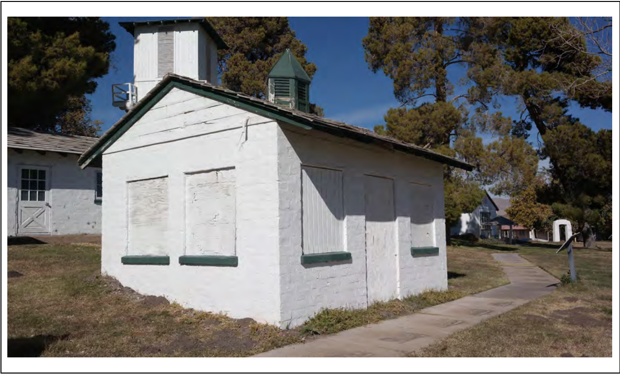
Power House – South corner Kautz Environmental Consultants, Inc., November 2024
