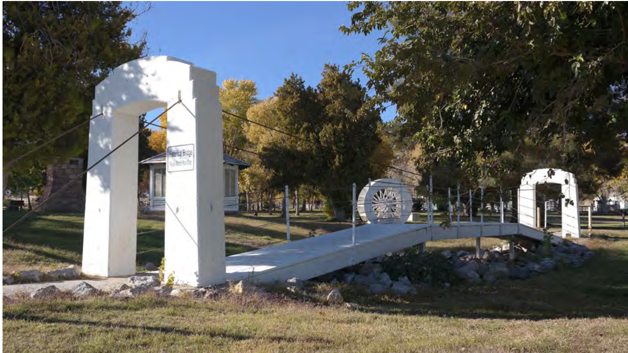
Suspension Bridge – Southeast corner
