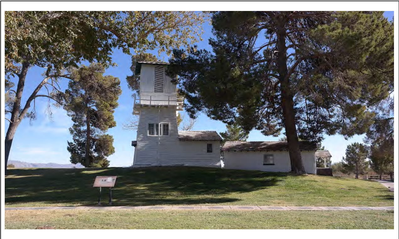
Water Tower – West elevation overview Kautz Environmental Consultants, Inc., November 2024
