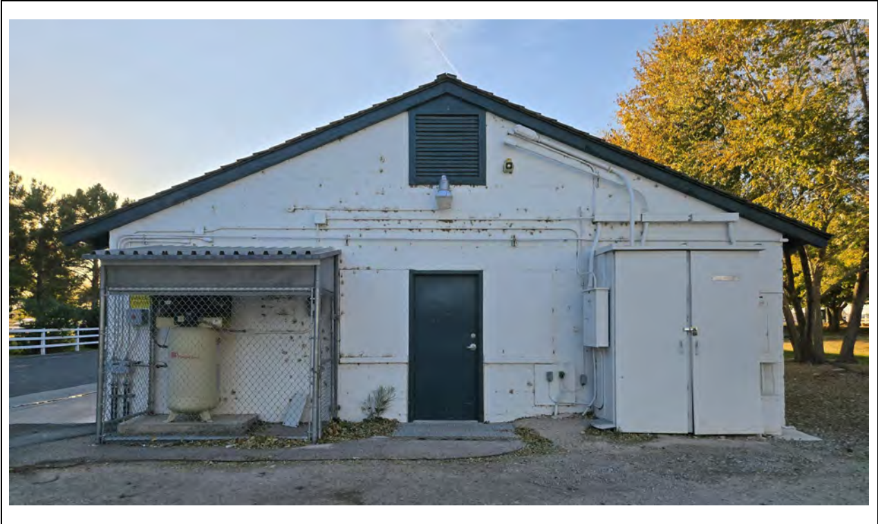
Machine Building/Firehouse – East elevation Kautz Environmental Consultants, Inc., November 2024
