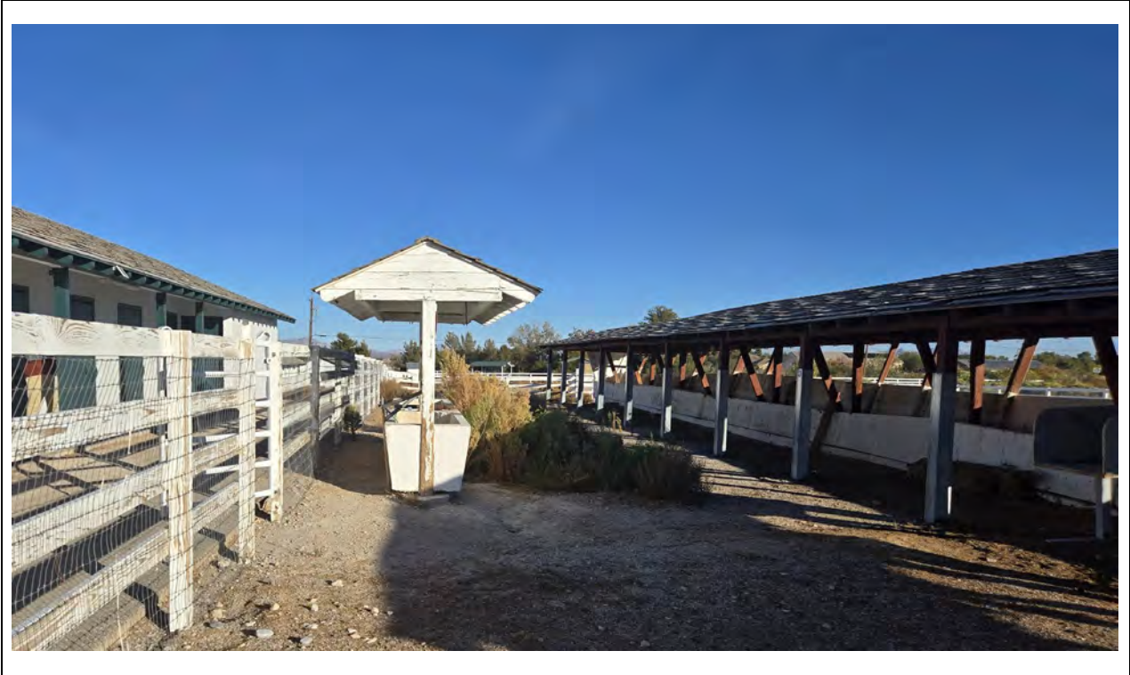
Covered Trough – West elevation overview with Feed Shelter on right Kautz Environmental Consultants, Inc., November 2024
