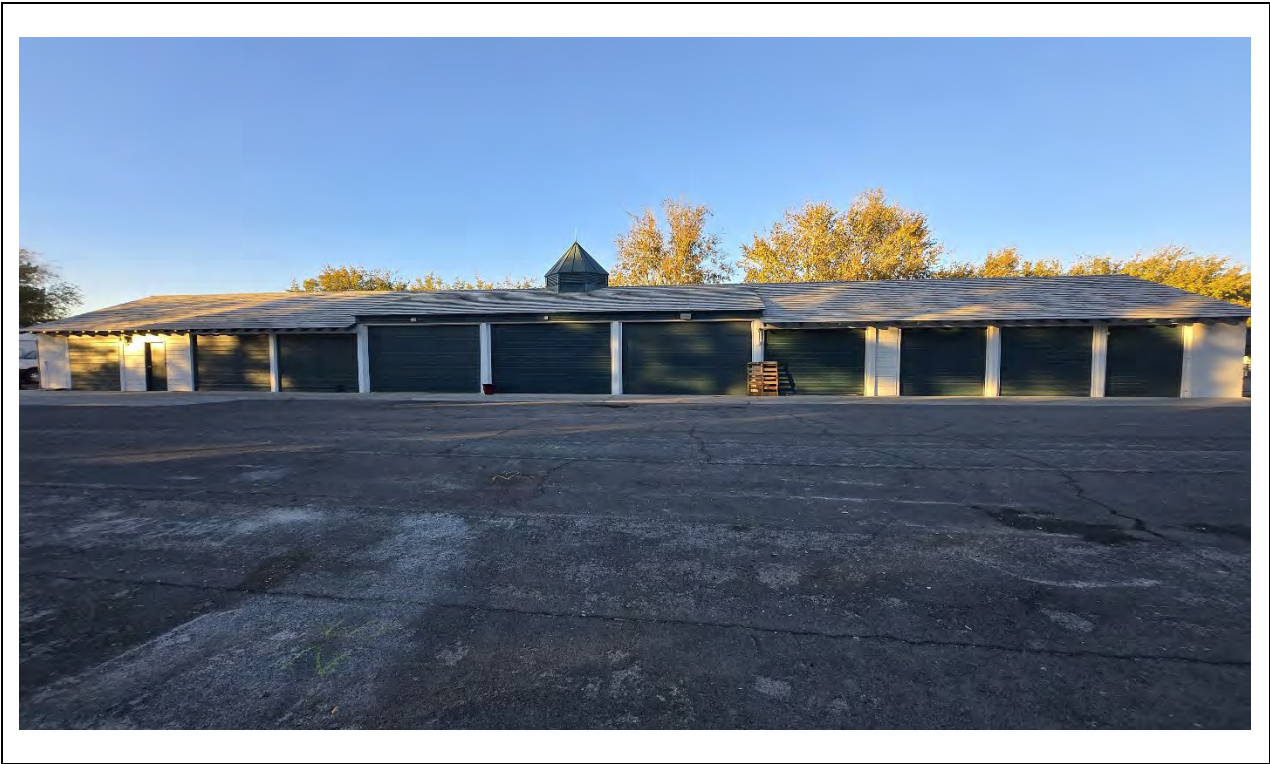
Machine Building/Firehouse – South elevation Kautz Environmental Consultants, Inc., November 2024
