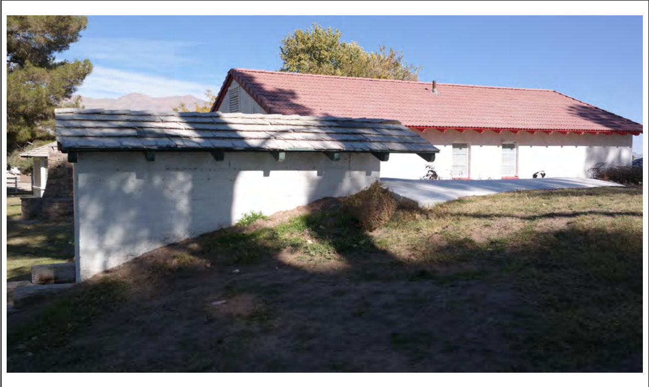
Root Cellar – Southwest elevation Kautz Environmental Consultants, Inc., November 2024
