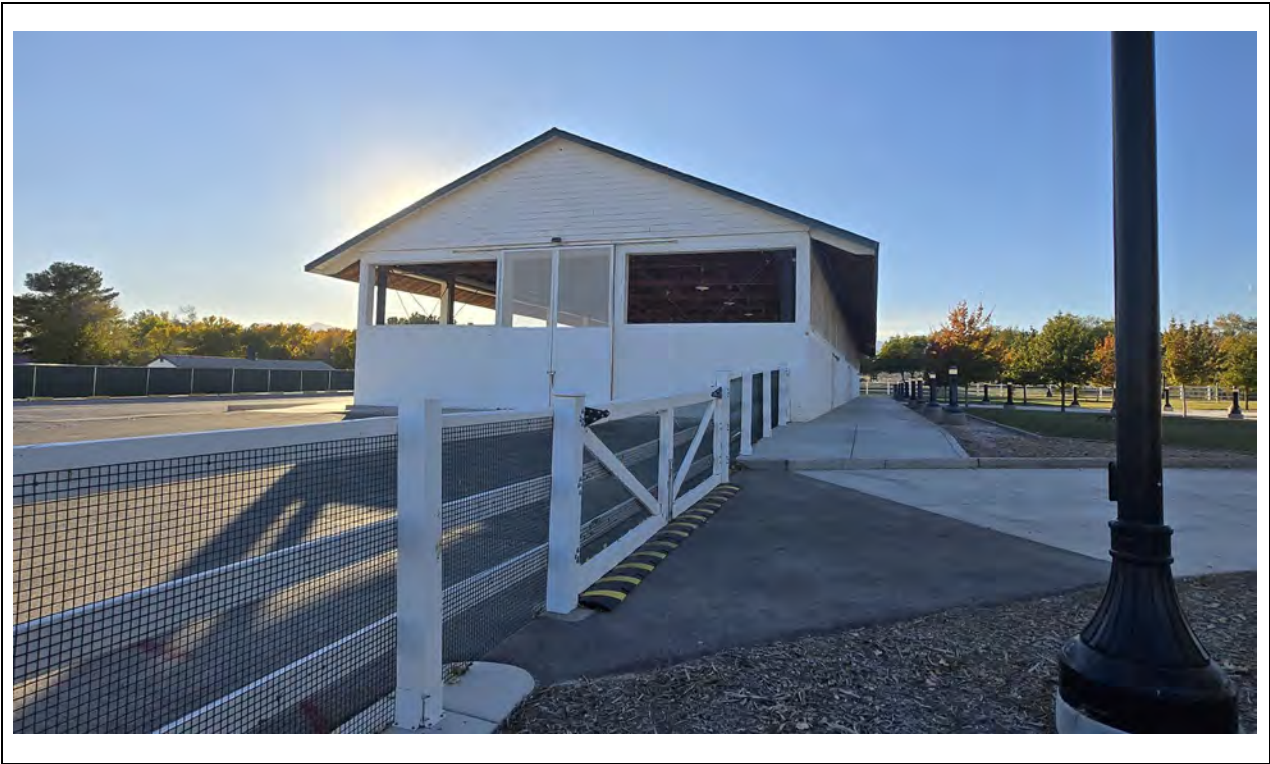
Hay Barn – East elevation
