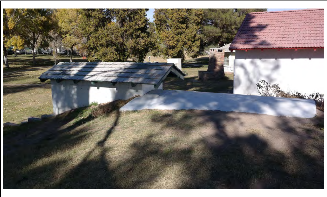
Root Cellar – Southwest elevation and south corner Kautz Environmental Consultants, Inc., November 2024
