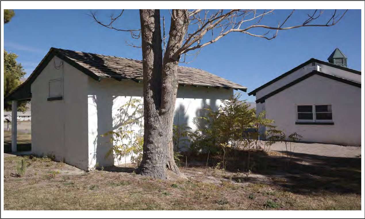
Bath House – Southwest corner overview Kautz Environmental Consultants, Inc., November 2024
