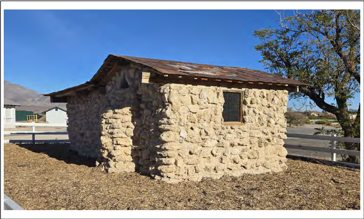
Adobe Hut – West corner Kautz Environmental Consultants, Inc., November 2024
