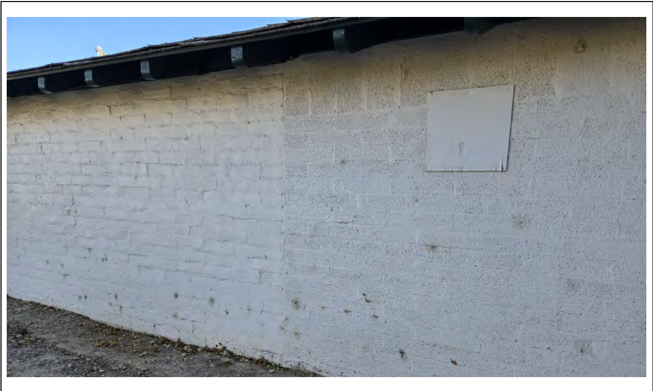
Office/Stables – North elevation, east/center Kautz Environmental Consultants, Inc., November 2024
