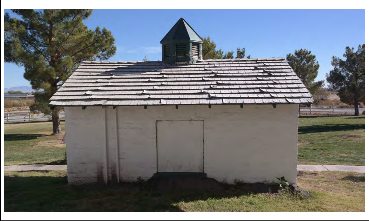
Power House – Northwest elevation Kautz Environmental Consultants, Inc., November 2024
