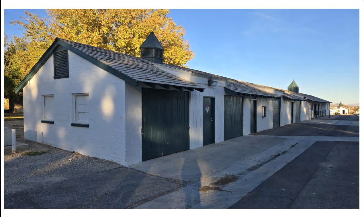
Office/Stables – Southwest corner Kautz Environmental Consultants, Inc., November 2024
