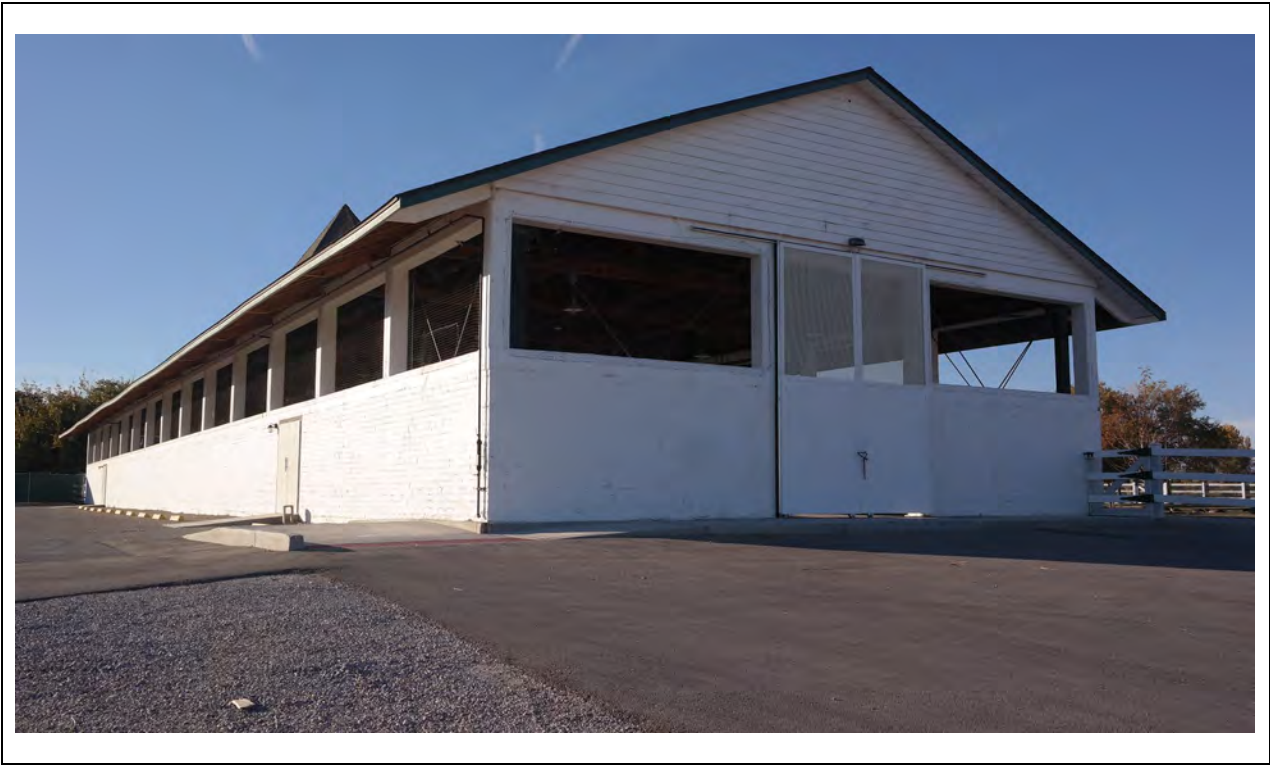
Hay Barn – East elevation and southeast corner Kautz Environmental Consultants, Inc., November 2024
