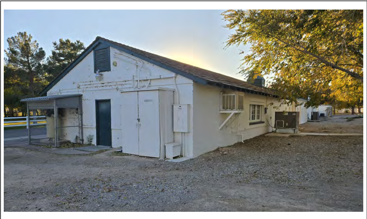
Machine Building/Firehouse – East elevation and northeast corner Kautz Environmental Consultants, Inc., November 2024
