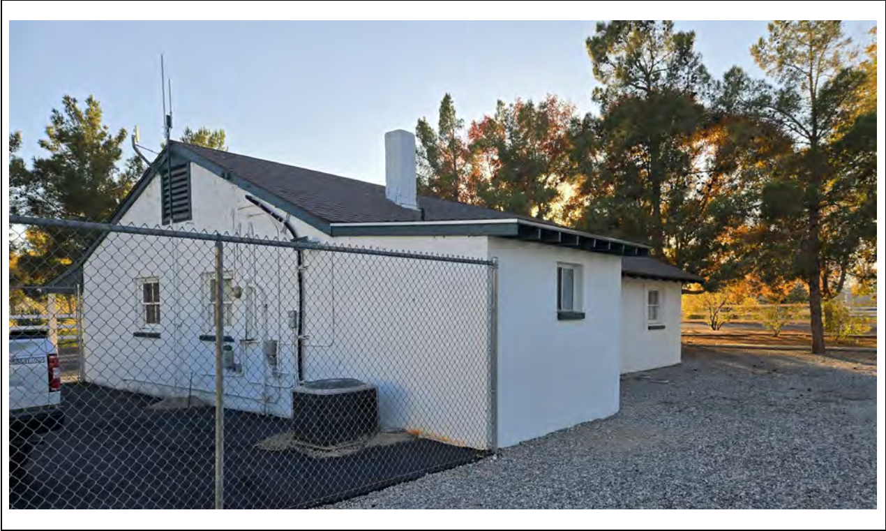
Caretaker's House – East elevation and northeast corner Kautz Environmental Consultants, Inc., November 2024
