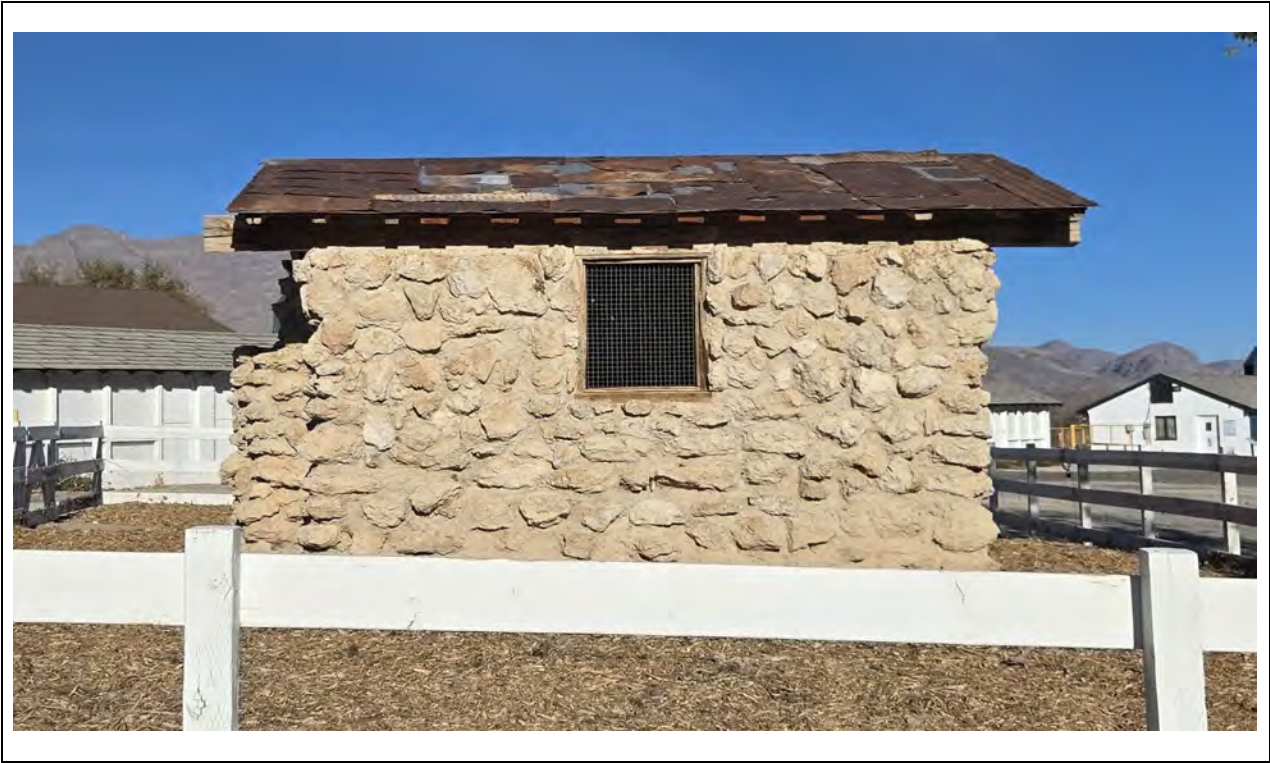
Adobe Hut – Southwest elevation Kautz Environmental Consultants, Inc., November 2024
