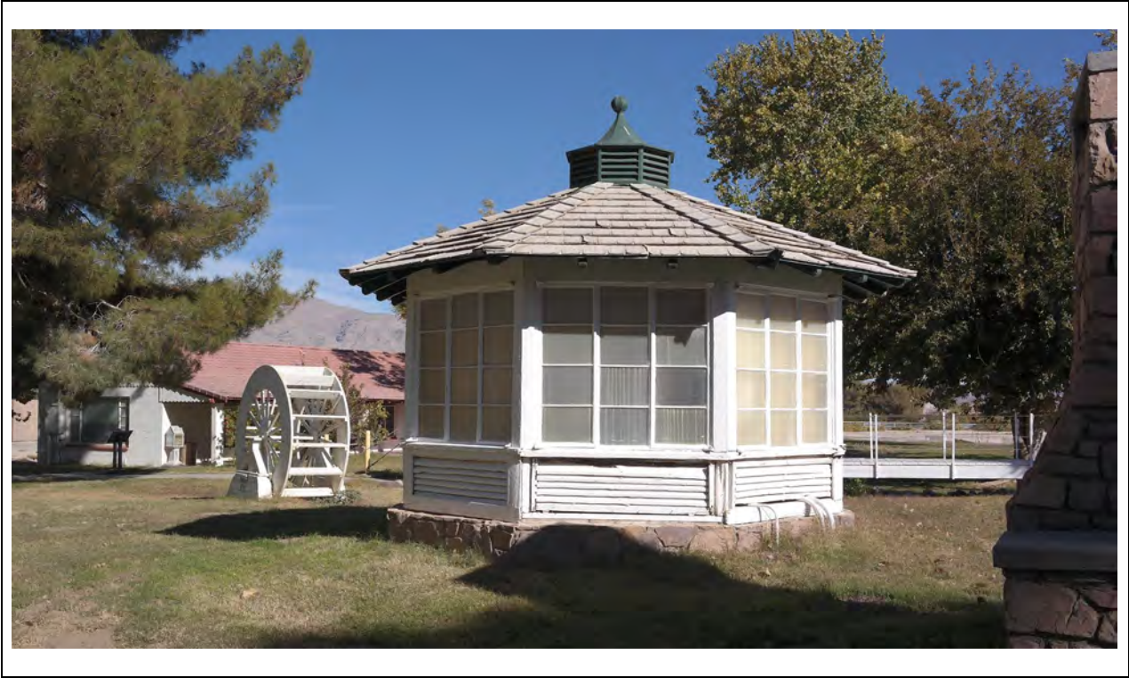
Pump House – Southwest elevation Kautz Environmental Consultants, Inc., November 2024
