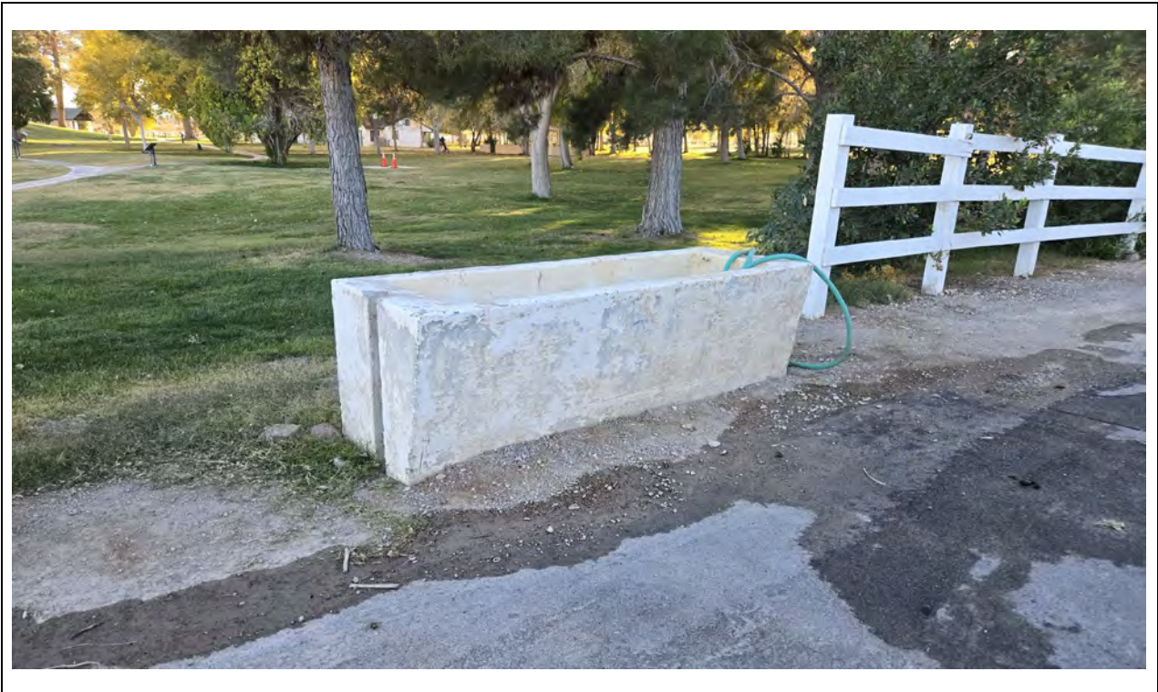
Office/Stables - Trough Kautz Environmental Consultants, Inc., November 2024
