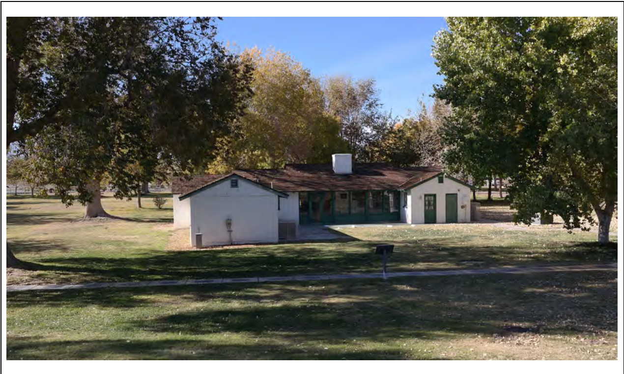
Foreman's House – East elevation overview Kautz Environmental Consultants, Inc., November 2024
