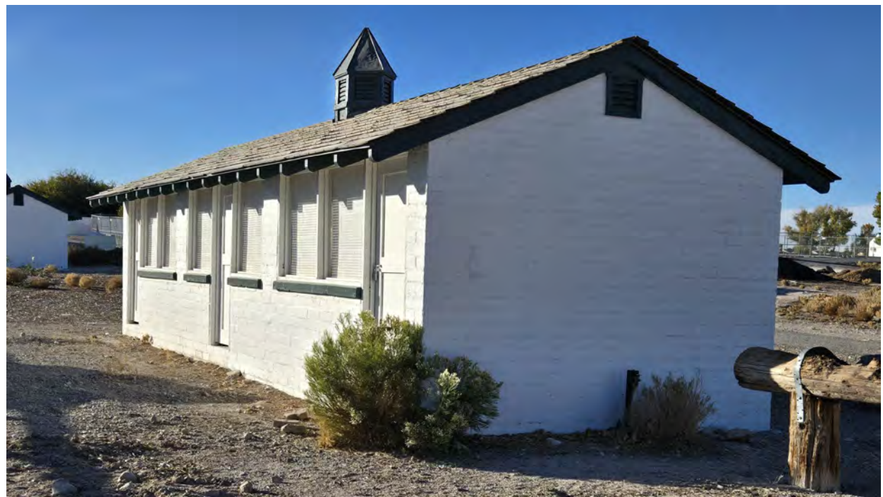
East Pig Housing – Southeast corner Kautz Environmental Consultants, Inc., November 2024
