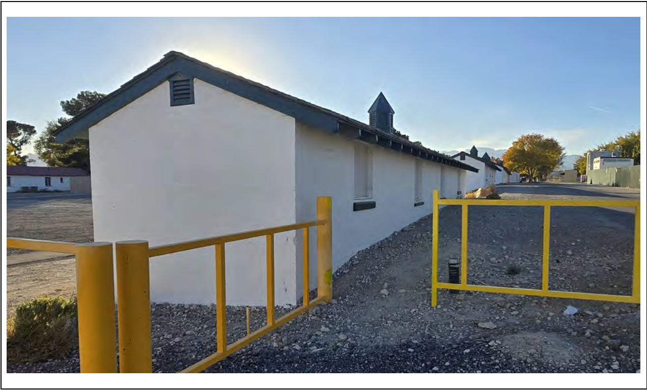
East Chicken Coop – East elevation and northeast corner Kautz Environmental Consultants, Inc., November 2024
