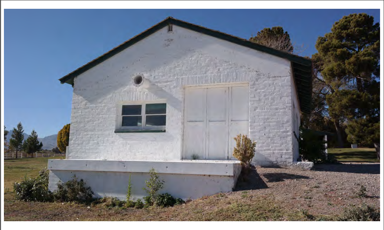
Generator Building – East elevation Kautz Environmental Consultants, Inc., November 2024
