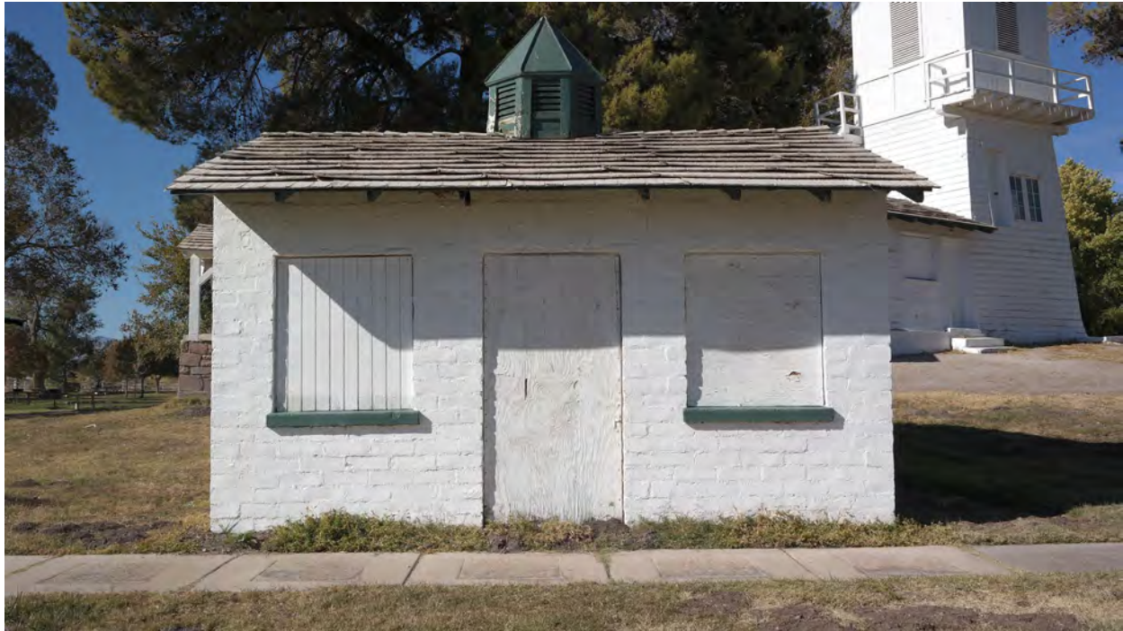
Power House – Southeast elevation
