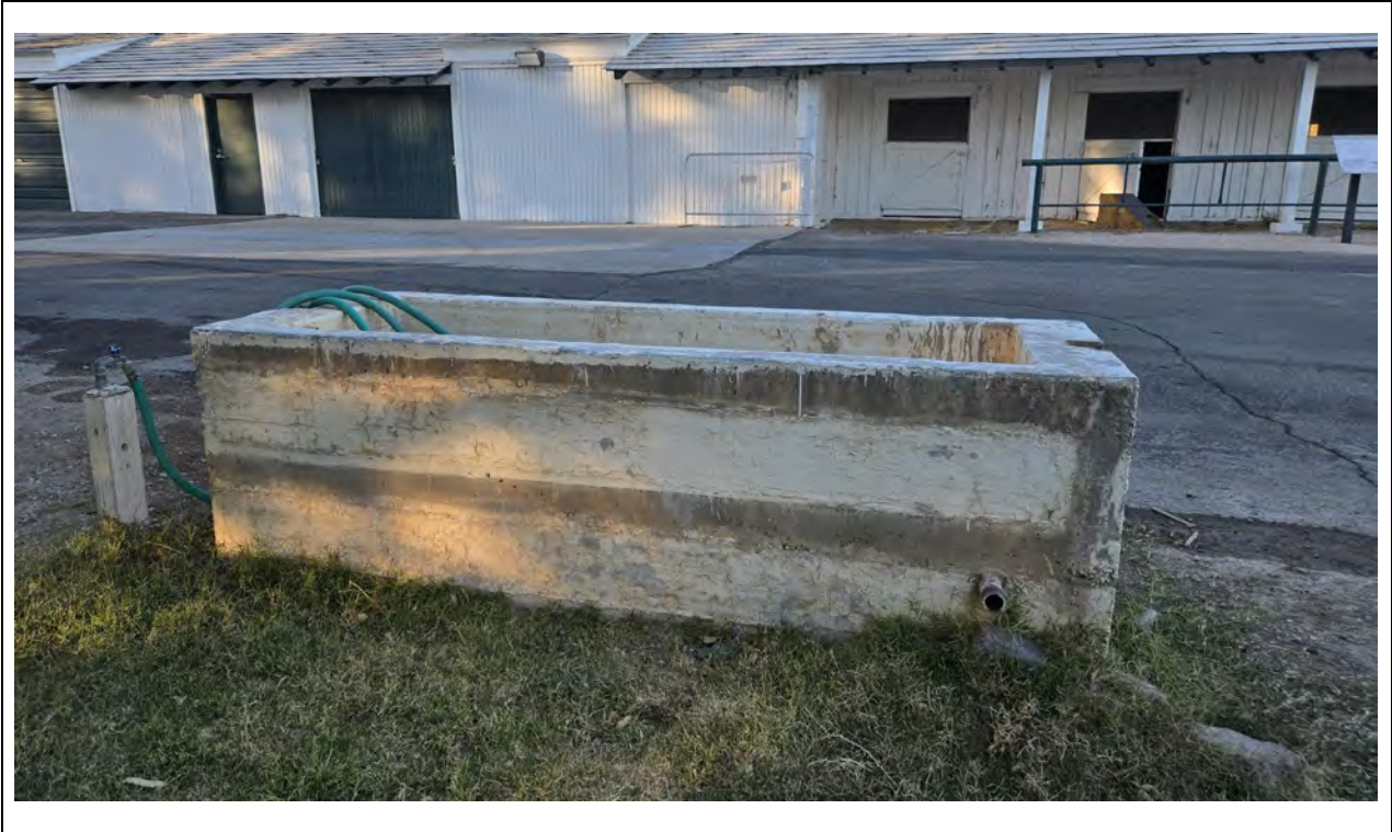
Office/Stables – Trough Kautz Environmental Consultants, Inc., November 2024
