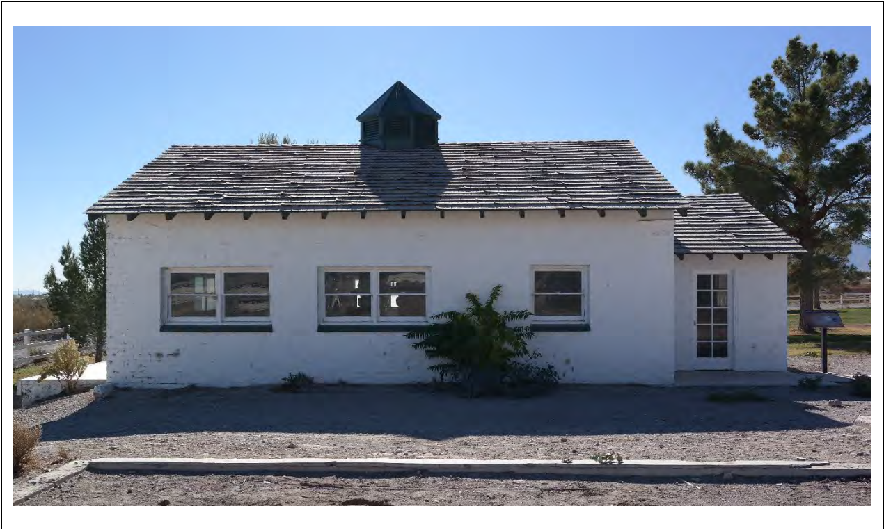
Generator Building – North elevation Kautz Environmental Consultants, Inc., November 2024
