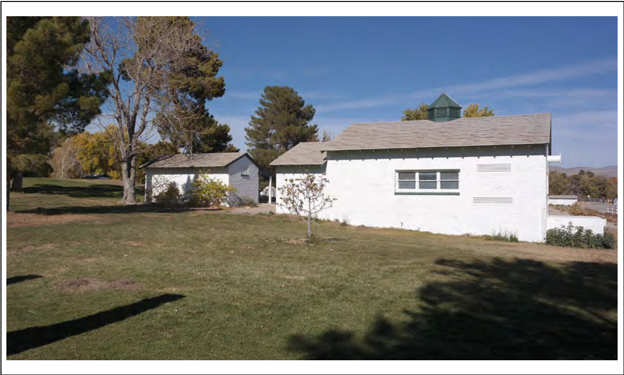
Generator Building – South elevation overview Kautz Environmental Consultants, Inc., November 2024
