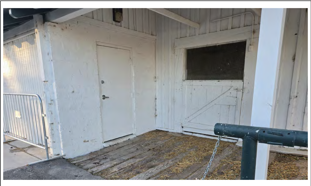
Office/Stables – South elevation, stable door detail Kautz Environmental Consultants, Inc., November 2024
