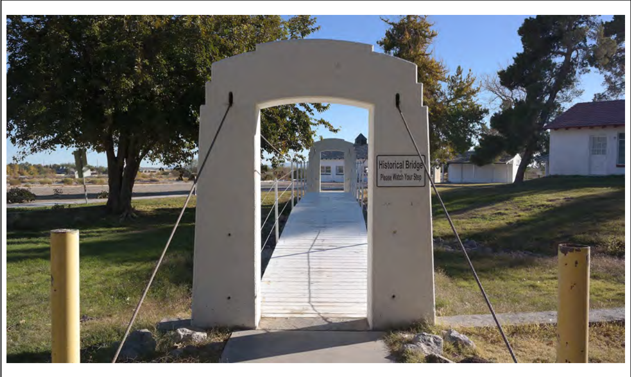
Suspension Bridge – North elevation Kautz Environmental Consultants, Inc., November 2024
