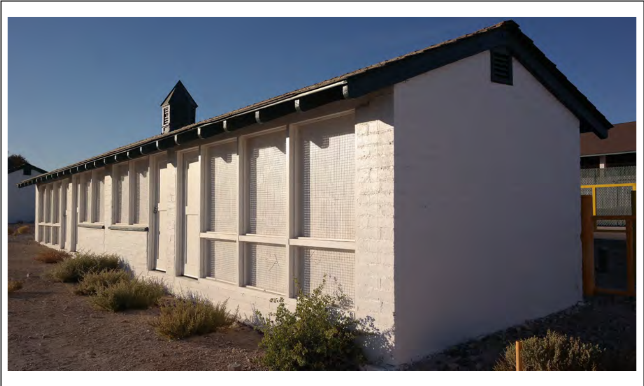
East Chicken Coop – Southeast corner Kautz Environmental Consultants, Inc., November 2024
