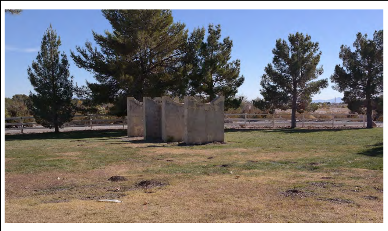
Diesel Oil Support – Northwest corner overview Kautz Environmental Consultants, Inc., November 2024
