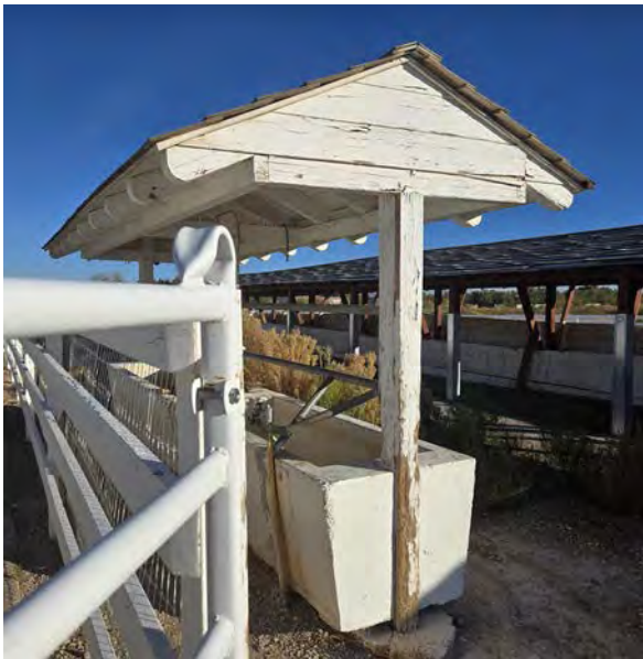
Covered Trough - NW corner 11.20.24
