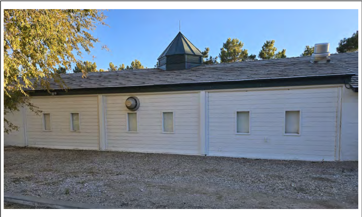
Machine Building/Firehouse – North elevation, center Kautz Environmental Consultants, Inc., November 2024
