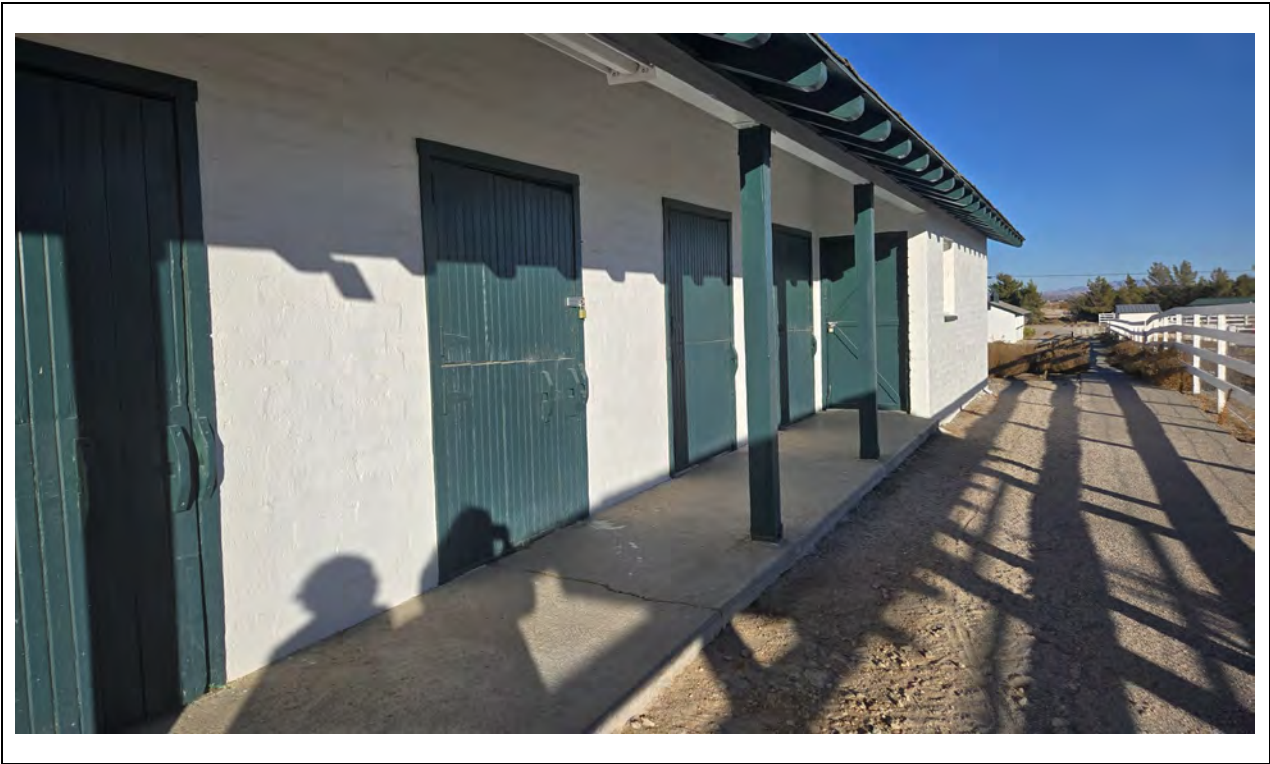
Cow Barn / Dairy Building – South elevation Kautz Environmental Consultants, Inc., November 2024
