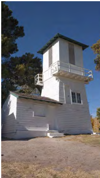
Water Tower - SE corner 11.20.14
