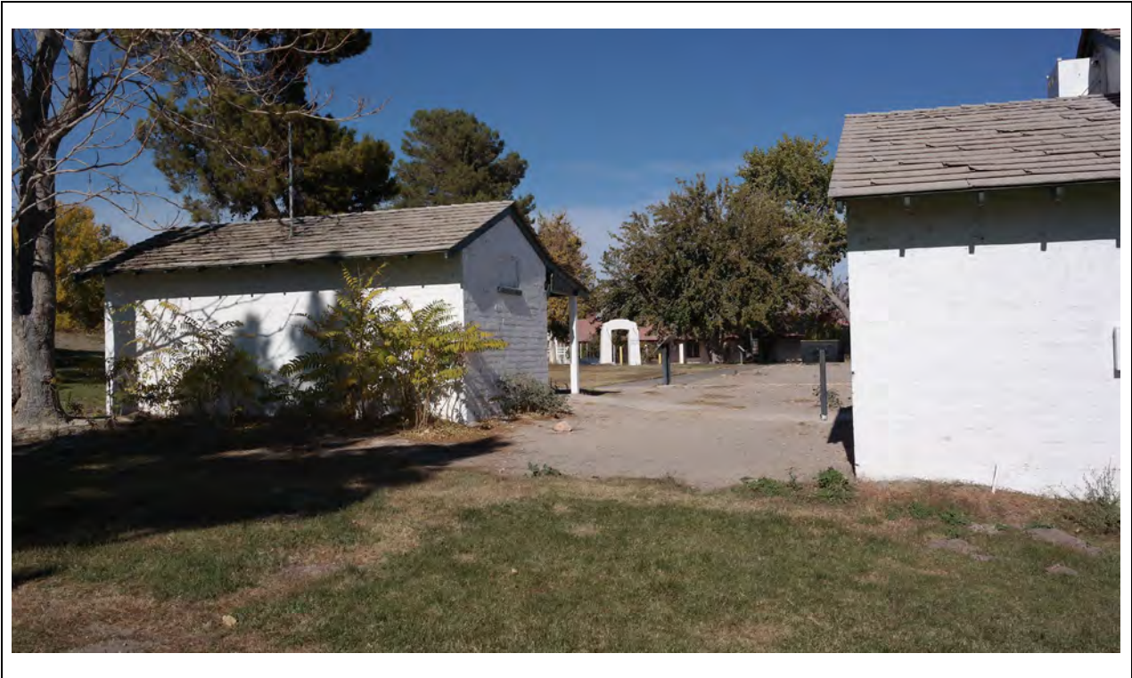
Bath House – Southeast corner overview Kautz Environmental Consultants, Inc., November 2024
