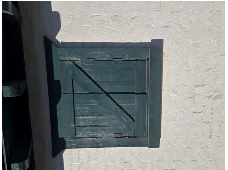
Cow Barn-Dairy - S window detail 11.20.24
