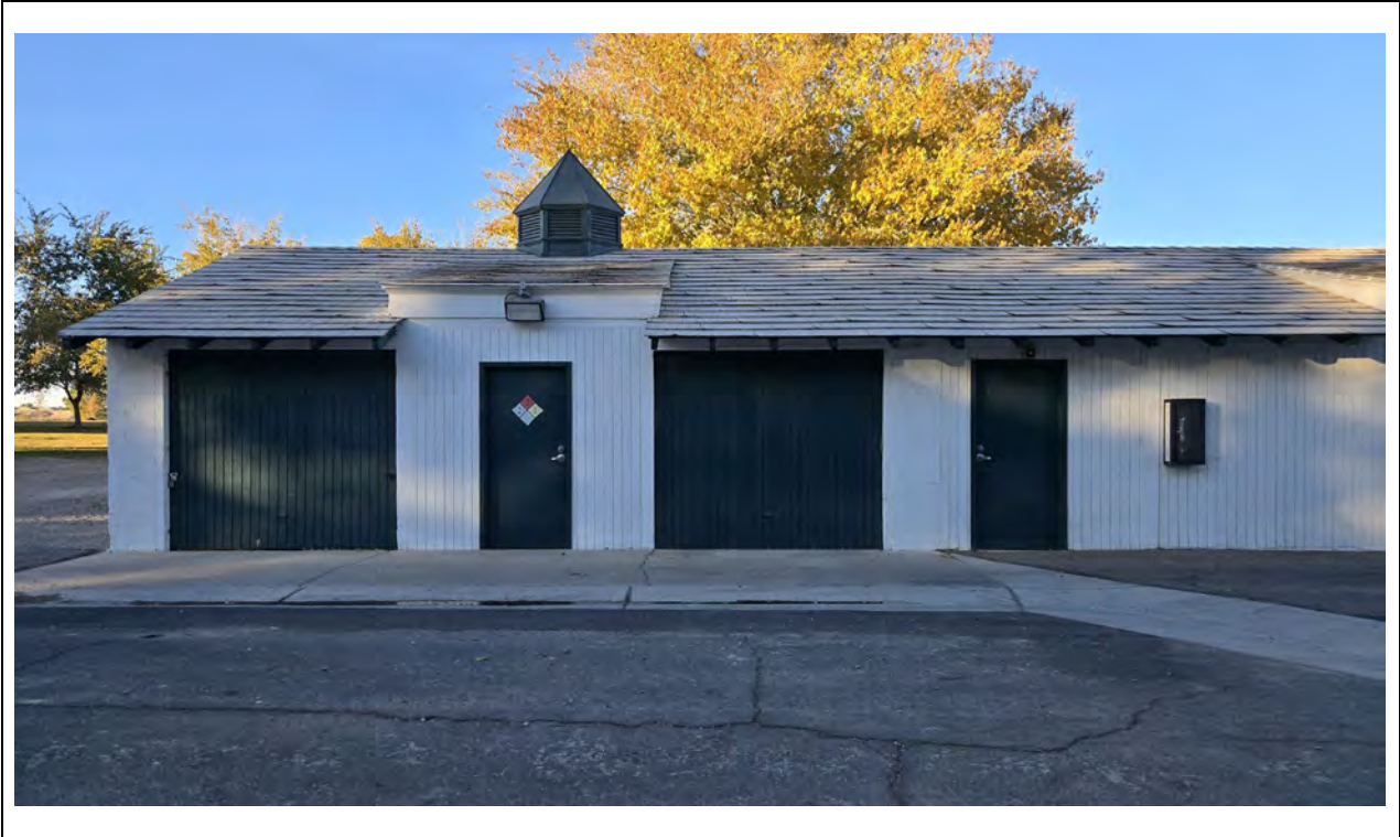
Office/Stables – South elevation, west end Kautz Environmental Consultants, Inc., November 2024
