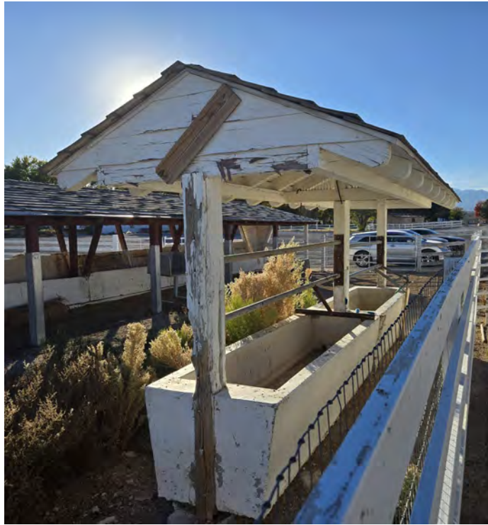
Covered Trough – Northeast corner
