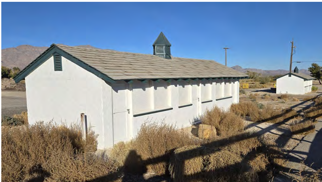
West Pig Housing – Southwest corner overview with East Pig Housing in background Kautz Environmental Consultants, Inc., November 2024
