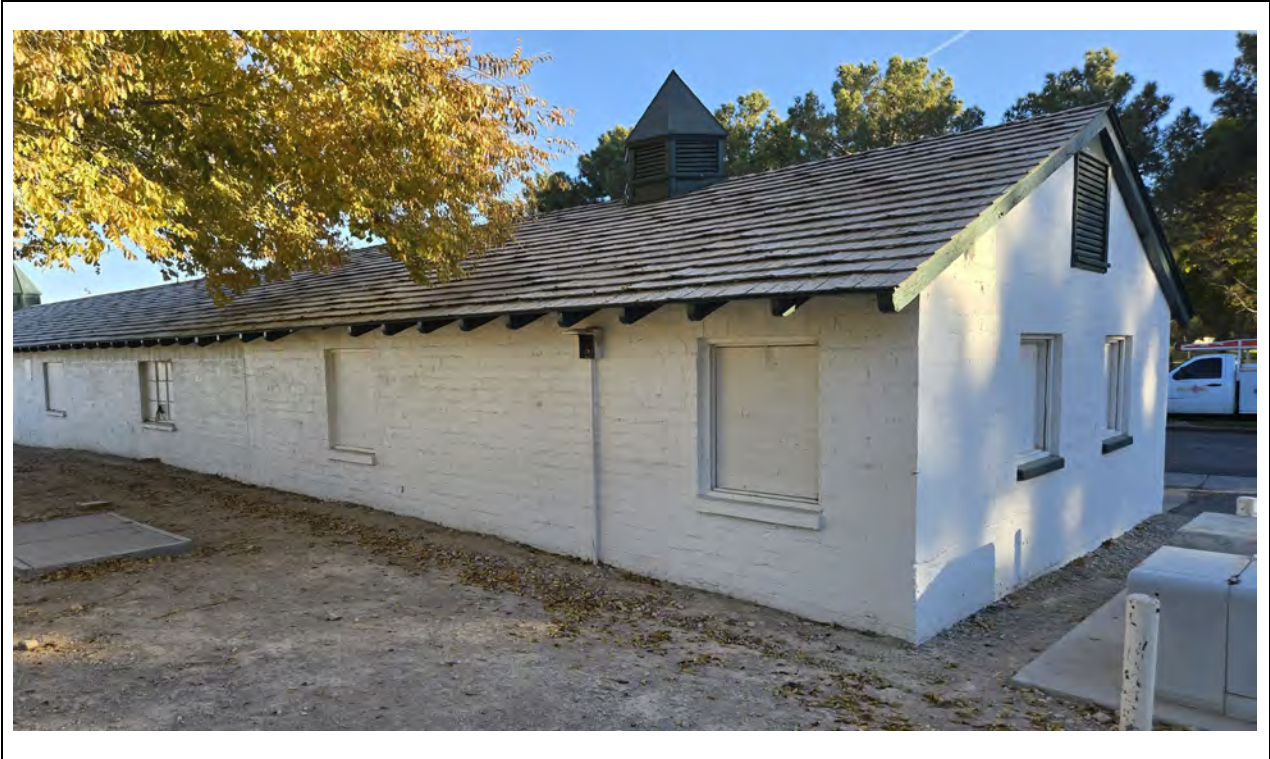
Office/Stables – Northwest corner and west elevation Kautz Environmental Consultants, Inc., November 2024
