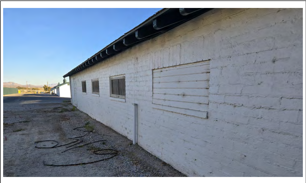
Office/Stables – North elevation, east end Kautz Environmental Consultants, Inc., November 2024
