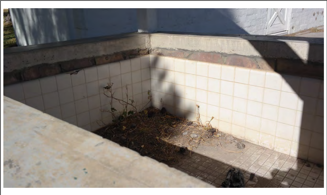
Well – Interior detail Kautz Environmental Consultants, Inc., November 2024
