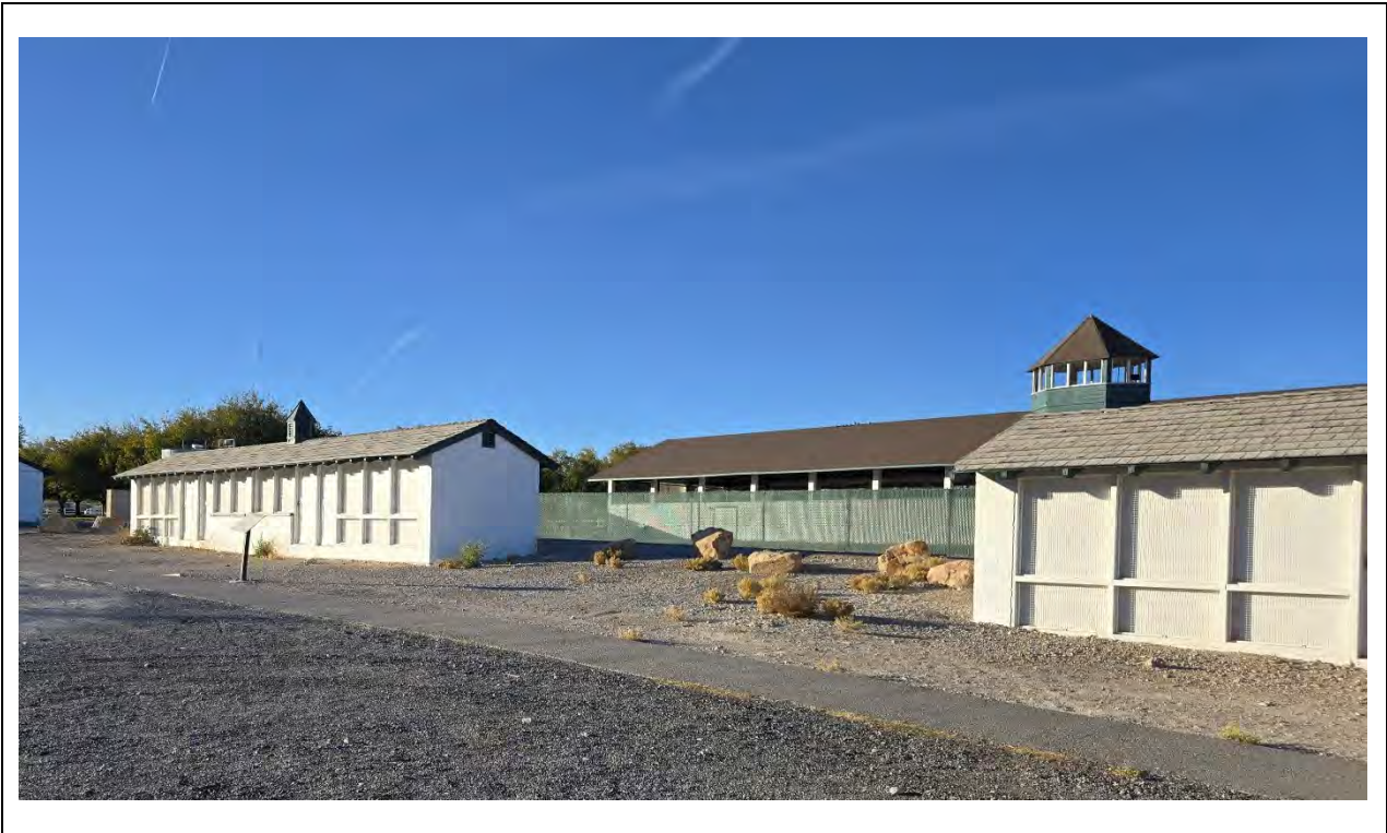
West Chicken Coop – Overview with East Chicken Coop on right Kautz Environmental Consultants, Inc., November 2024
