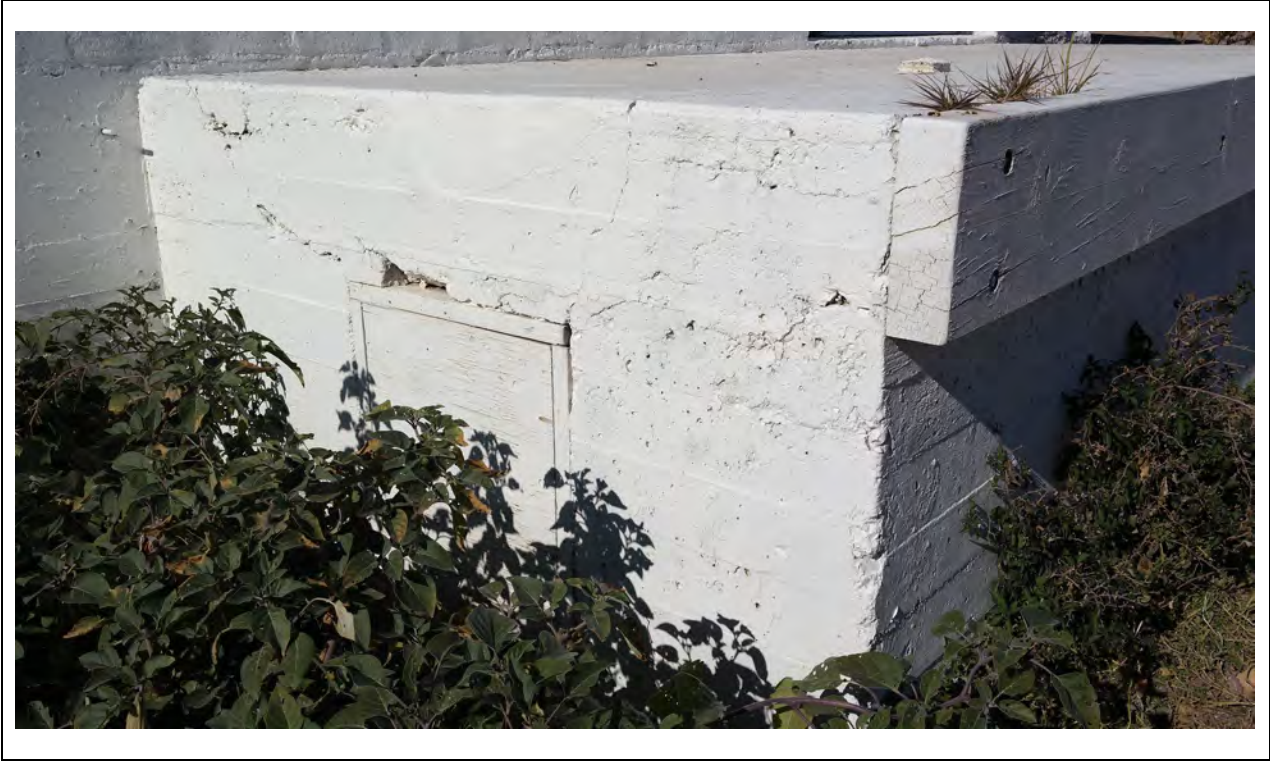
Generator Building – East elevation loading dock detail Kautz Environmental Consultants, Inc., November 2024
