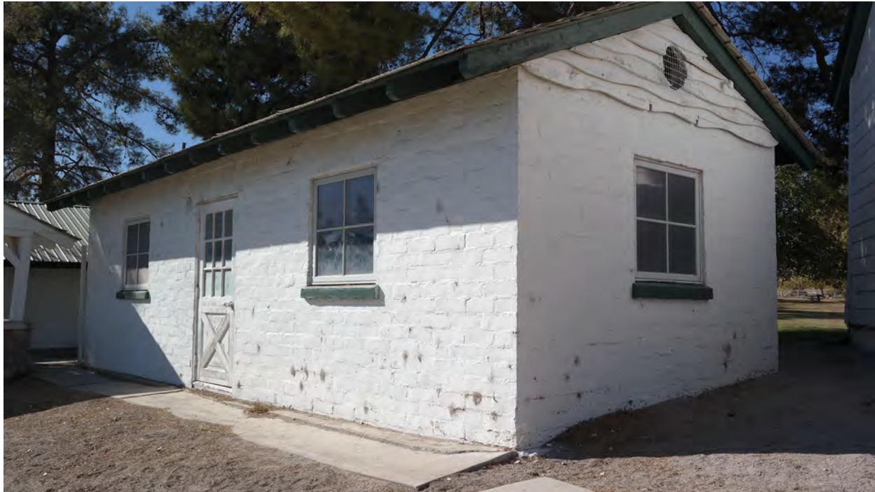
Spring House – East corner
