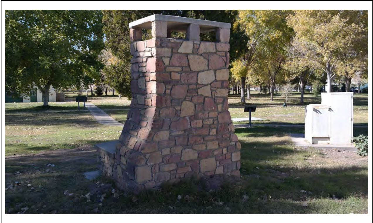
Outdoor Fireplace – East elevation and southeast corner Kautz Environmental Consultants, Inc., November 2024
