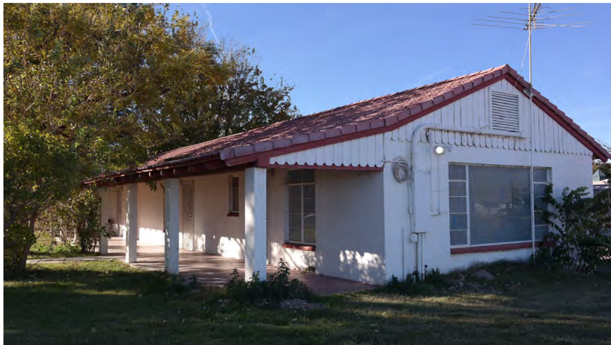
Guest House – Southeast corner
