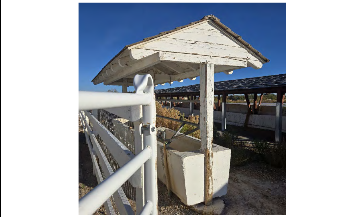
Covered Trough – Northwest corner Kautz Environmental Consultants, Inc., November 2024
