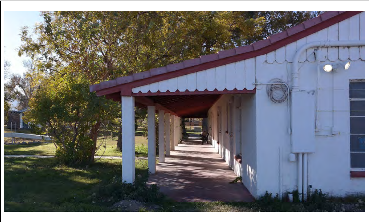
Guest House – East elevation and porch detail Kautz Environmental Consultants, Inc., November 2024
