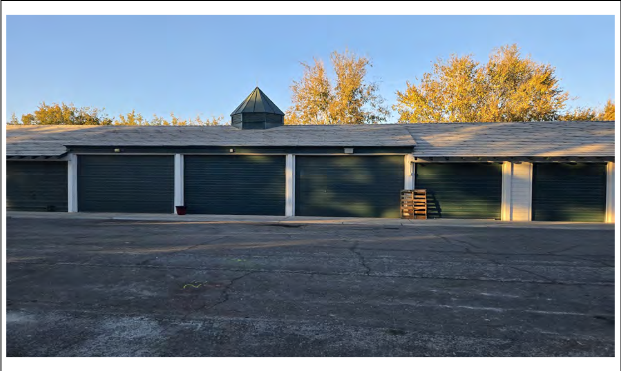
Machine Building/Firehouse – South elevation garage doors detail Kautz Environmental Consultants, Inc., November 2024
