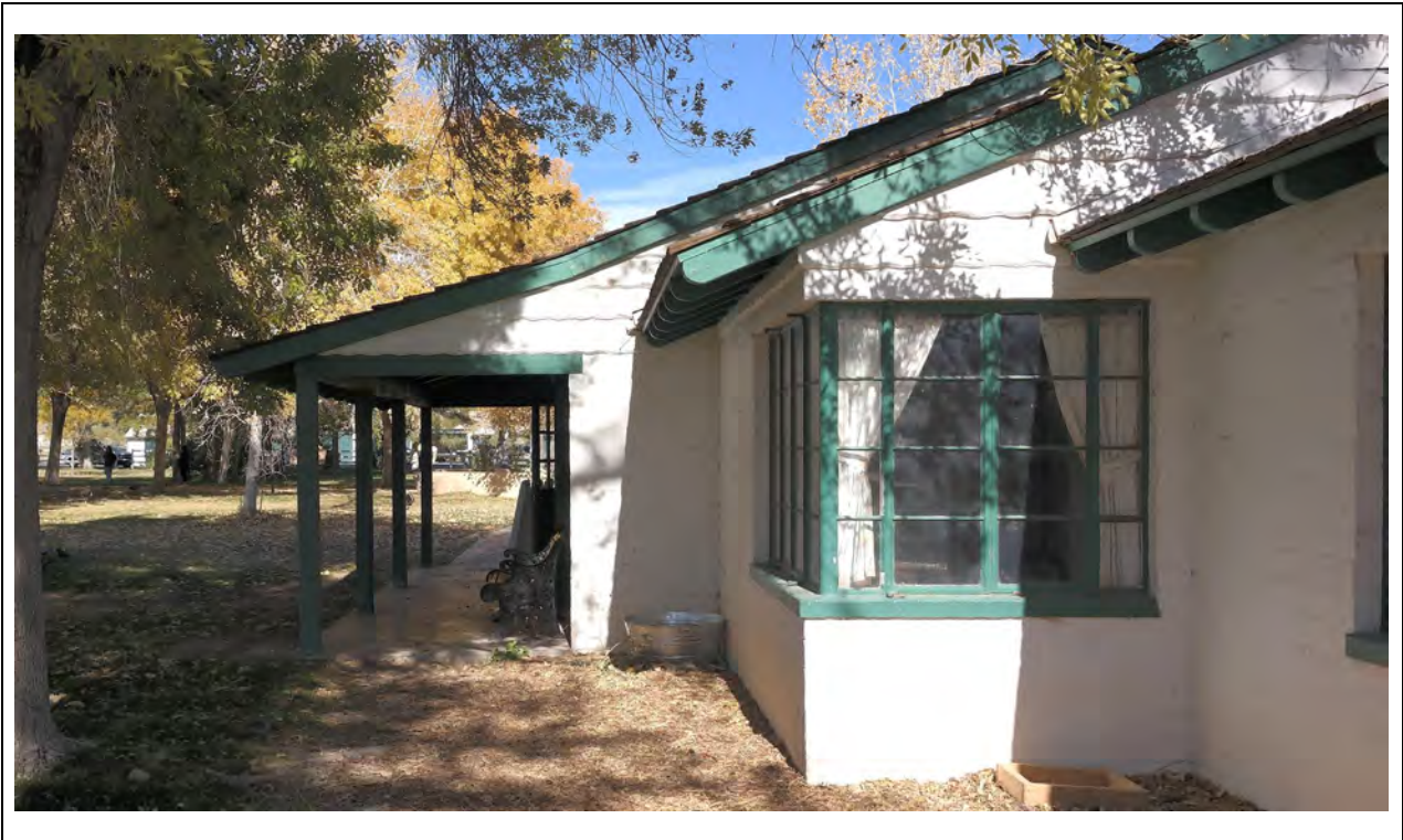
Foreman's House – West window and porch detail Kautz Environmental Consultants, Inc., November 2024
