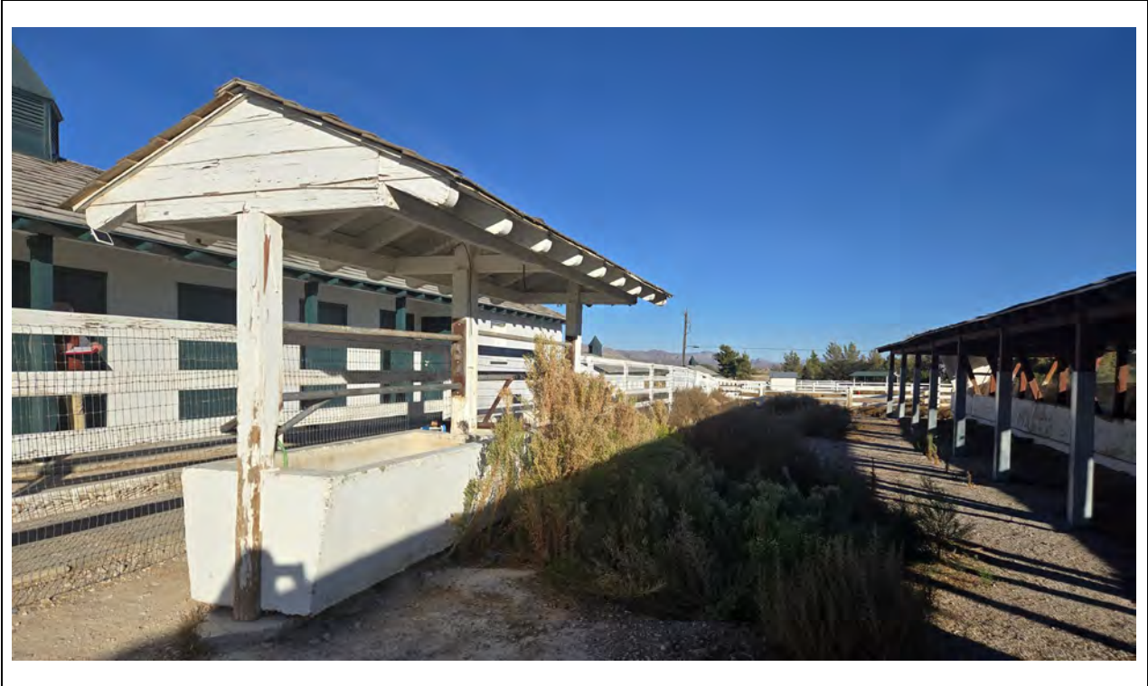
Covered Trough – Southwest corner Kautz Environmental Consultants, Inc., November 2024
