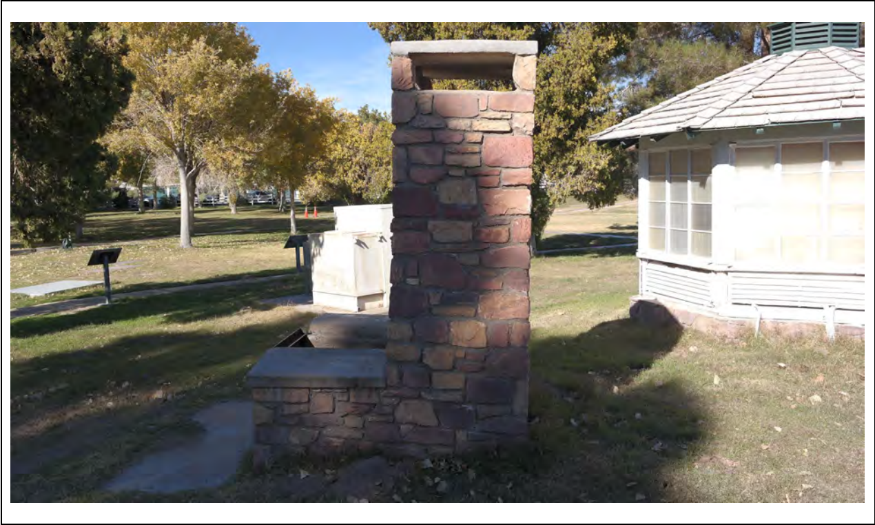
Outdoor Fireplace – South elevation Kautz Environmental Consultants, Inc., November 2024
