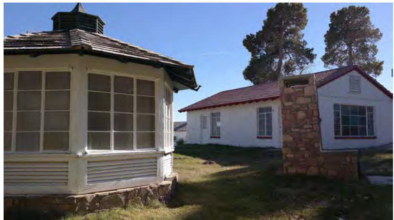
Overview - Near Water Wheel looking S 11.20.24
