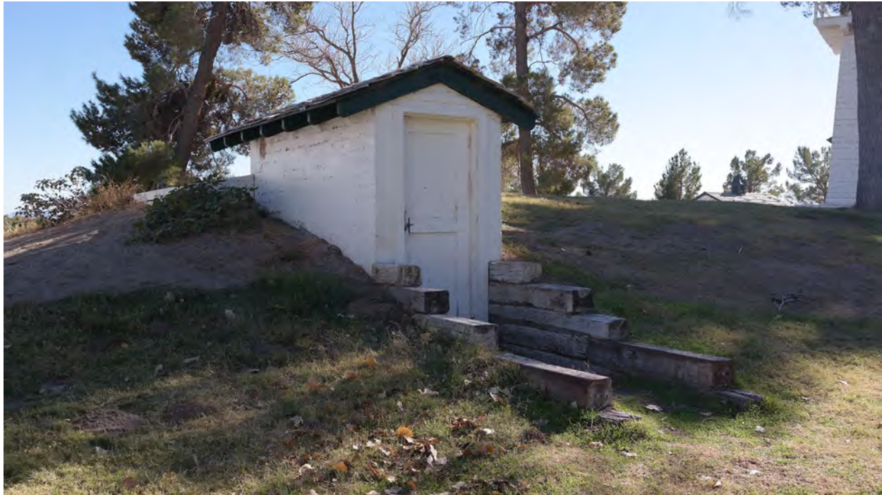
Root Cellar – North corner
