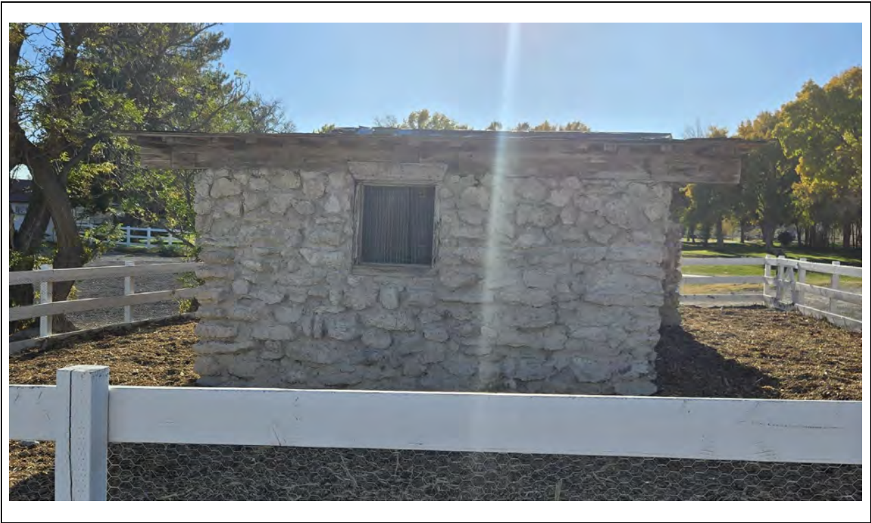
Adobe Hut – Northeast elevation Kautz Environmental Consultants, Inc., November 2024
