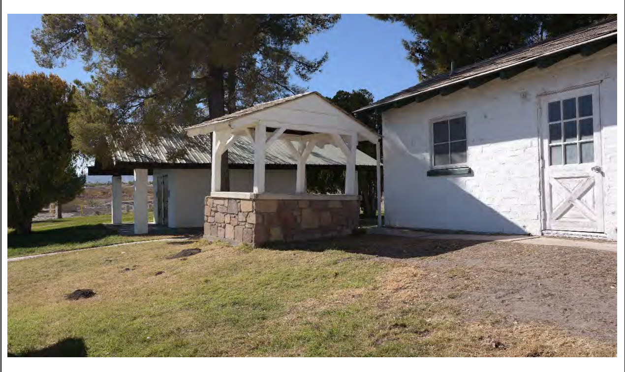
Well – Northeast corner overview with Spring House on right Kautz Environmental Consultants, Inc., November 2024
