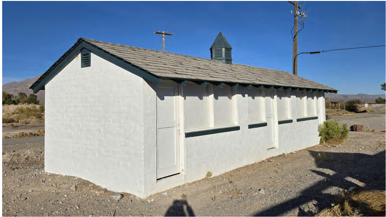
East Pig Housing – South elevation and southwest corner Kautz Environmental Consultants, Inc., November 2024
