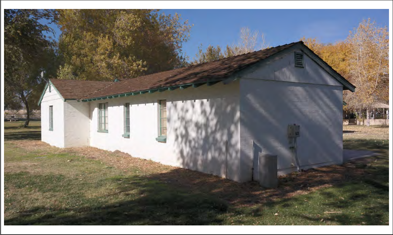
Foreman's House – Southeast corner Kautz Environmental Consultants, Inc., November 2024
