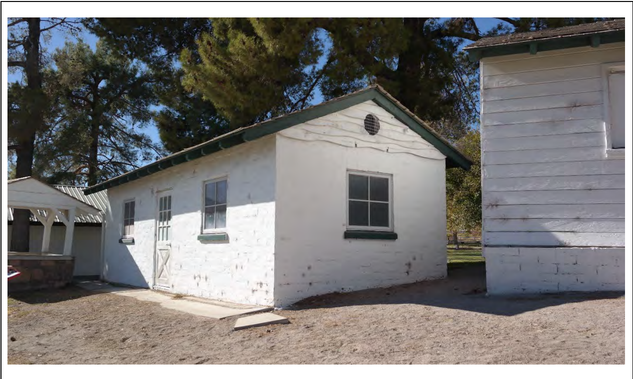
Spring House – East corner overview Kautz Environmental Consultants, Inc., November 2024
