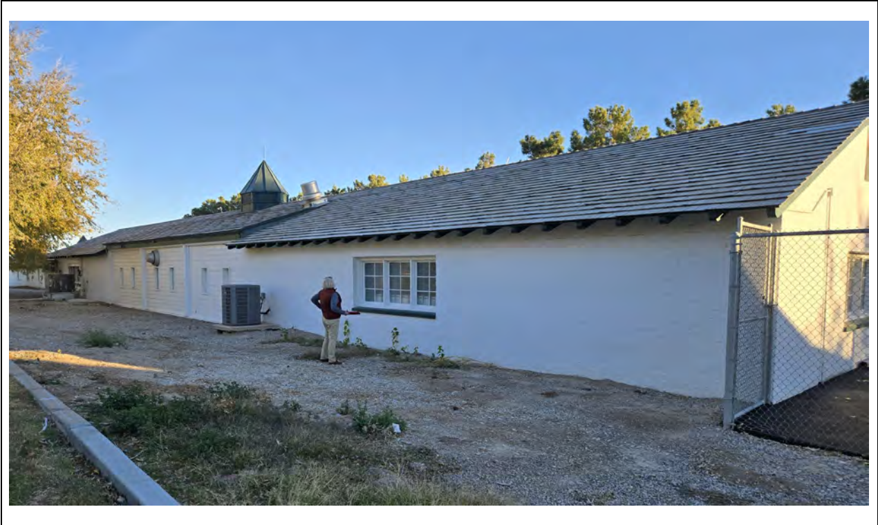
Machine Building/Firehouse – North elevation, west end Kautz Environmental Consultants, Inc., November 2024
