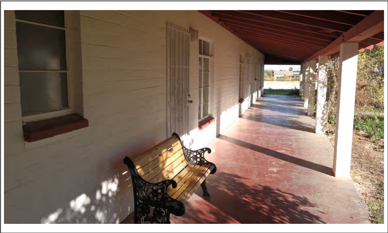
Guest House – South elevation porch Kautz Environmental Consultants, Inc., November 2024
