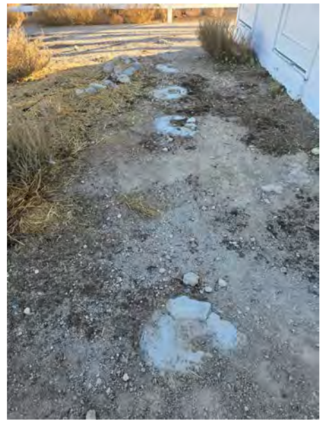
Cow Barn-Dairy - Former post detail 11.20.24
