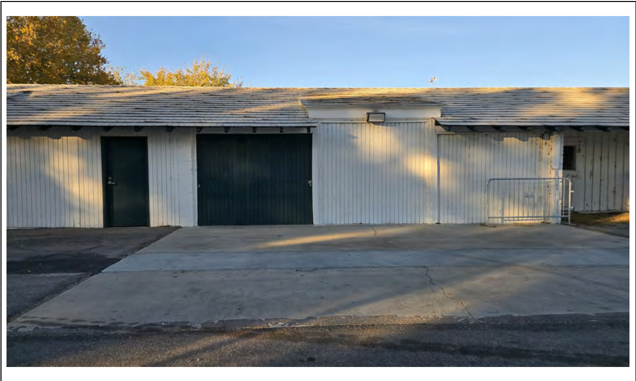
Office/Stables – South elevation, center Kautz Environmental Consultants, Inc., November 2024
