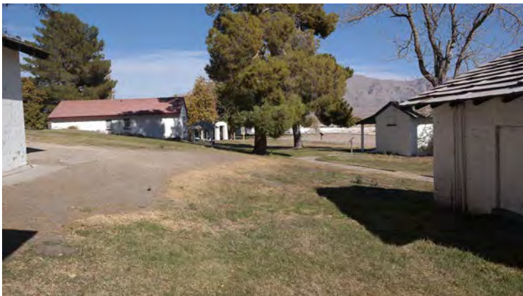
Overview - Near Power House looking NNE 11.20.24
