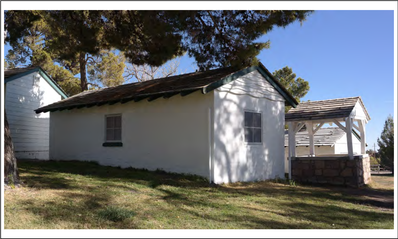
Spring House – West corner Kautz Environmental Consultants, Inc., November 2024
