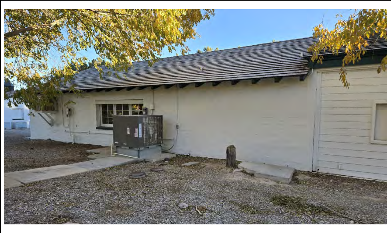
Machine Building/Firehouse – North elevation, east end Kautz Environmental Consultants, Inc., November 2024
