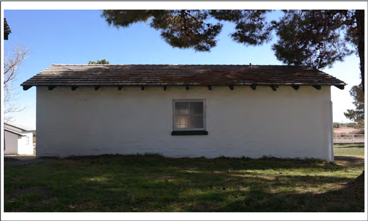
Spring House – Northwest elevation Kautz Environmental Consultants, Inc., November 2024
