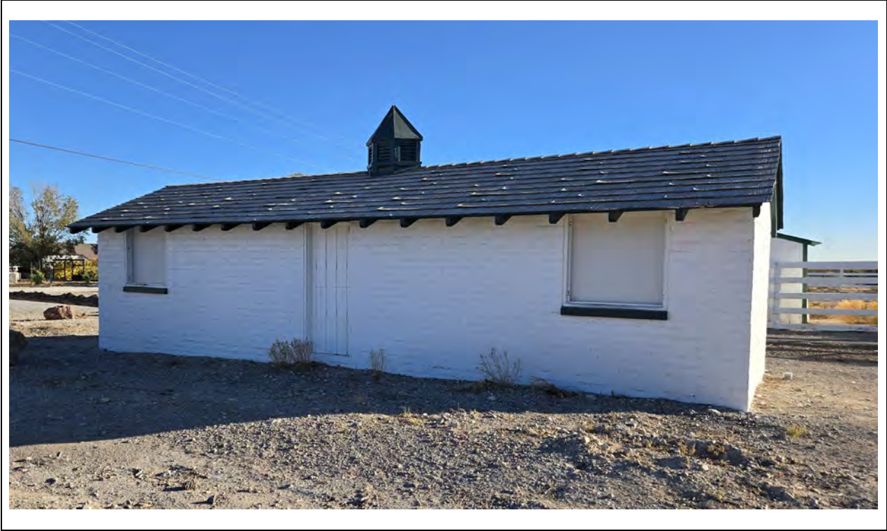
East Pig Housing – North elevation Kautz Environmental Consultants, Inc., November 2024
