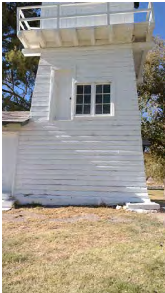
Water Tower - Siding detail E elev. 11.20.24
