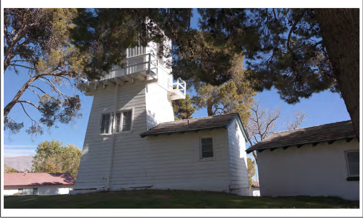
Water Tower – West elevation and southwest corner Kautz Environmental Consultants, Inc., November 2024
