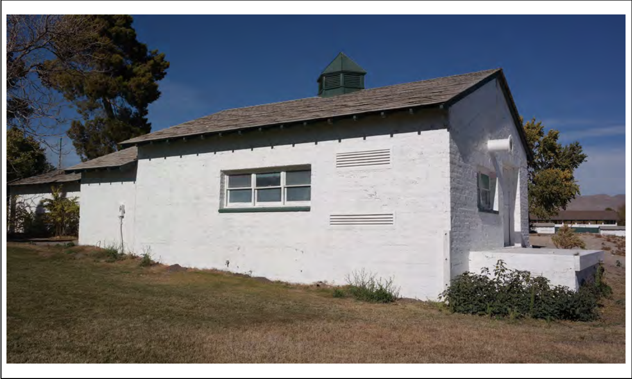
Generator Building – South elevation and southeast corner Kautz Environmental Consultants, Inc., November 2024
