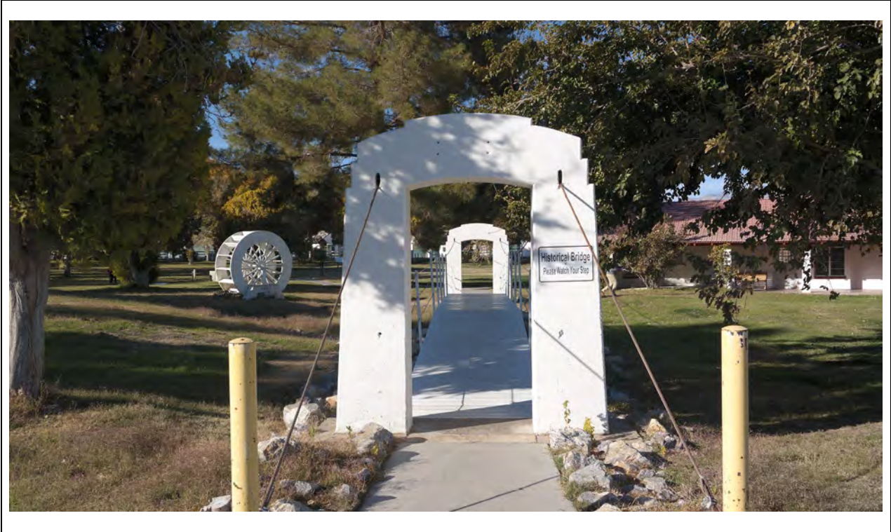
Suspension Bridge – South elevation Kautz Environmental Consultants, Inc., November 2024
