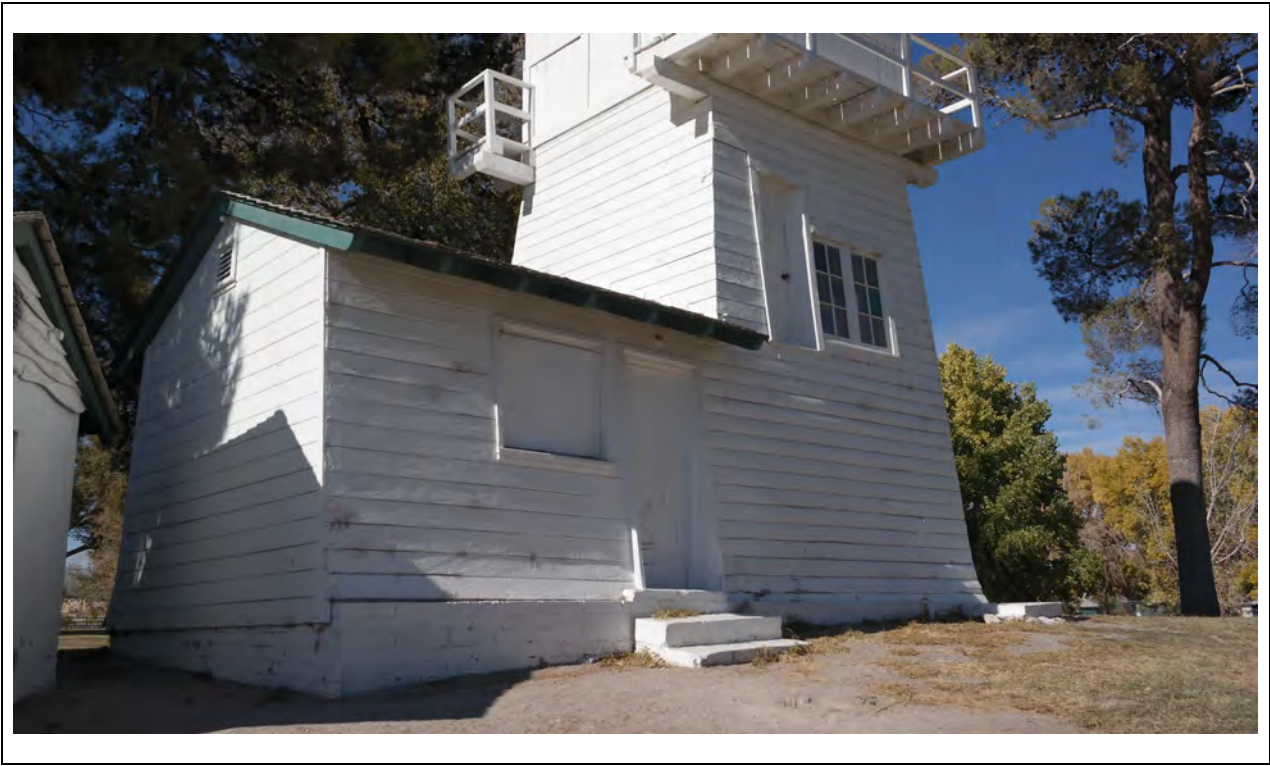
Water Tower – Southeast corner Kautz Environmental Consultants, Inc., November 2024
