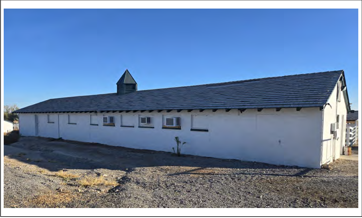
Cow Barn / Dairy Building – North elevation Kautz Environmental Consultants, Inc., November 2024
