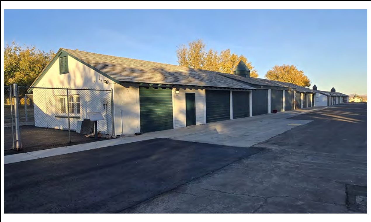
Machine Building/Firehouse – Southwest corner Kautz Environmental Consultants, Inc., November 2024
