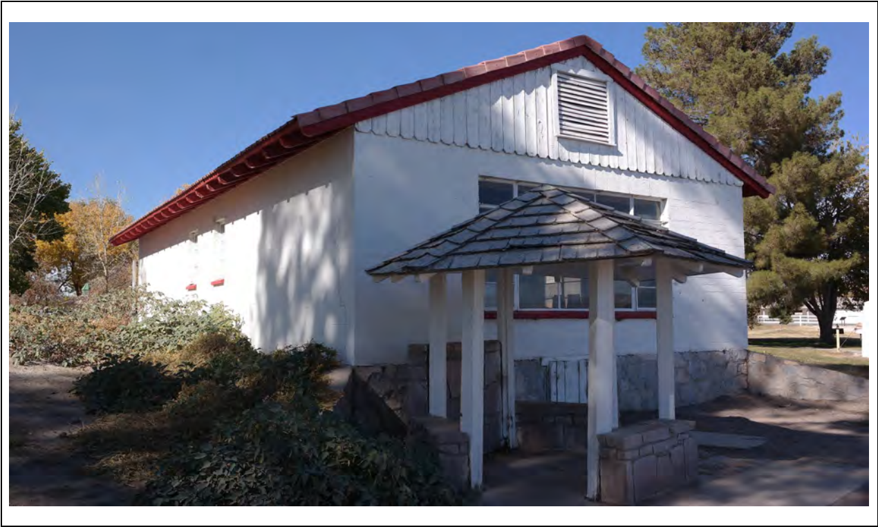
Duplex and Gazebo – South corner Kautz Environmental Consultants, Inc., November 2024
