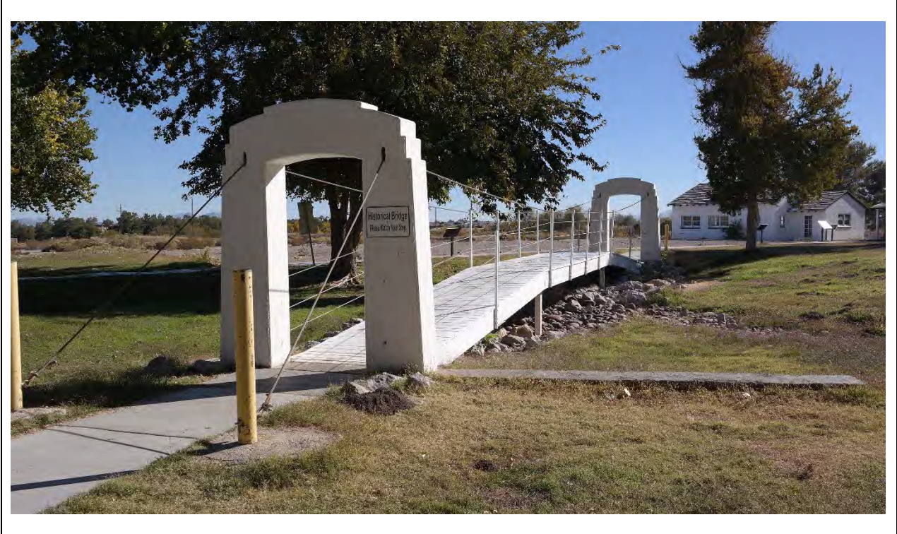
Suspension Bridge – Northwest corner Kautz Environmental Consultants, Inc., November 2024
