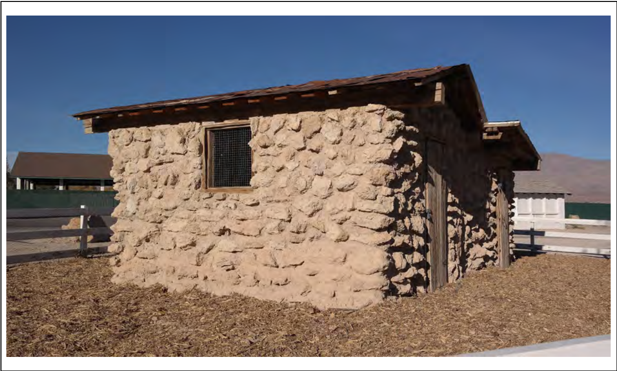
Adobe Hut – Southwest elevation and south corner Kautz Environmental Consultants, Inc., November 2024
