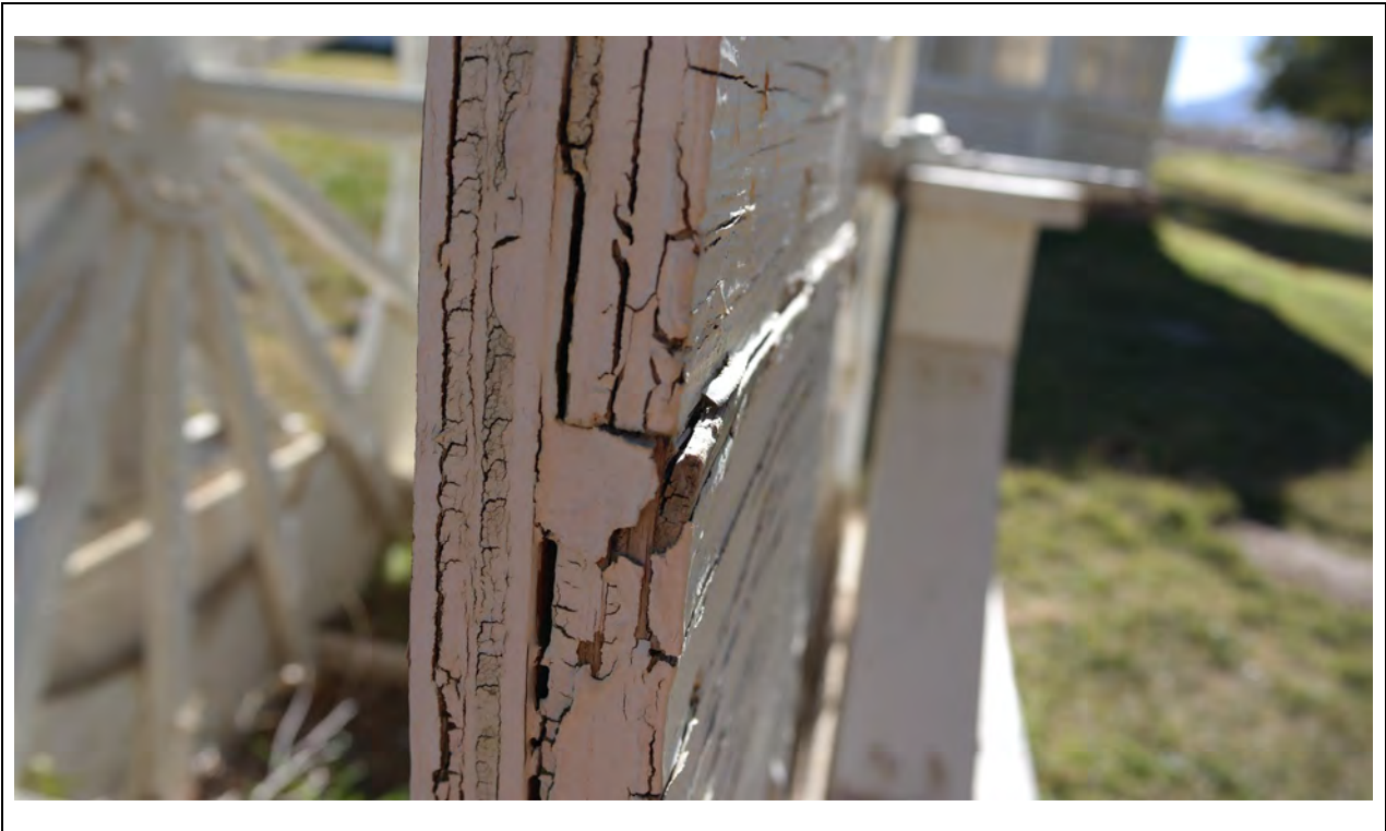
Water Wheel – Plywood detail Kautz Environmental Consultants, Inc., November 2024
