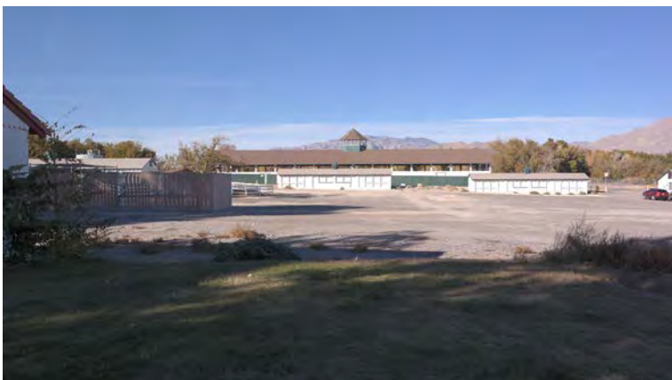
Overview - Near Guest House looking N 11.20.24
