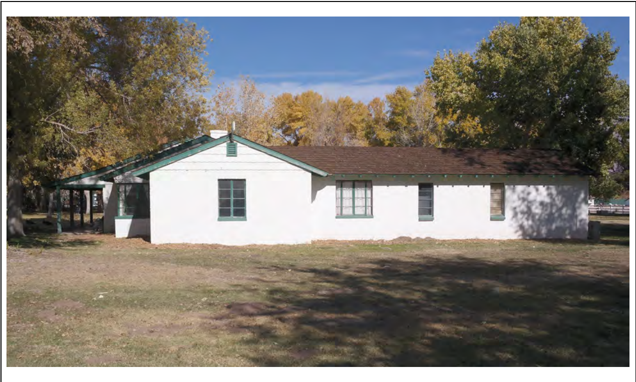
Foreman's House – South elevation Kautz Environmental Consultants, Inc., November 2024
