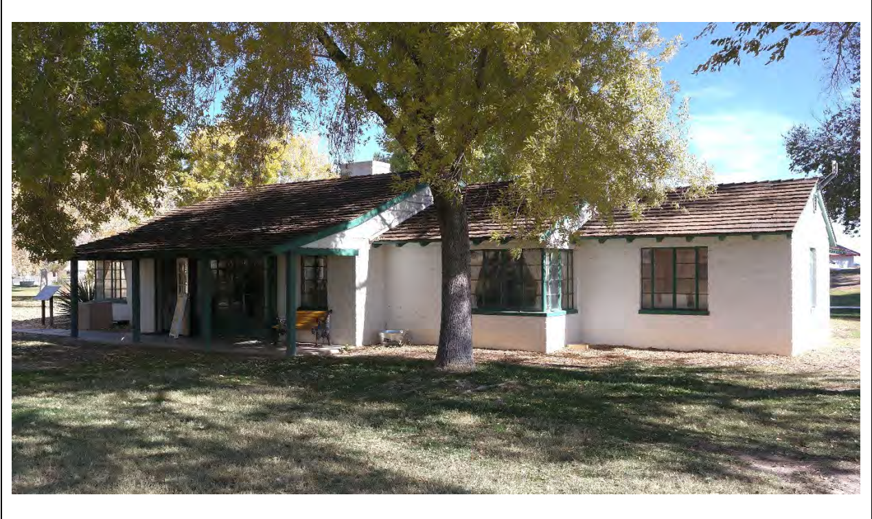
Foreman's House – West elevation and southwest corner Kautz Environmental Consultants, Inc., November 2024
