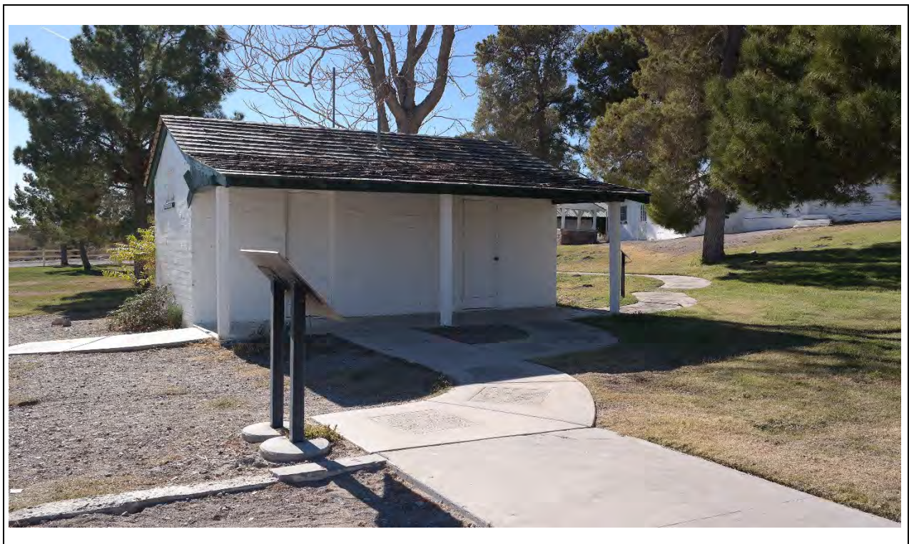
Bath House – North elevation overview
