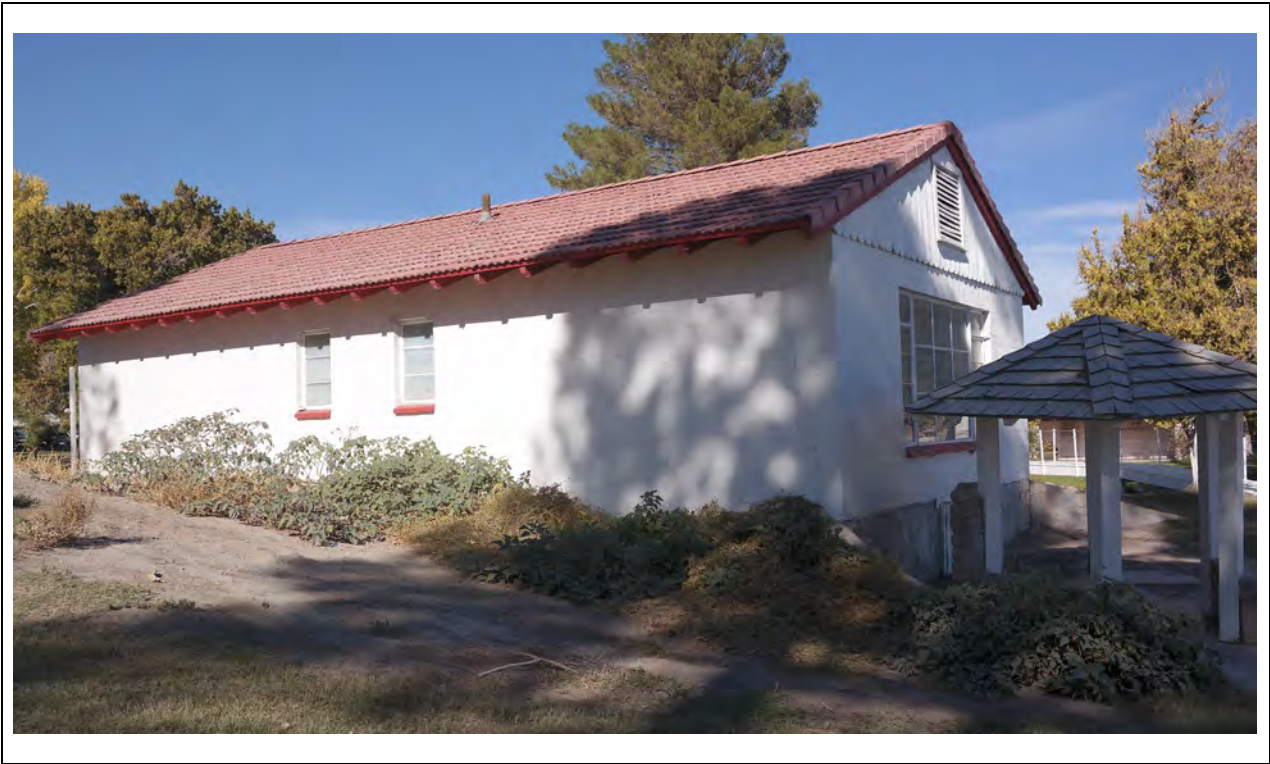
Duplex and Gazebo – Southwest elevation and south corner Kautz Environmental Consultants, Inc., November 2024
