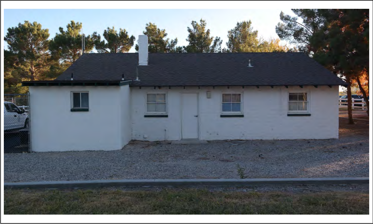
Caretaker's House – North elevation Kautz Environmental Consultants, Inc., November 2024
