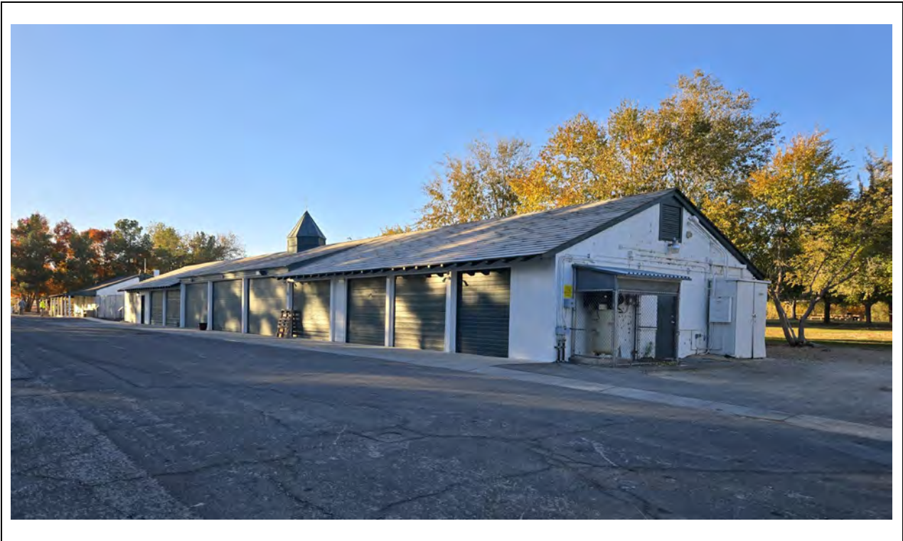
Machine Building/Firehouse – Southeast corner Kautz Environmental Consultants, Inc., November 2024
