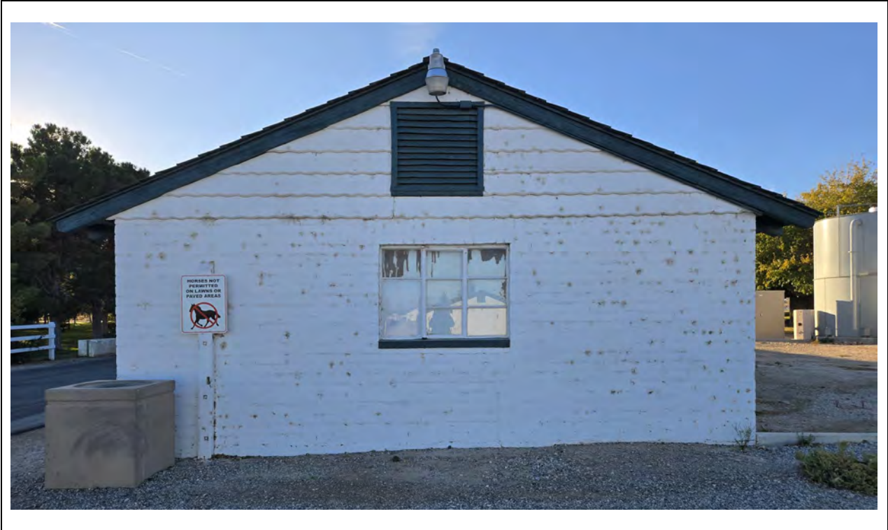
Office/Stables – East elevation Kautz Environmental Consultants, Inc., November 2024
