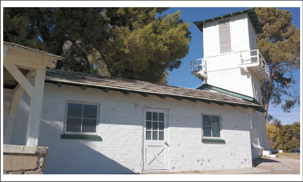
Spring House – Southeast elevation with Water Tower in background Kautz Environmental Consultants, Inc., November 2024
