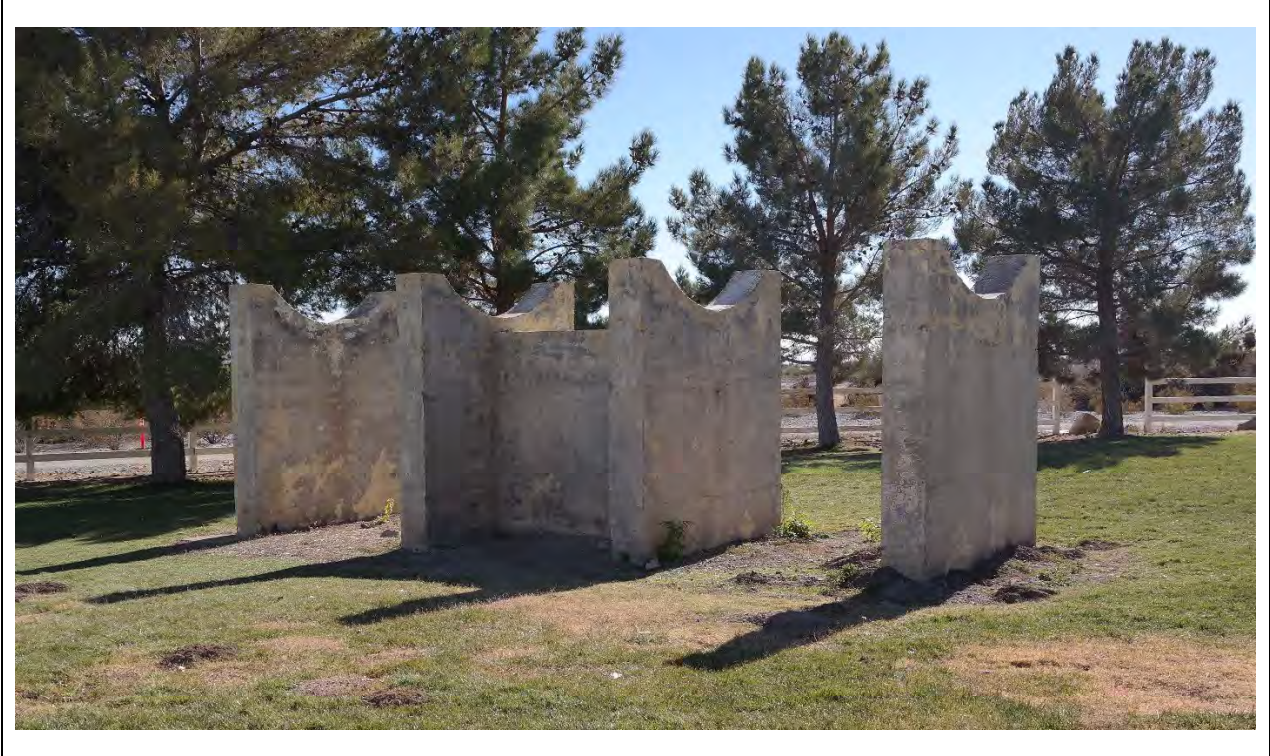
Diesel Oil Support – Northwest corner Kautz Environmental Consultants, Inc., November 2024
