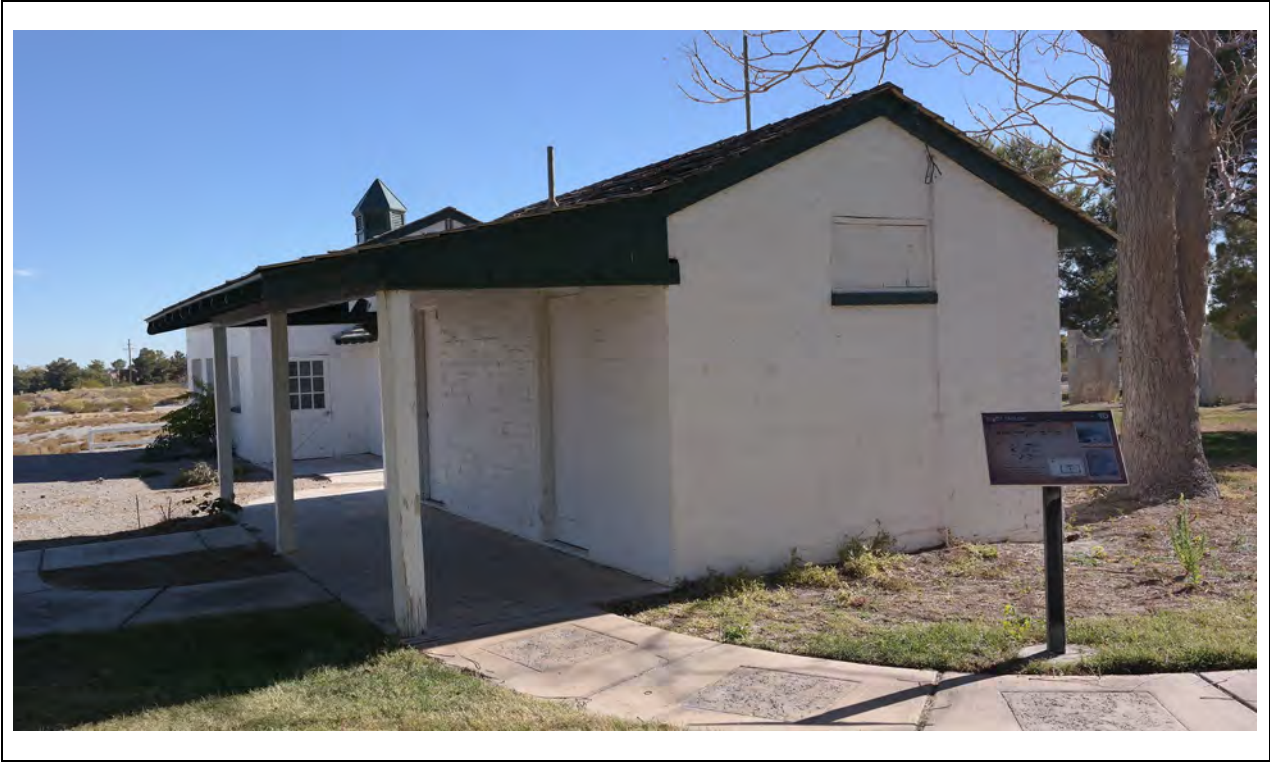
Bath House – Northwest corner Kautz Environmental Consultants, Inc., November 2024
