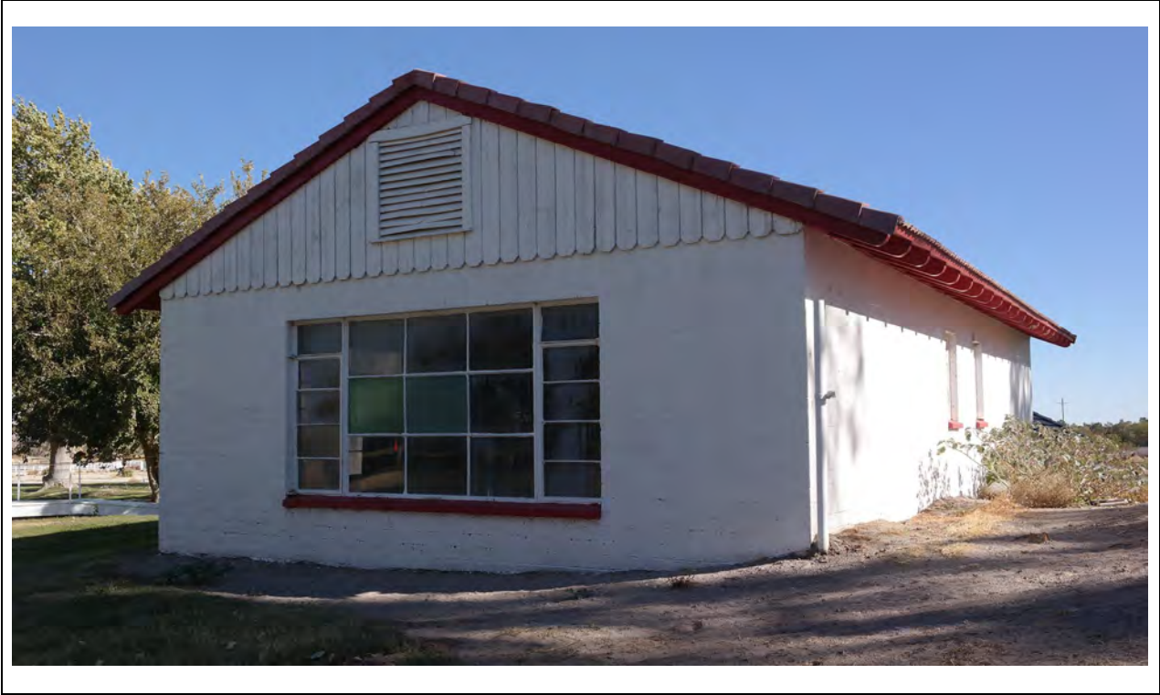
Duplex – Northwest elevation and west corner Kautz Environmental Consultants, Inc., November 2024
