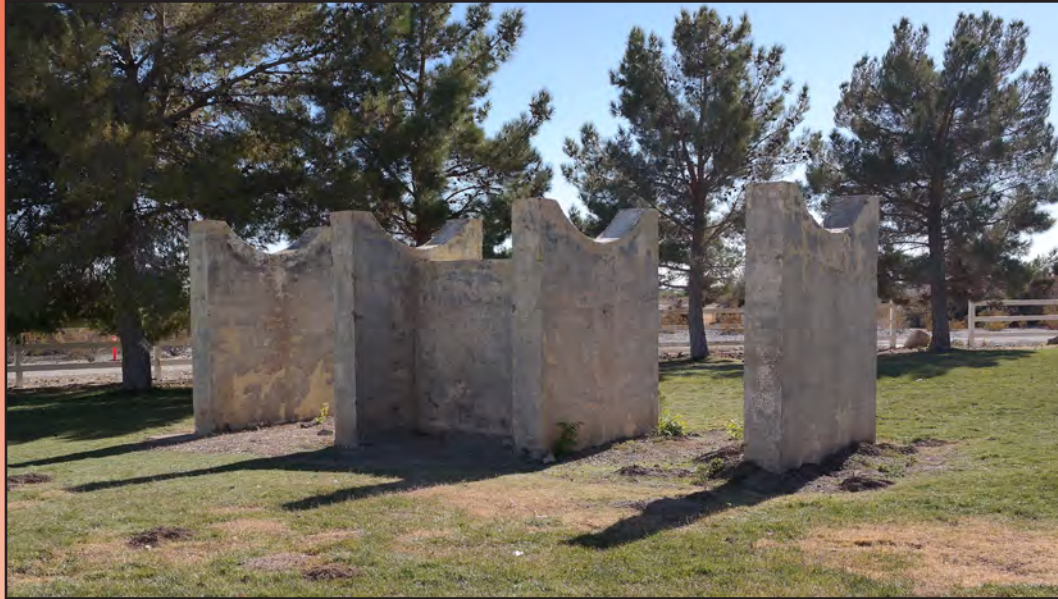
Figure 5.8 Diesel Oil Support (#8)
