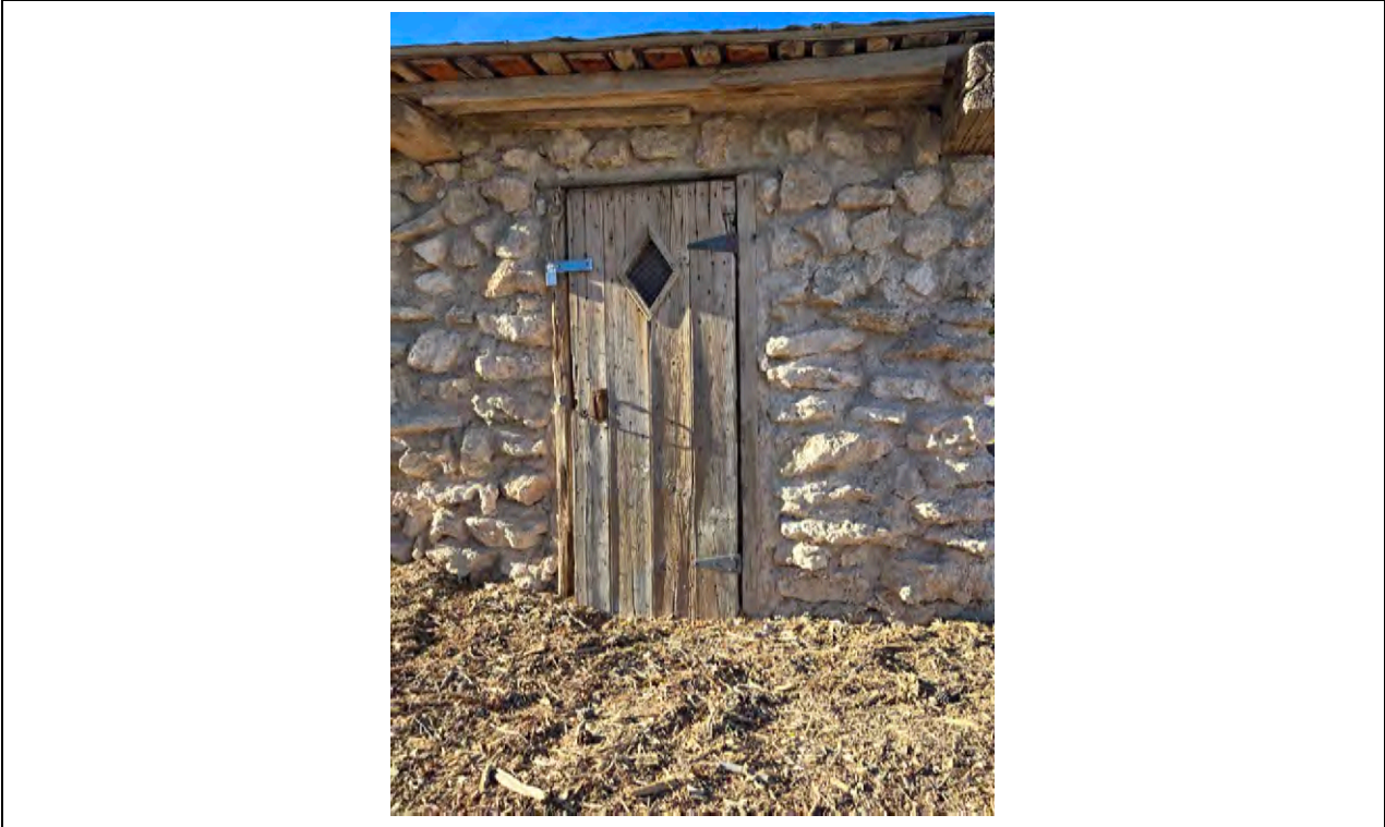
Adobe Hut – Door detail, southeast elevation Kautz Environmental Consultants, Inc., November 2024
