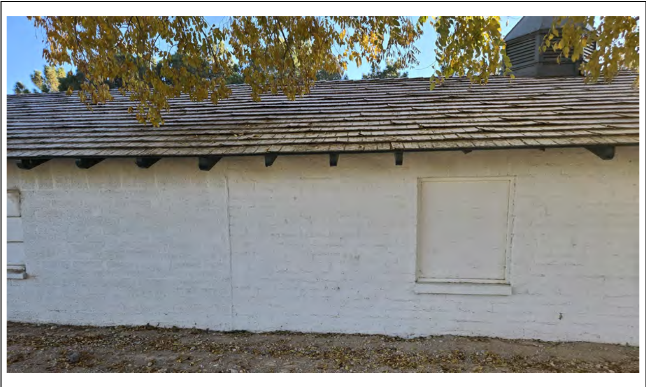
Office/Stables – North elevation, west/center Kautz Environmental Consultants, Inc., November 2024
