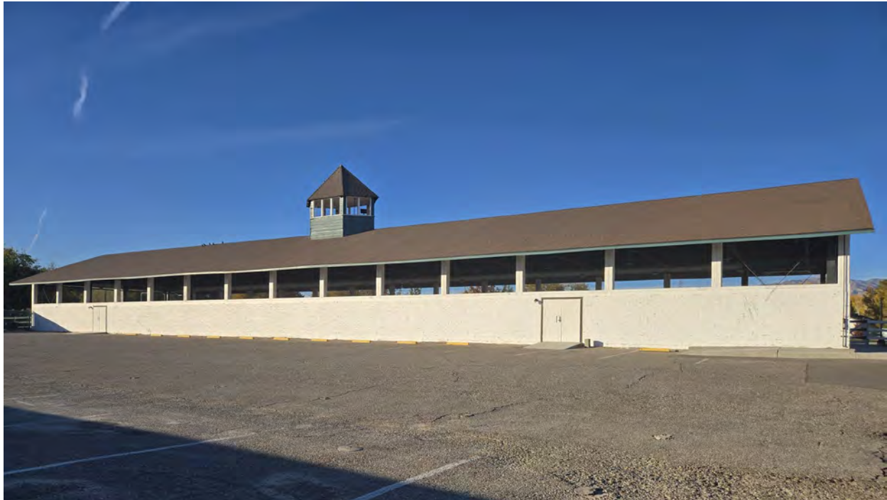
Hay Barn – South elevation
