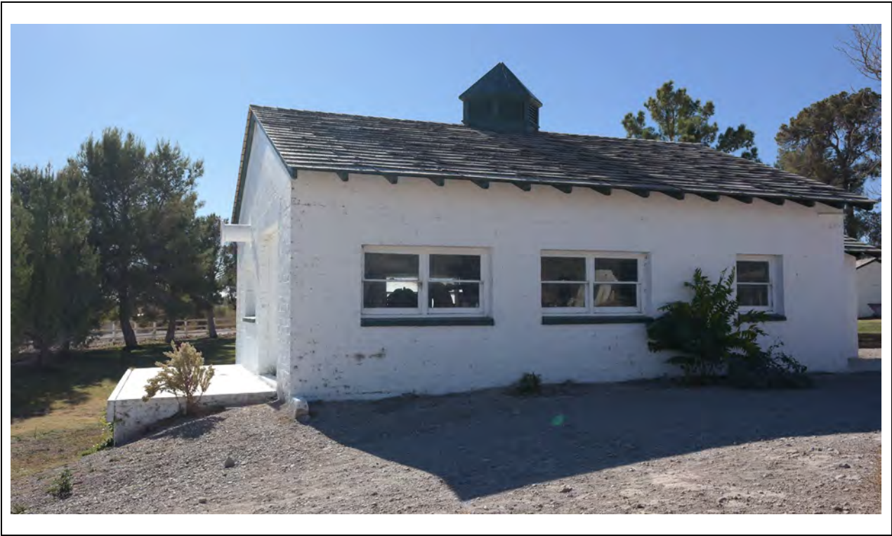
Generator Building – North elevation and northeast corner Kautz Environmental Consultants, Inc., November 2024
