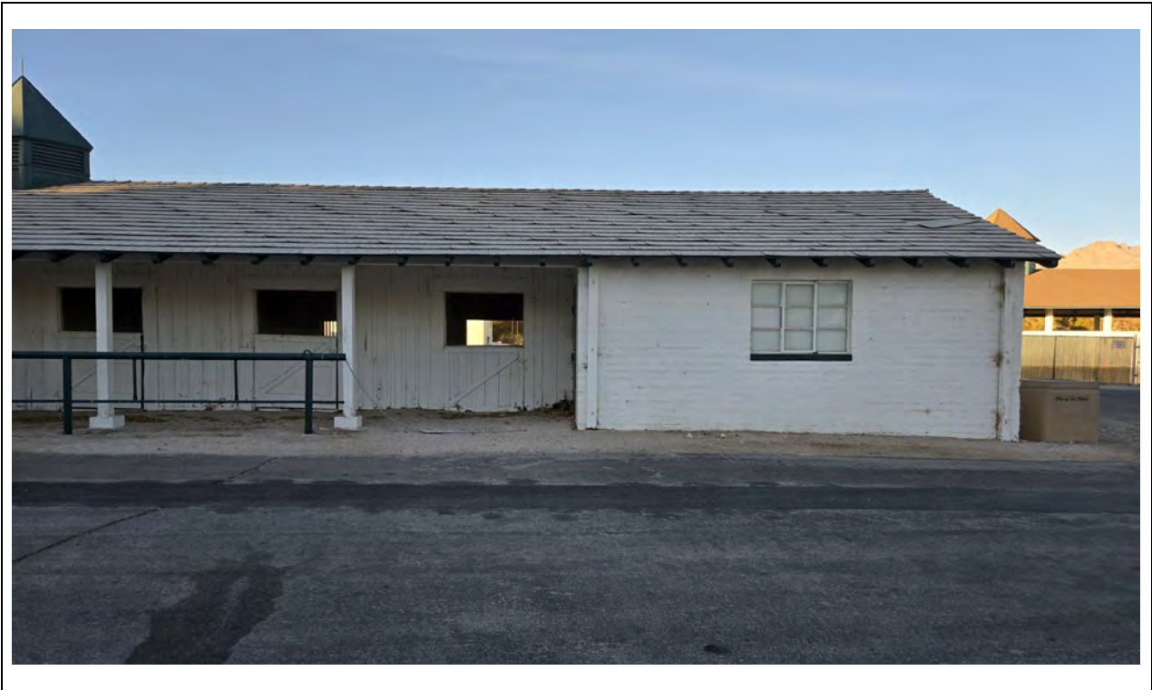
Office/Stables – South elevation, east end Kautz Environmental Consultants, Inc., November 2024
