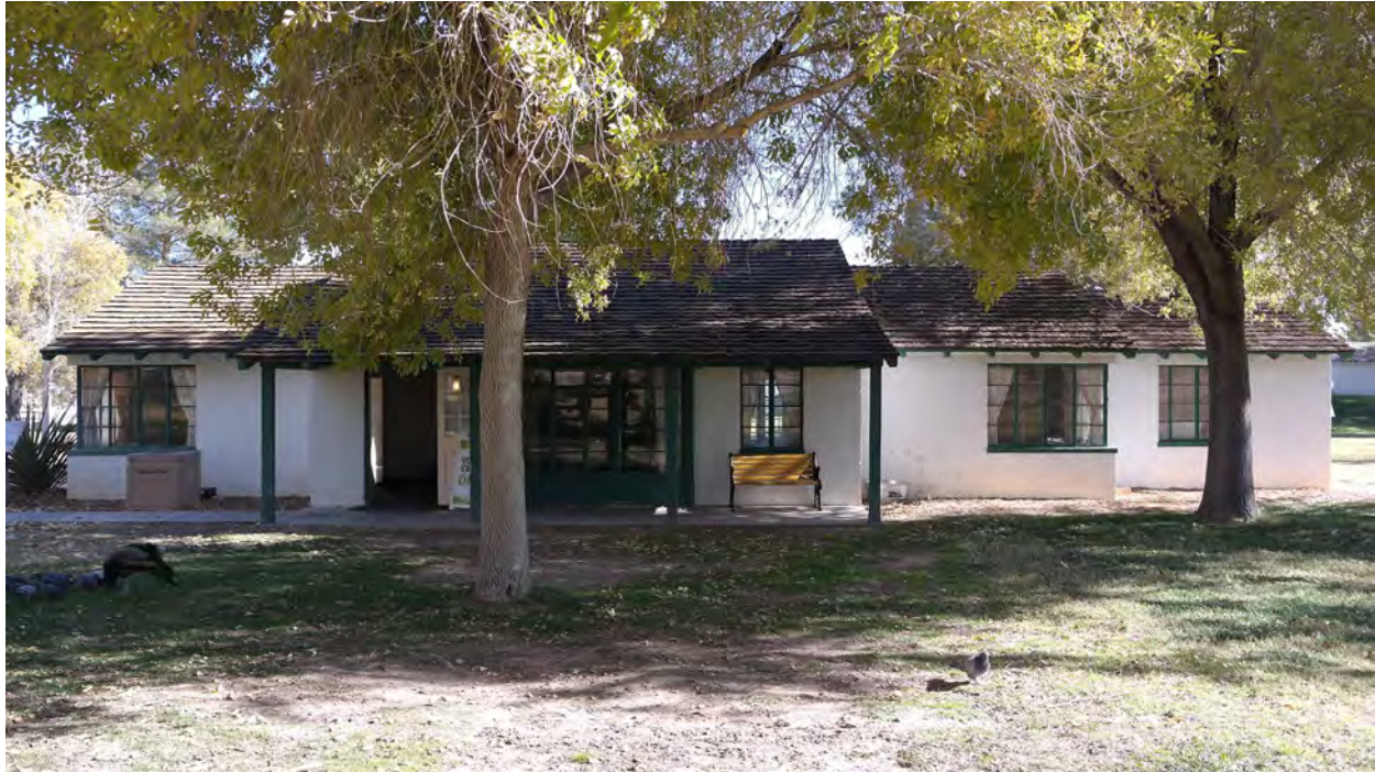
Foreman's House – West elevation
