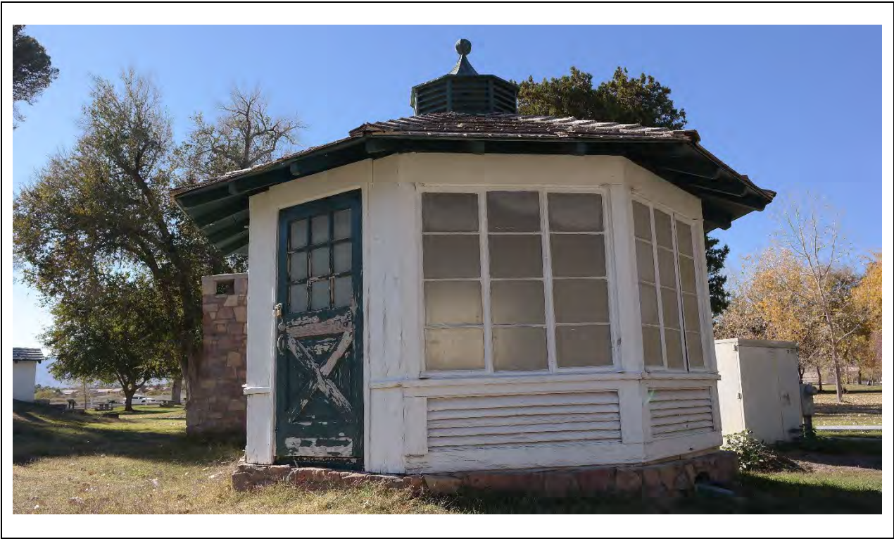
Pump House – East/northeast elevation Kautz Environmental Consultants, Inc., November 2024
