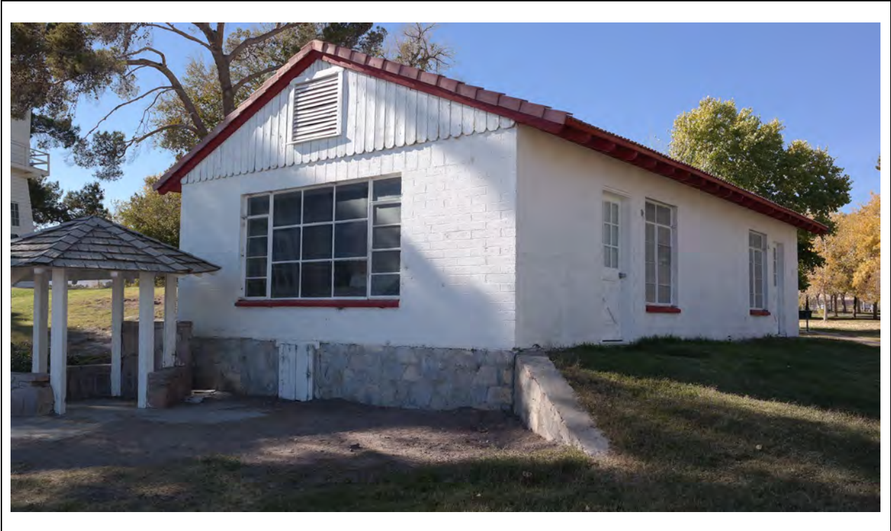
Duplex and Gazebo – East corner Kautz Environmental Consultants, Inc., November 2024
