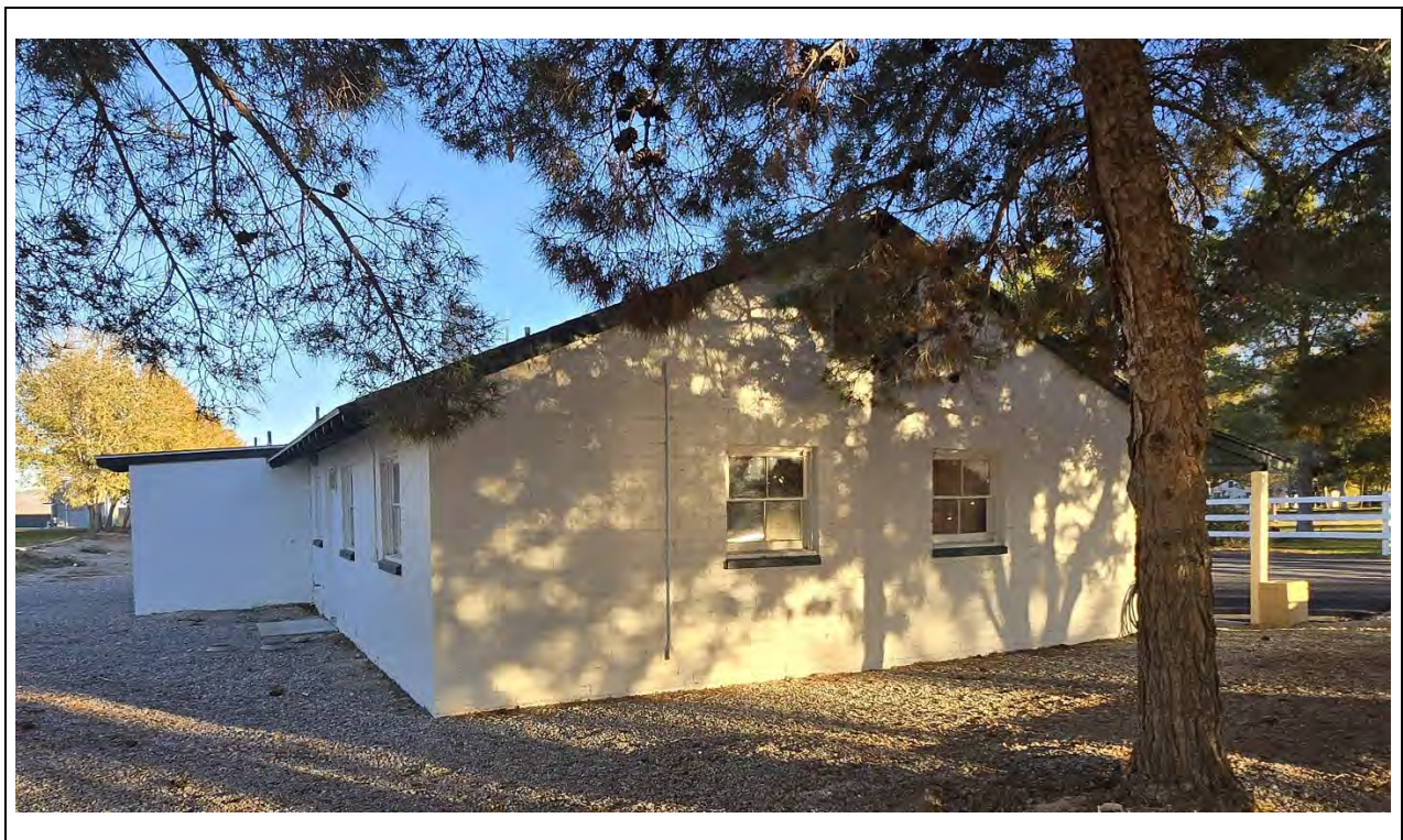
Caretaker's House – West elevation and northwest corner
