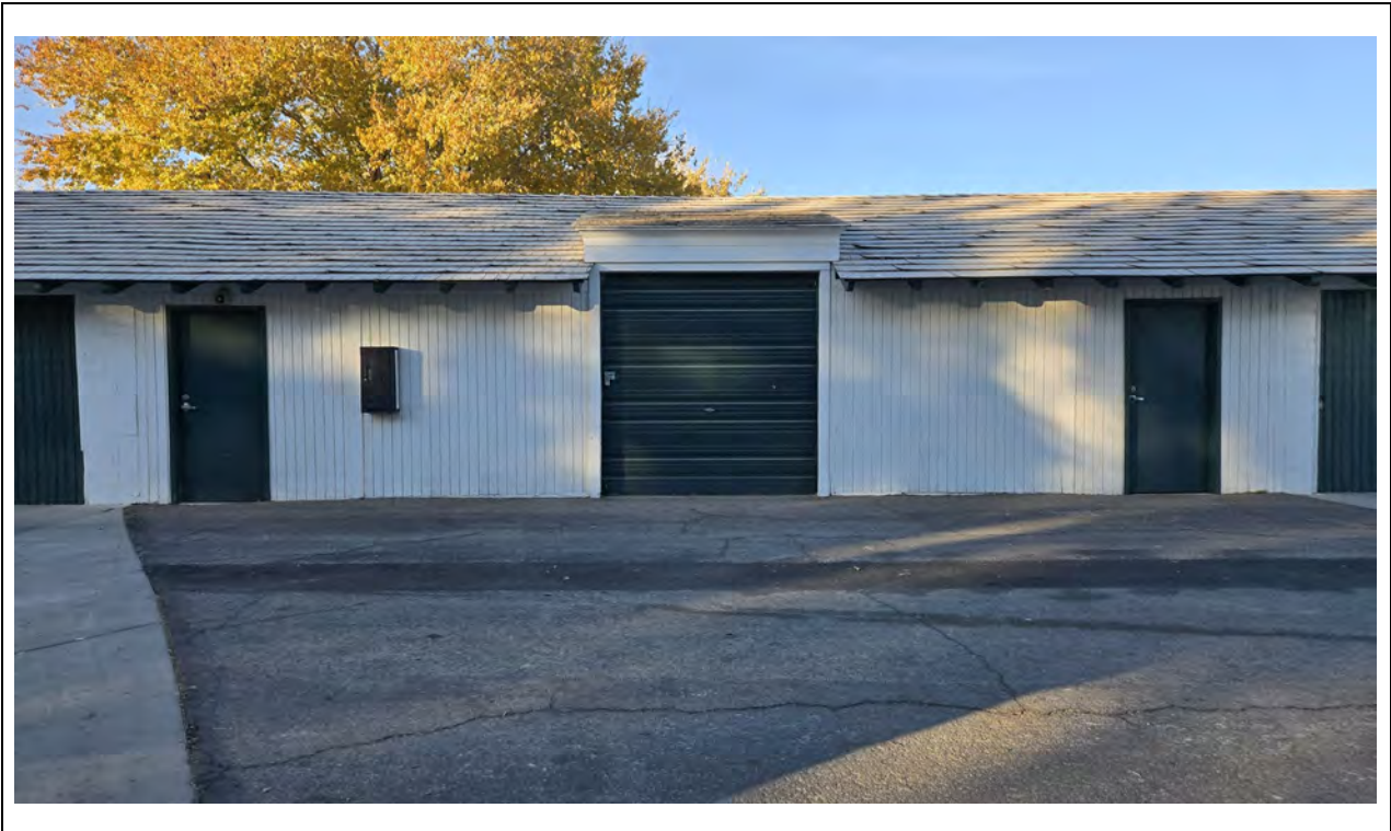
Office/Stables – South elevation, west/center Kautz Environmental Consultants, Inc., November 2024
