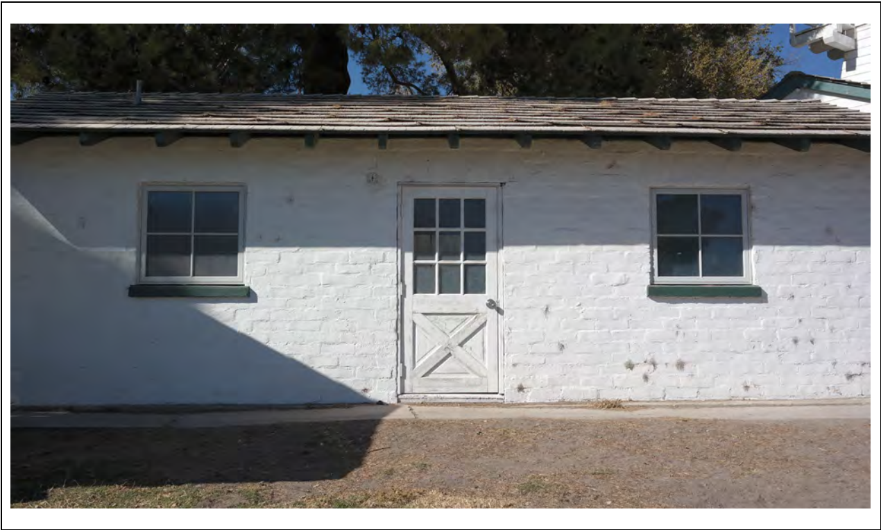
Spring House – Southeast elevation Kautz Environmental Consultants, Inc., November 2024
