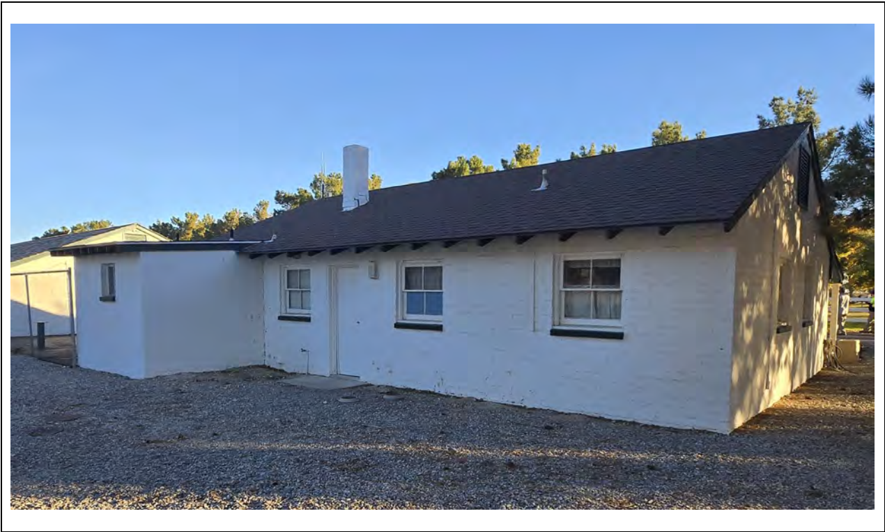
Caretaker's House – North elevation and northwest corner Kautz Environmental Consultants, Inc., November 2024
