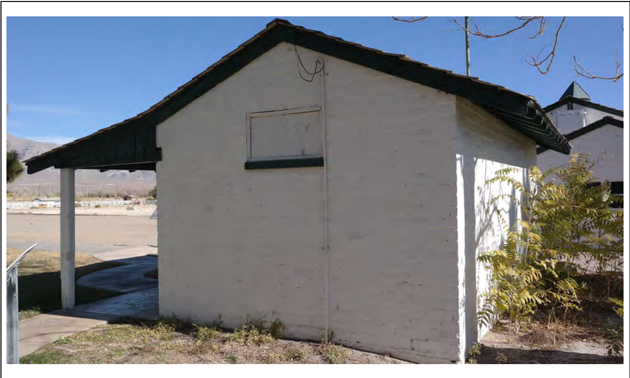
Bath House – West elevation and southwest corner Kautz Environmental Consultants, Inc., November 2024
