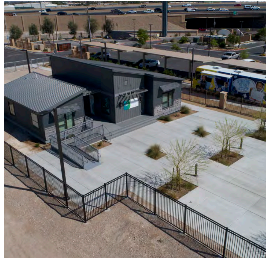
Cox Innovation Lab at the Strong Future Technology Training Center
