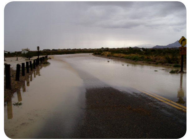
Park access road flooding. Flooding is more common with the increased development surrounding Floyd Lamb Park. Land that once served as surface area for storm water filtration is being developed and storm water flow is increasingly more channelized resulting in greater amounts of water travelling at high speeds. These are examples of flooding at the Park. (Photos courtesy of Park Supervisor Steve Santee).
