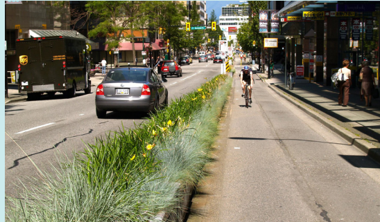
1. Planter box or concrete barriers
