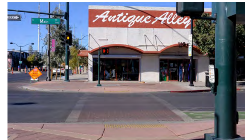
Pedestrian crosswalk with curb cut, tactile indicators, and pedestrian signal on Main St., Las Vegas. (Happy Cities)
