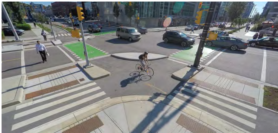
Protected intersection for bikes and pedestrians in Vancouver, allowing bikes to complete a two-stage turn within a curb-protected area. (Dylan Passmore / Flickr)
