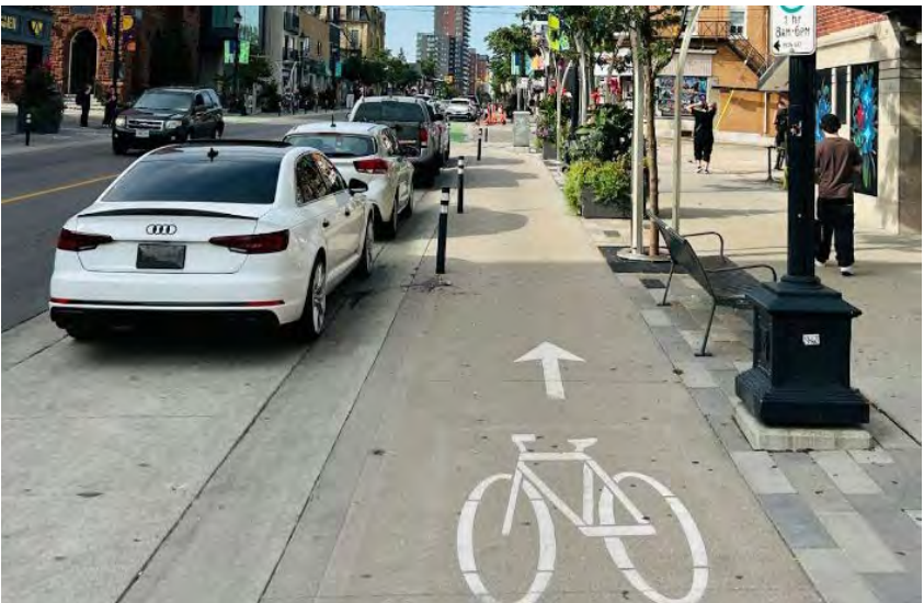
■ Raised cycle track in Waterloo, with bollards and parking offering physical protection from the road, and an amenity zone in between the sidewalk and bikeway. (Jason Thorne / Flickr)
