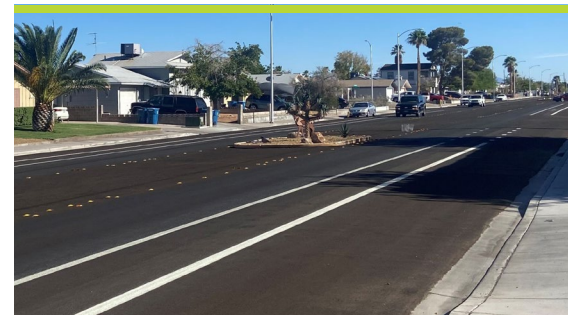
Curbed Road Diet (Level 4)
