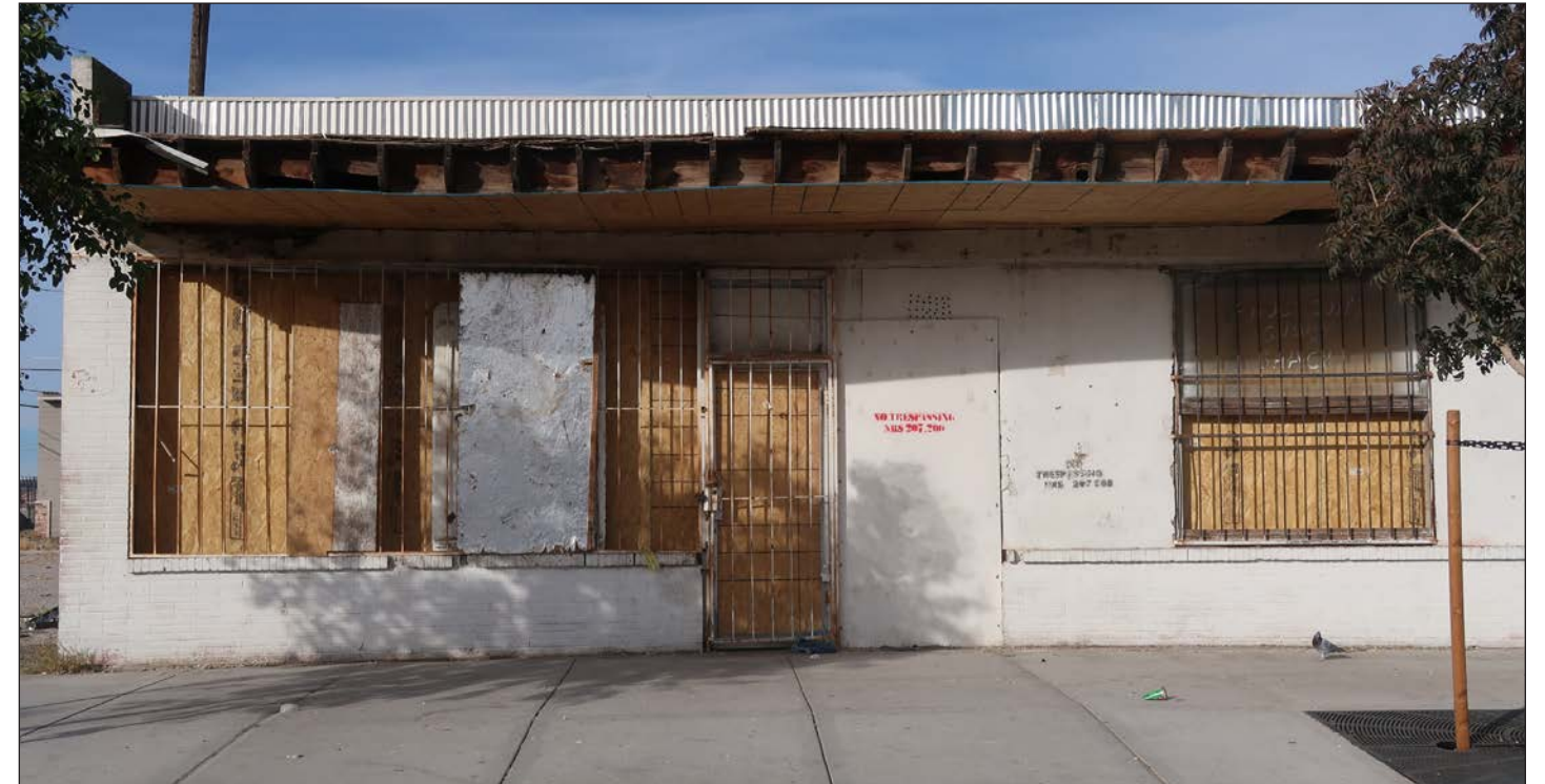
Recommend incorporating beveled storefronts and bulkheads into new infill construction
