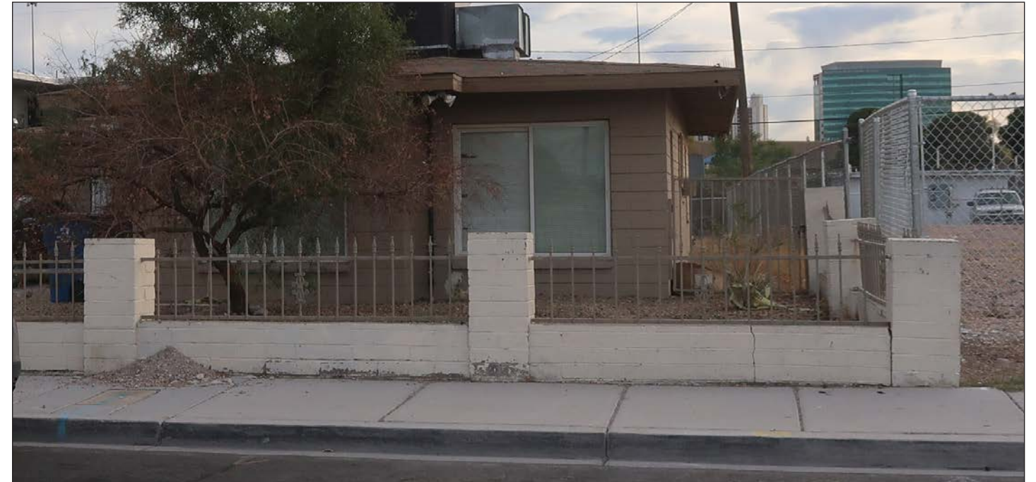
Wrought iron fence with CMU stem wall
