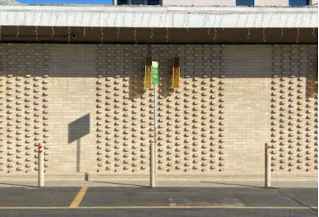
Running bond with decorative projecting block/shadow block
