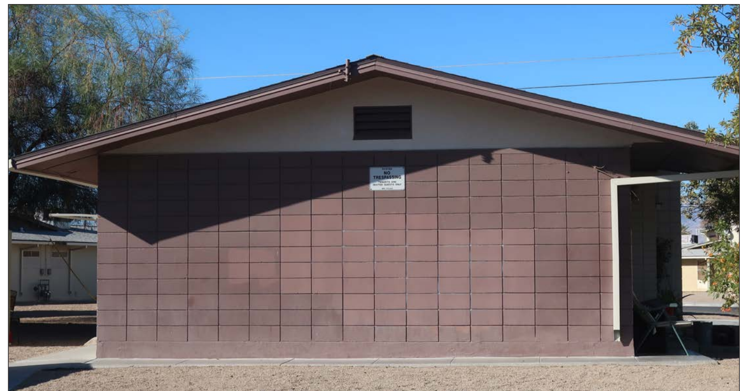
Recommend retaining CMU on existing buildings in the District
