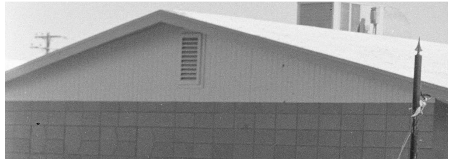
Wood in the upper eaves
