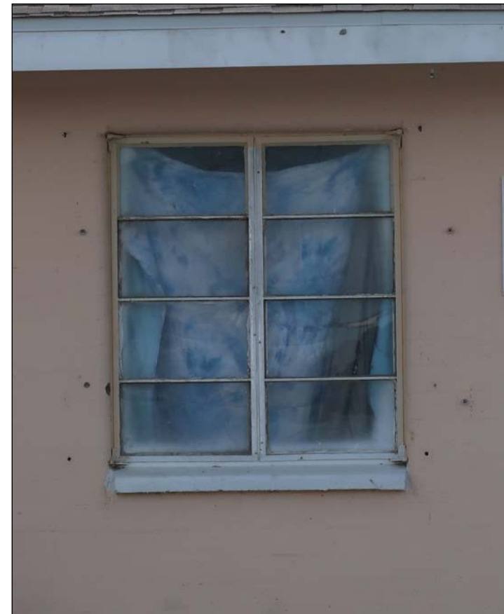
Example of steel sash window
