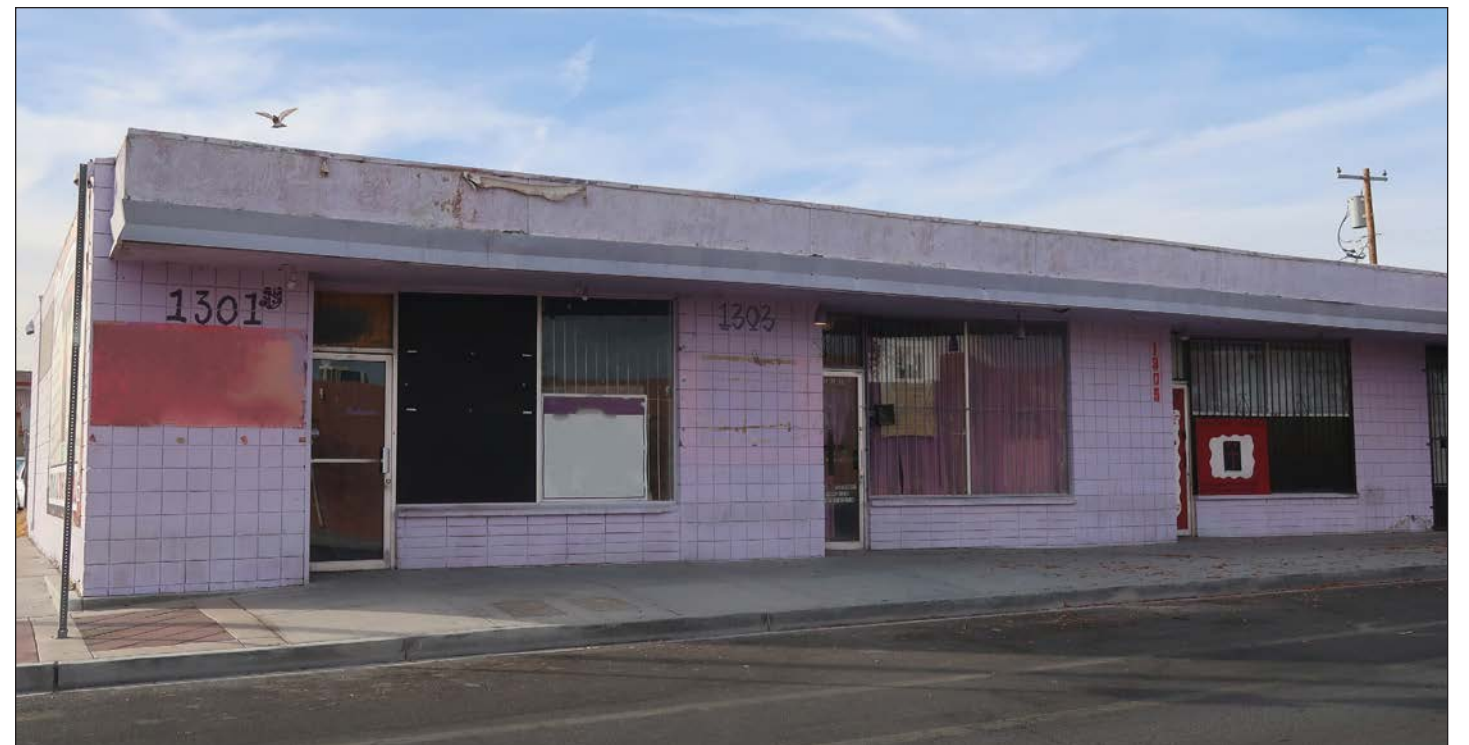
Recommend incorporating angled storefronts into new infill construction
