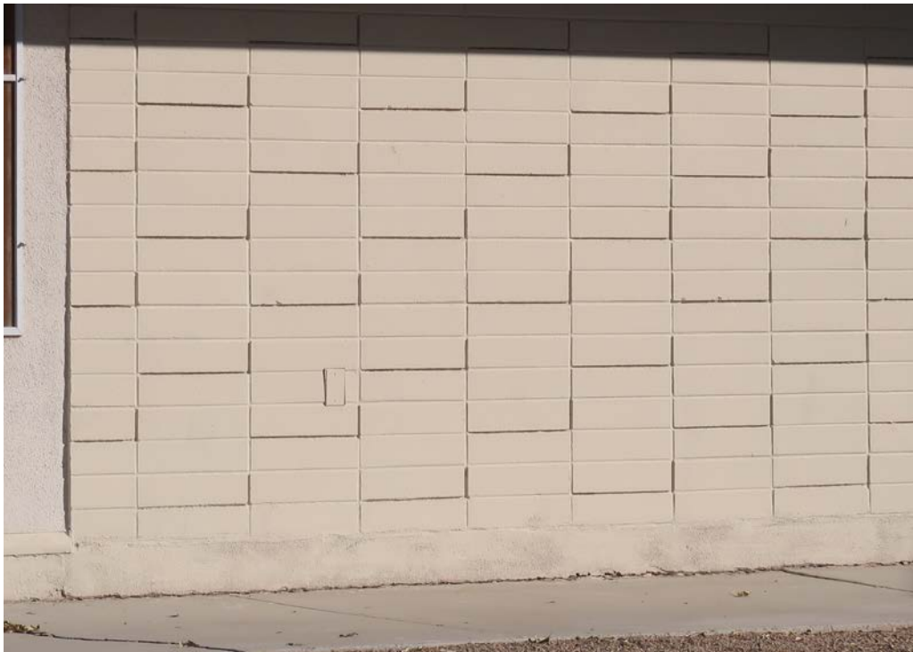
Stack bond with recessed mortar joint detailing
