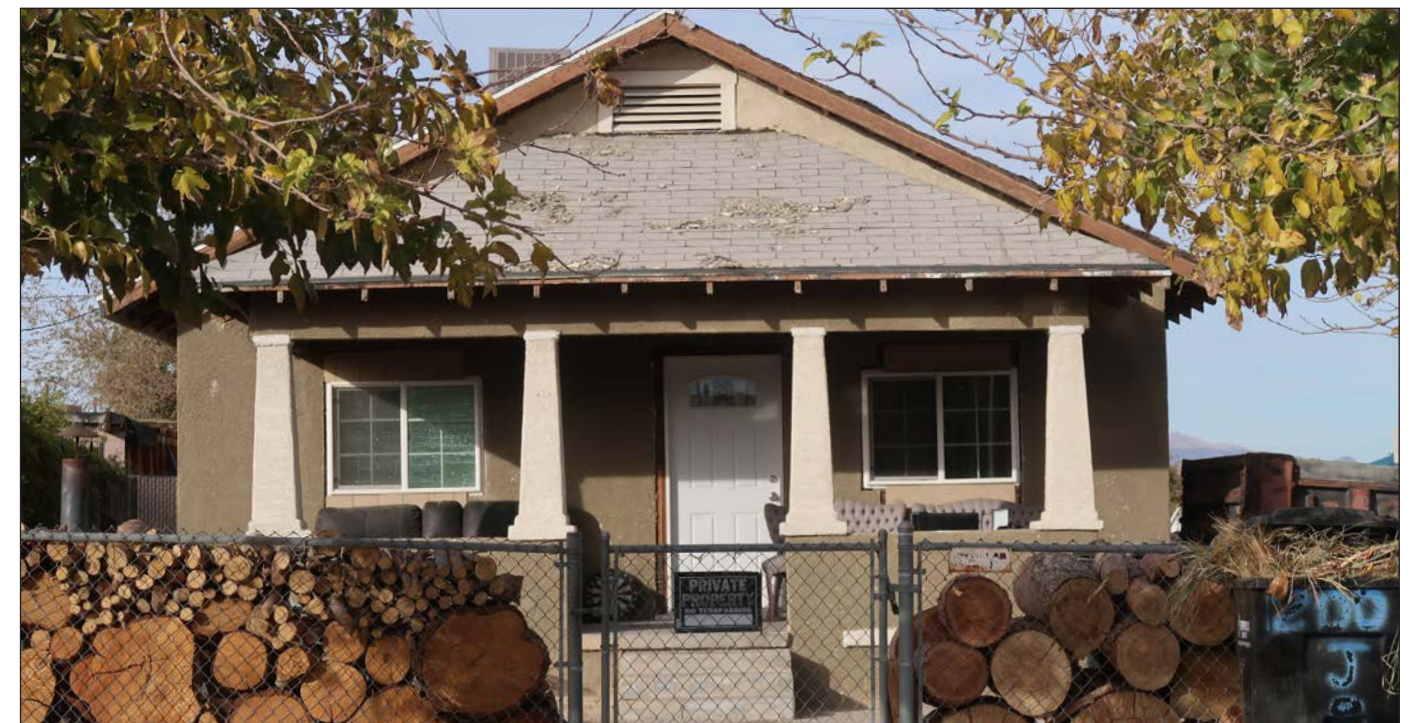
Example of historic porch in the District
