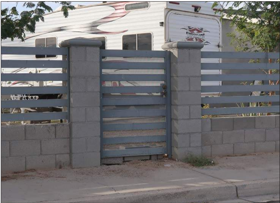
CMU wall with vertical panel fencing
