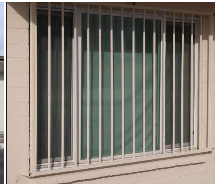
Example window with security grille
