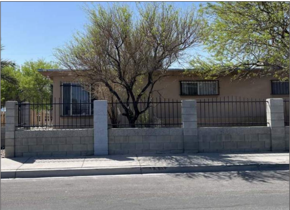
Wrought iron fence with CMU stem wall
