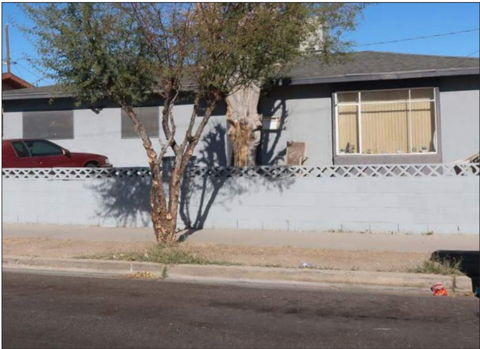
CMU wall with decorative block
