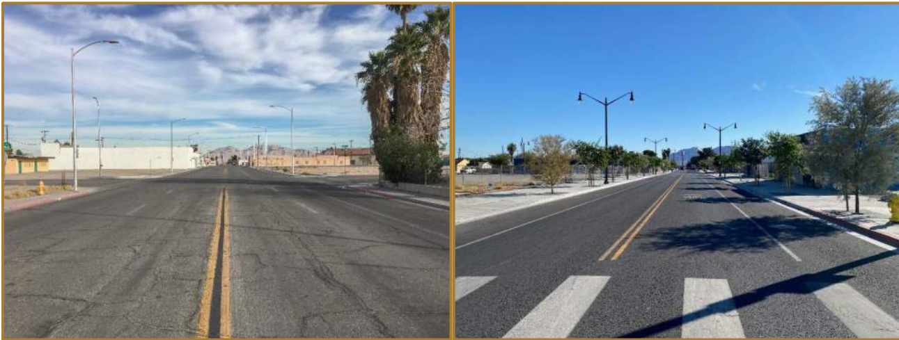
Figure 12: Before and After 2022 Roadway Improvement Photos of Jackson Ave. (Source: Wood Rodgers)
