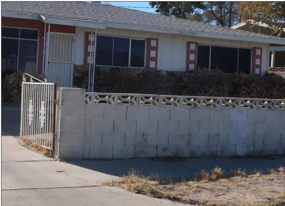
CMU wall with decorative block
