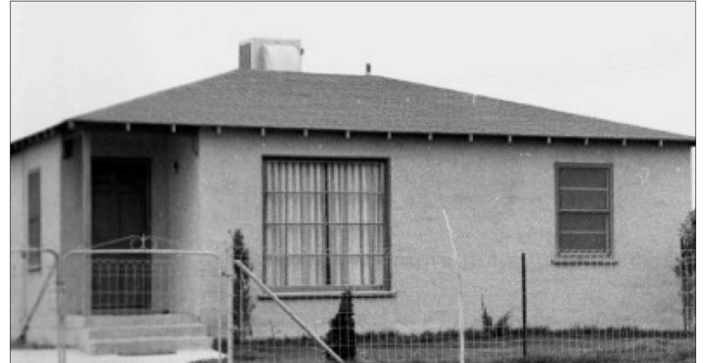
View of historic building with MEP at rear slope of roof
